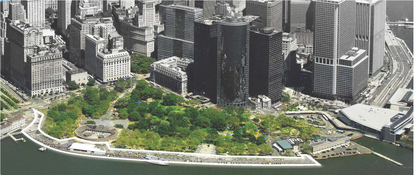
Image: Aerial image of The Battery and project limits (Stantec).
