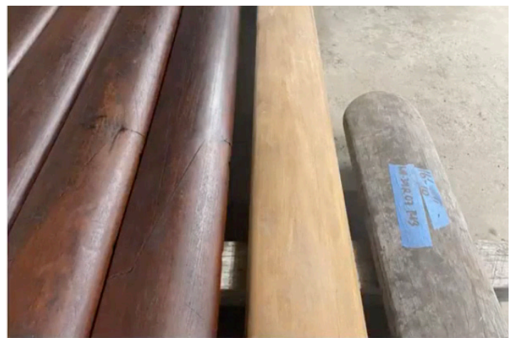
Image from right to left: Tropical hardwood searail undergoes several phases of refurbishment (salvage, cleaning/sanding, and oiling) until it is ready for re-installation.
