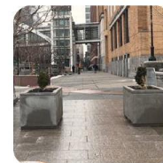
Planting Concrete Bollards
