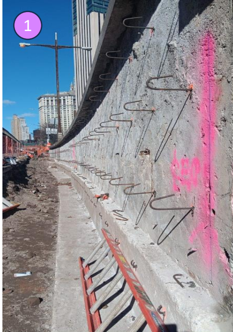
Rebar j-hooks for floodwall tie in on FDR off-ramp – March 2024
