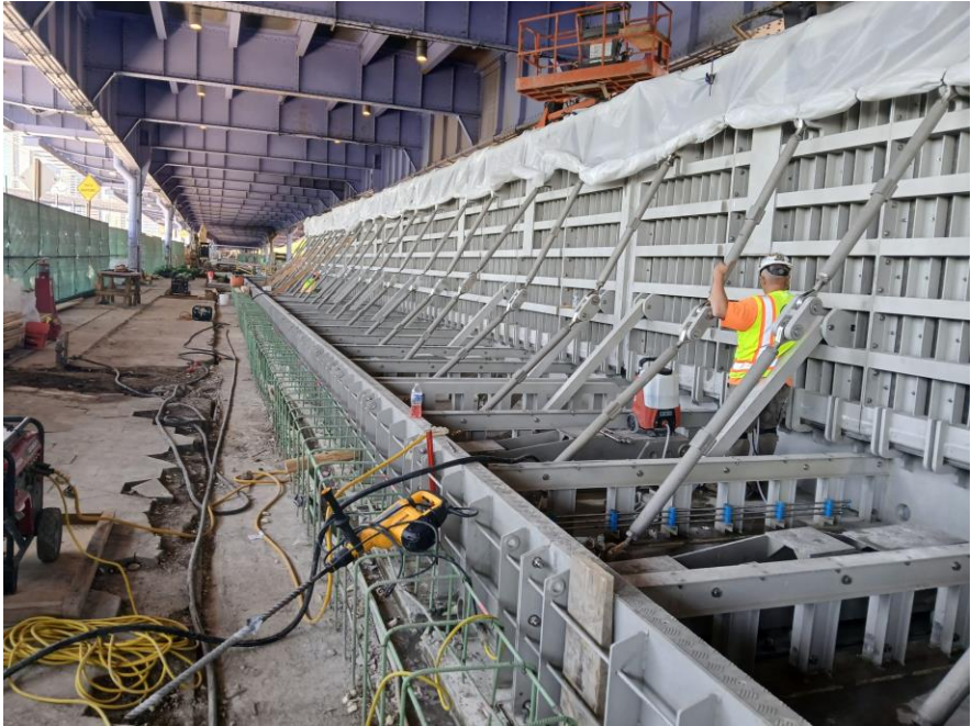
Deployed flip up gate during installation - June 2024
