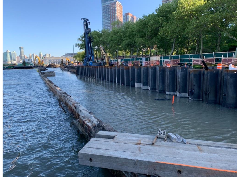
May 2024 – Sheet Pile Installation
