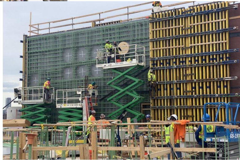
Wagner Park: Partial Installation of Pavilion Rebar & Concrete Formwork
