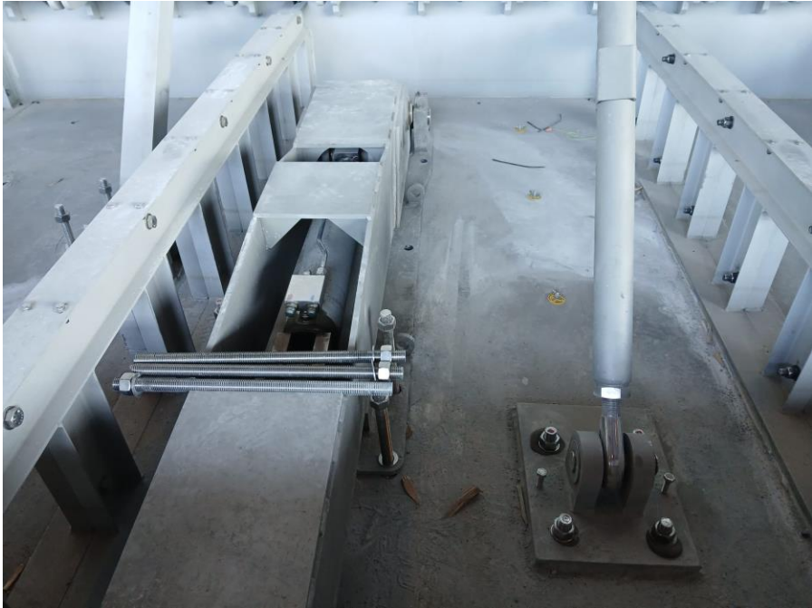
Flip up gate hydraulics – June 2024
