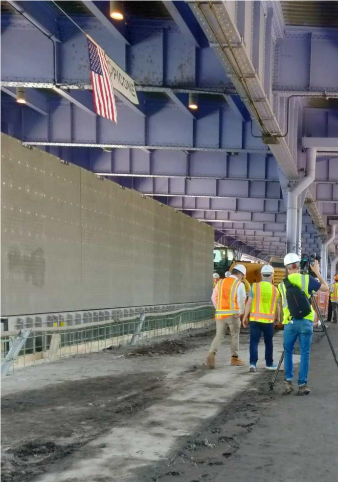
Deployed flip up gate, dry side during installation – June 2024
