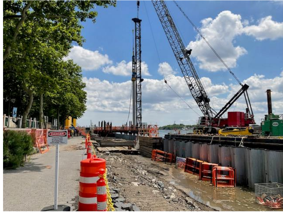
June 2024 – Pile Driving
