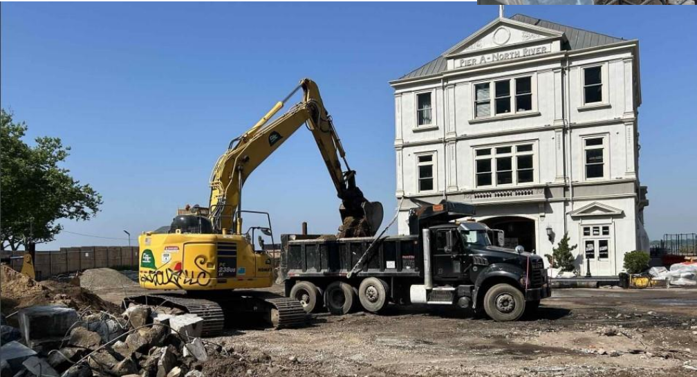
Pier A Plaza & The Battery: Site Demolition
