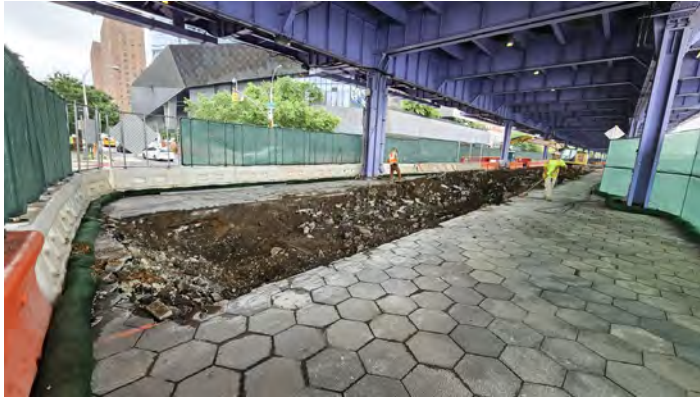
Excavation for floodgate foundation
