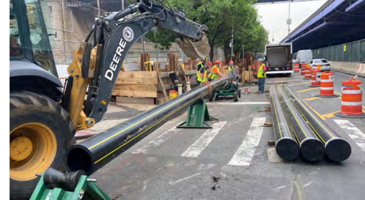
Gas main installation
