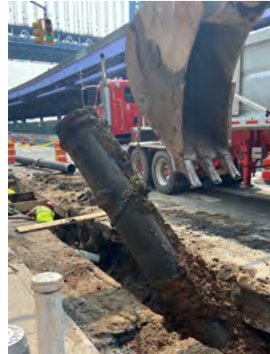
Water main removal
