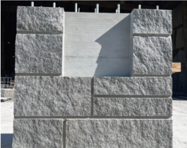
Image: Wharf Lower Fascia
