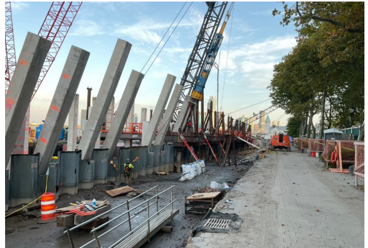
Image: Pile Driving
