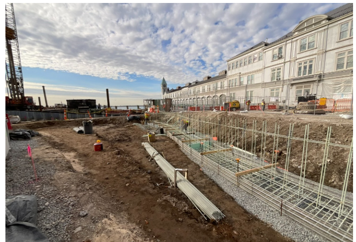
Image: Concrete Retaining Wall Installation to be Clad with Salvaged Granite
