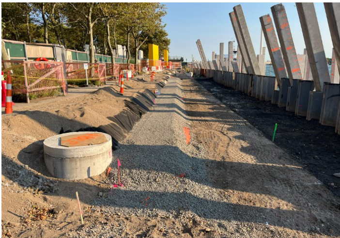
Image: Storm Drainage Backfill and Compaction
