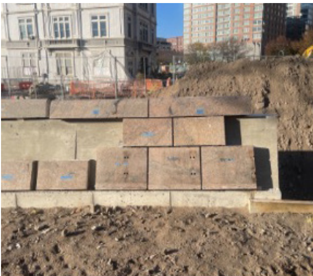
Image: Granite Back Bench Wall using Salvaged Stony Creek Granite
