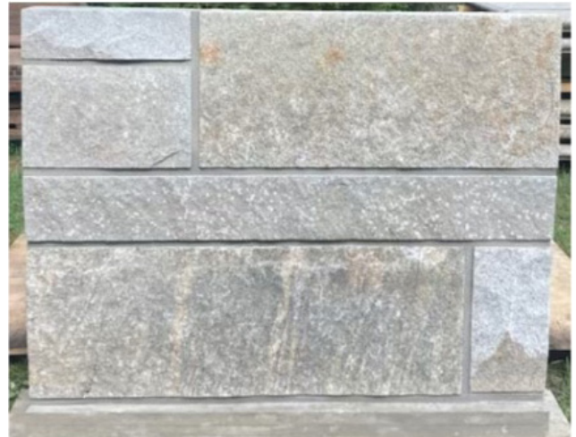
Image: Wharf Upper Fascia using Salvaged Stone
