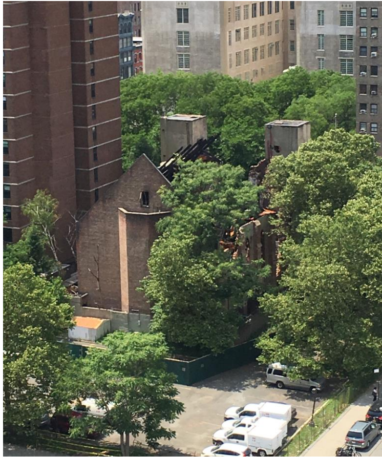
Aerial View from North East
