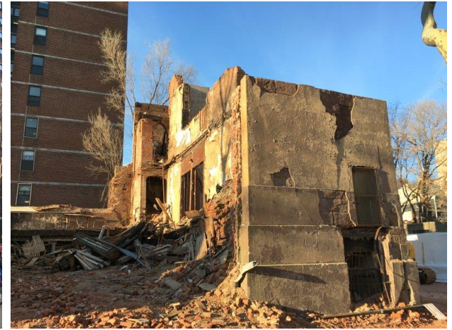
North West Corner
