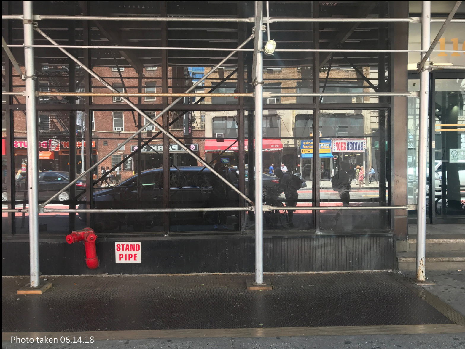
EXISTING STOREFRONT, ENTRY, & ADJACENT VAULT
