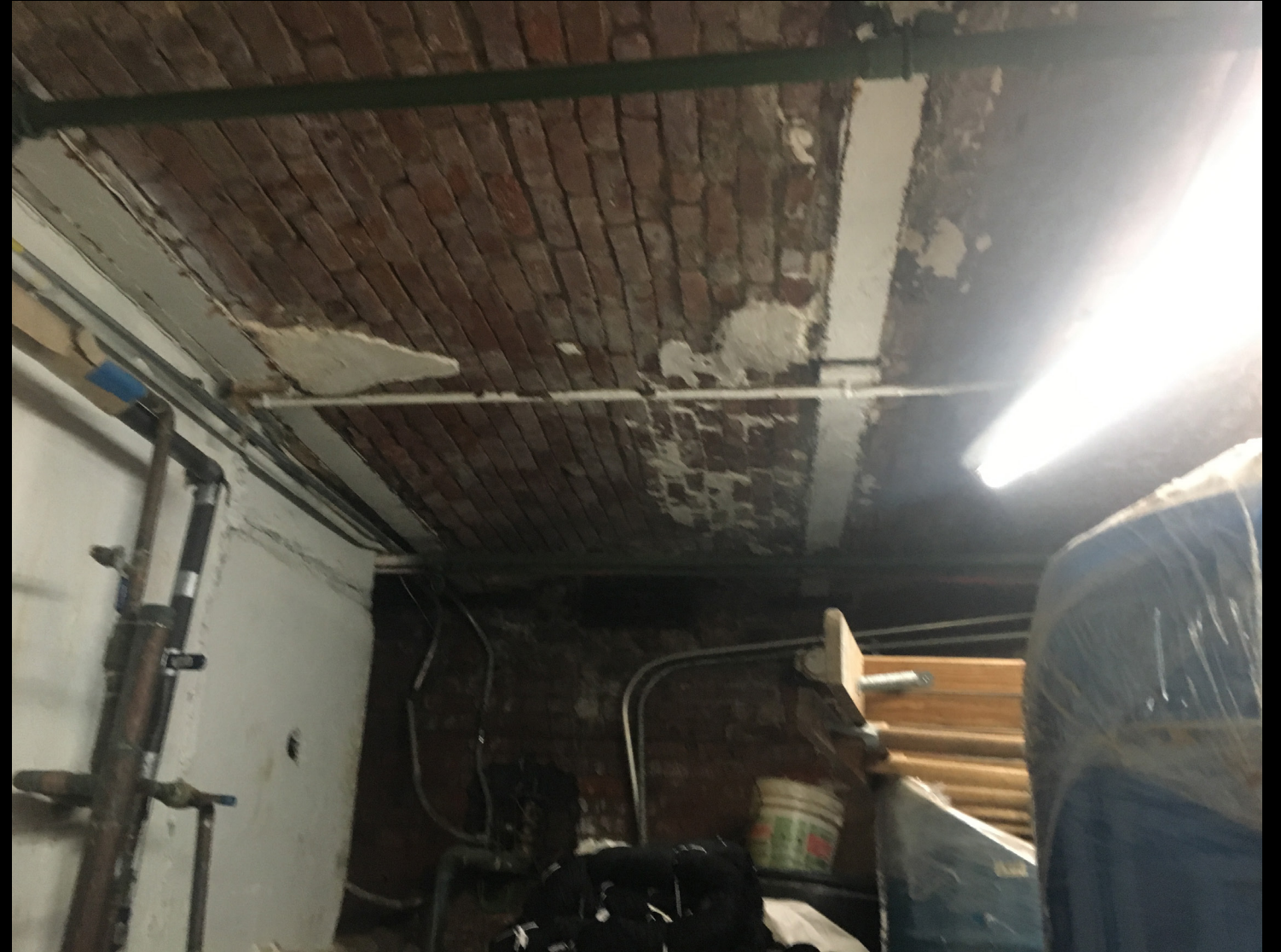
EXISTING UNDERSIDE OF SIDEWALK VAULT - EAST SIDE
