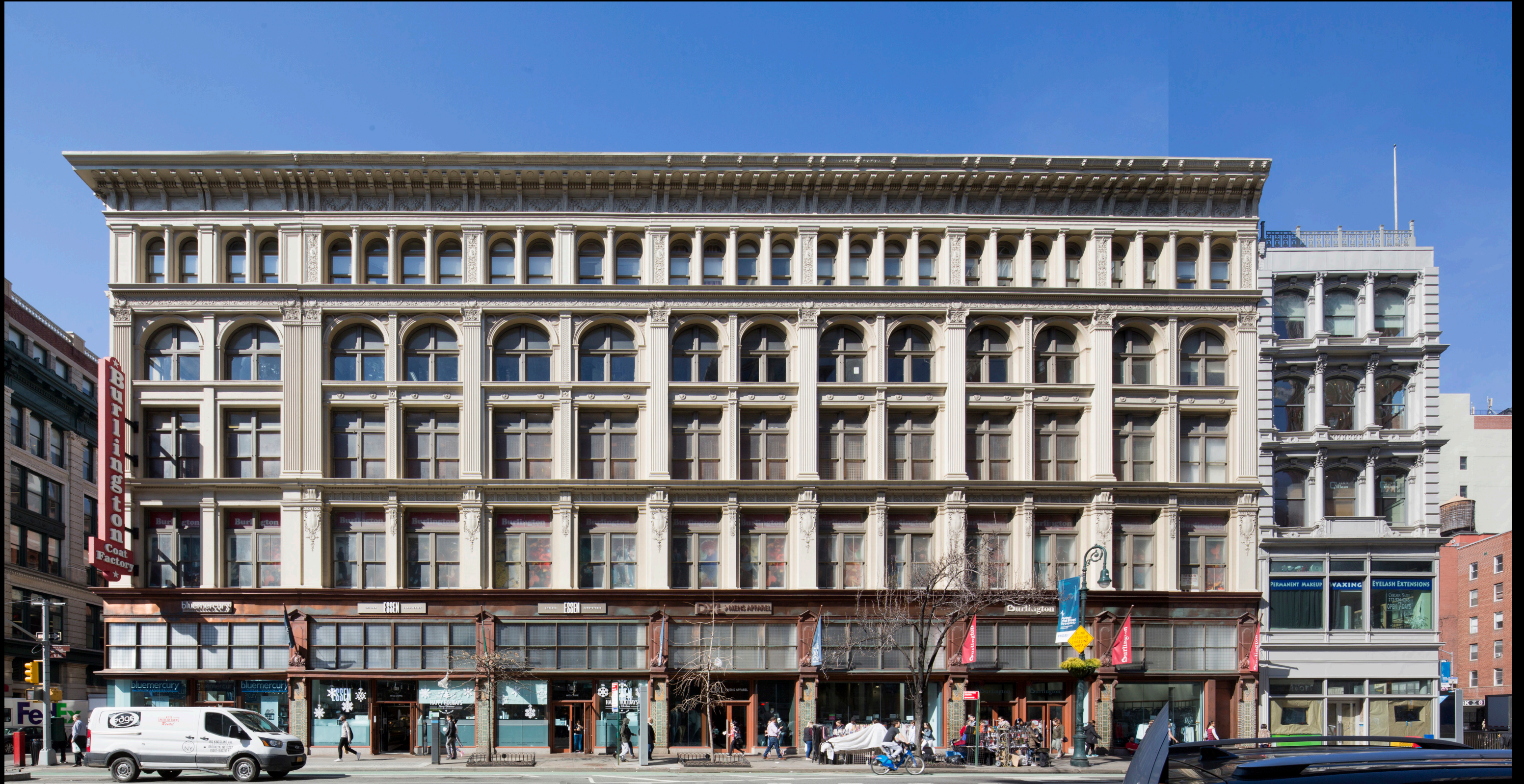
OVERALL 6TH AVENUE FACADE
