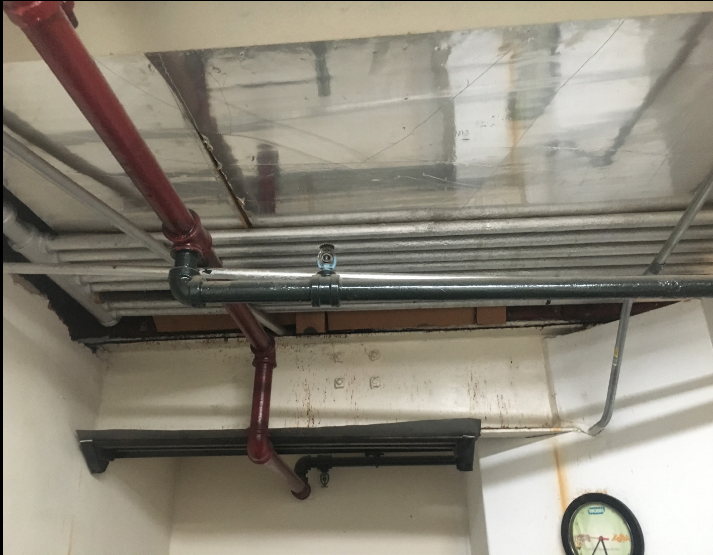
EXISTING UNDERSIDE OF SIDEWALK VAULT - WEST SIDE
