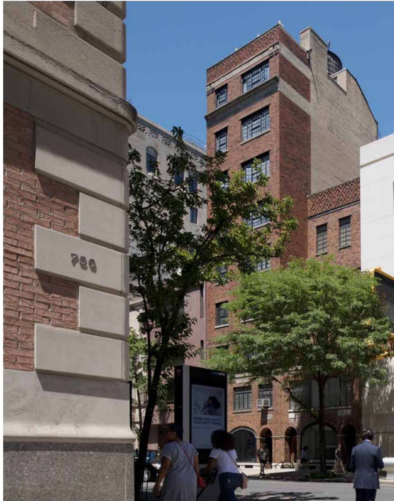
EXISTING CONDITION LOOKING NORTH-WEST
