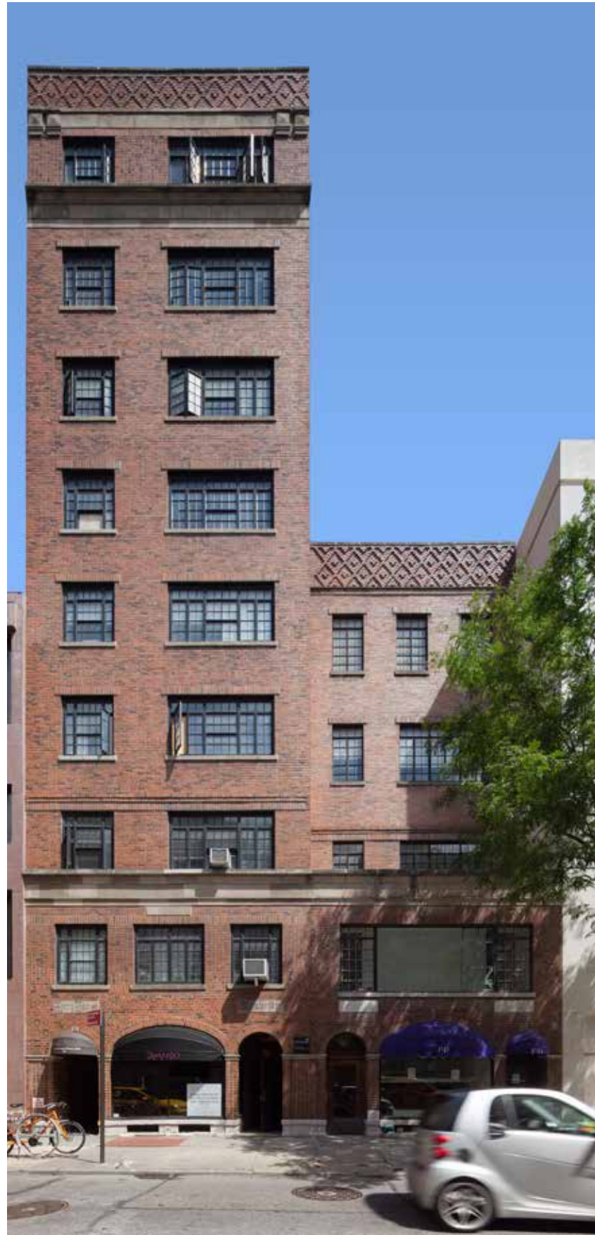
EXISTING CONDITION LOOKING NORTH
