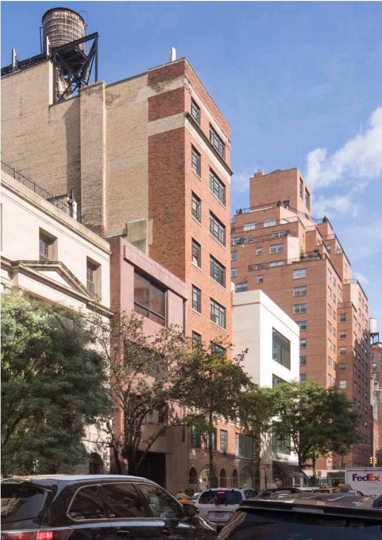
EXISTING CONDITION LOOKING NORTH-EAST
