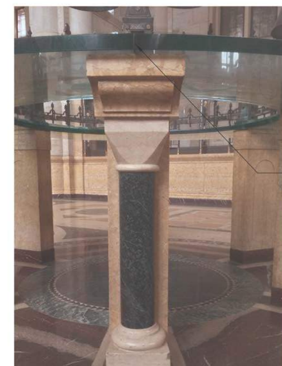
05 CIRCULAR TABLE - 1.5" PLATE GLASS TABLE TOP ALIGNMENT NFS
