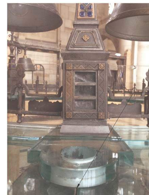
01 CIRCULAR TABLE - 1" GLASS MENDING PLATE CONNECTION NFS
