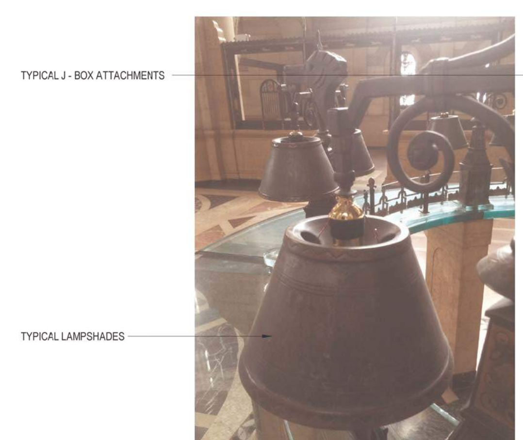
05 CIRCULAR TABLE - TYPICAL CONDITIONS OF TABLE COMPONENTS TO BE REPAIRED N7S
