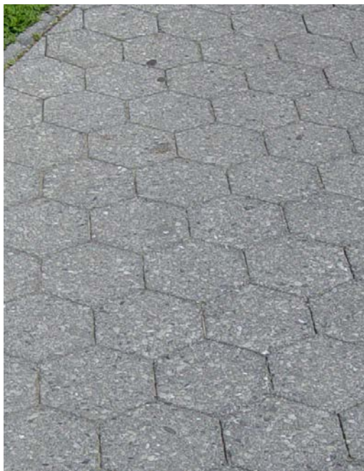
Asphalt Hex Block Paving
