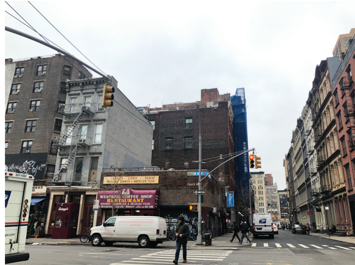
5) View looking south-east at cross street of Church and Lispenard
