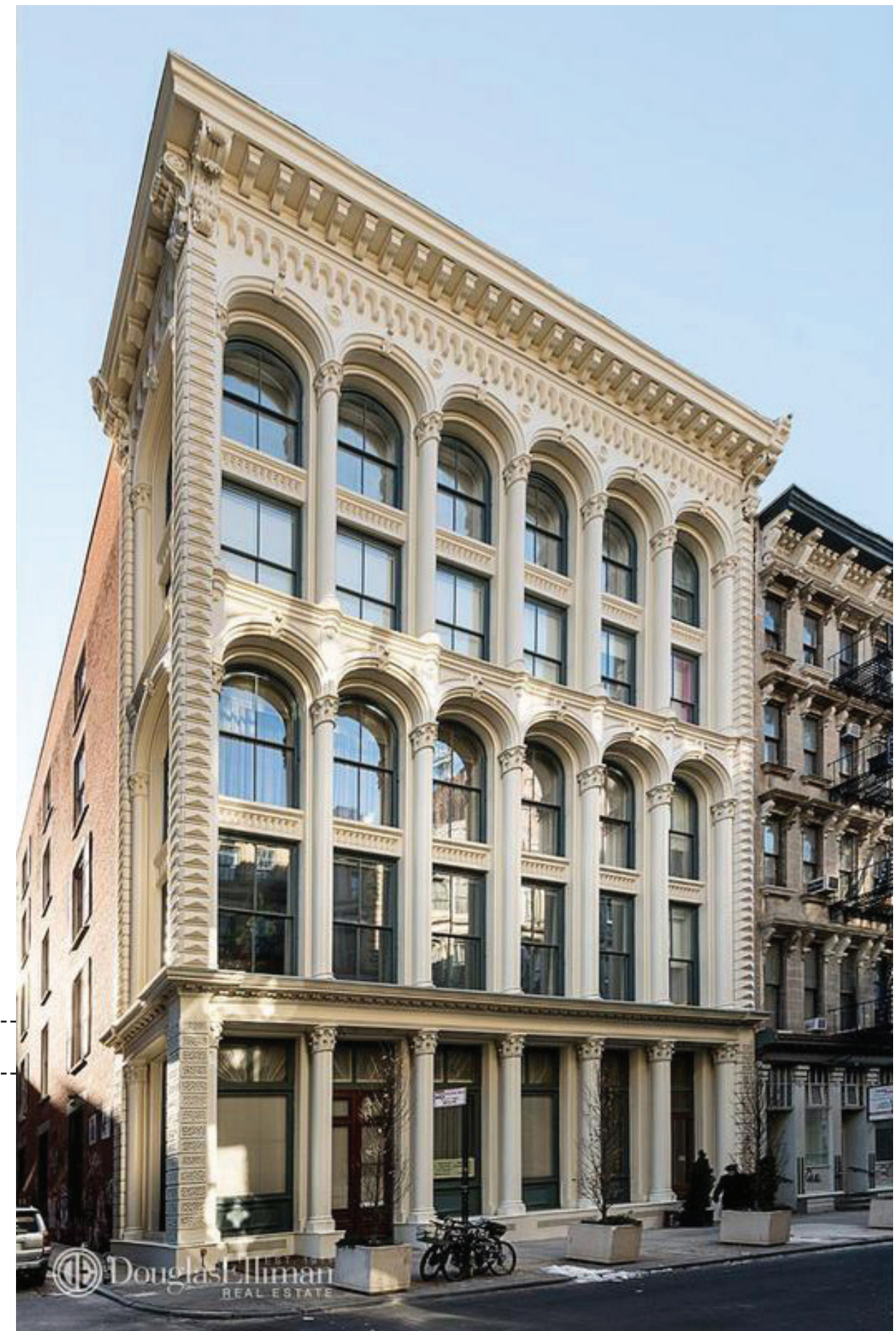
Italianate cast iron warehouse, John Kellum, 55 White Street (1861)
