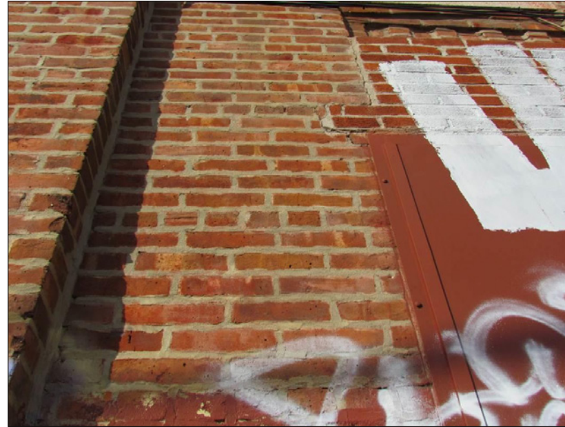
Image 1: Original brick along Belvidere St. façade with light firing pattern on surface
