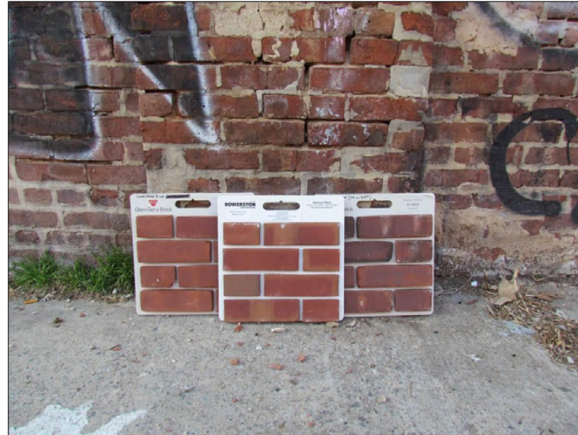
Image 2: Brick boards against original brick on Belvidere St. façade. Irish Gold brick board at center. Glen-Gery 52-DD at left.
