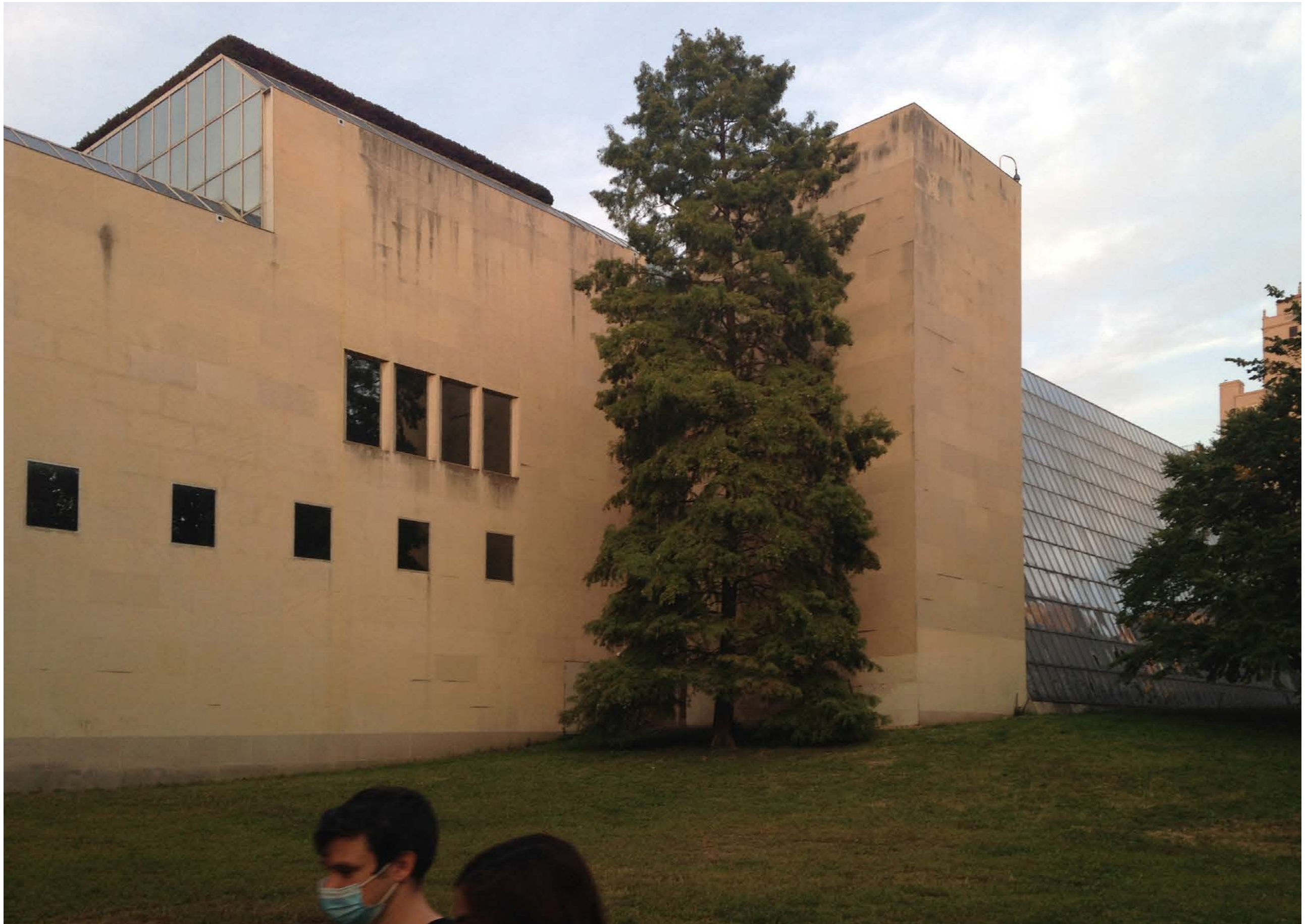
EXISTING CONDITION PHOTO: VIEW OF MET SOUTHWEST WING AND ROCKEFELLER WING
