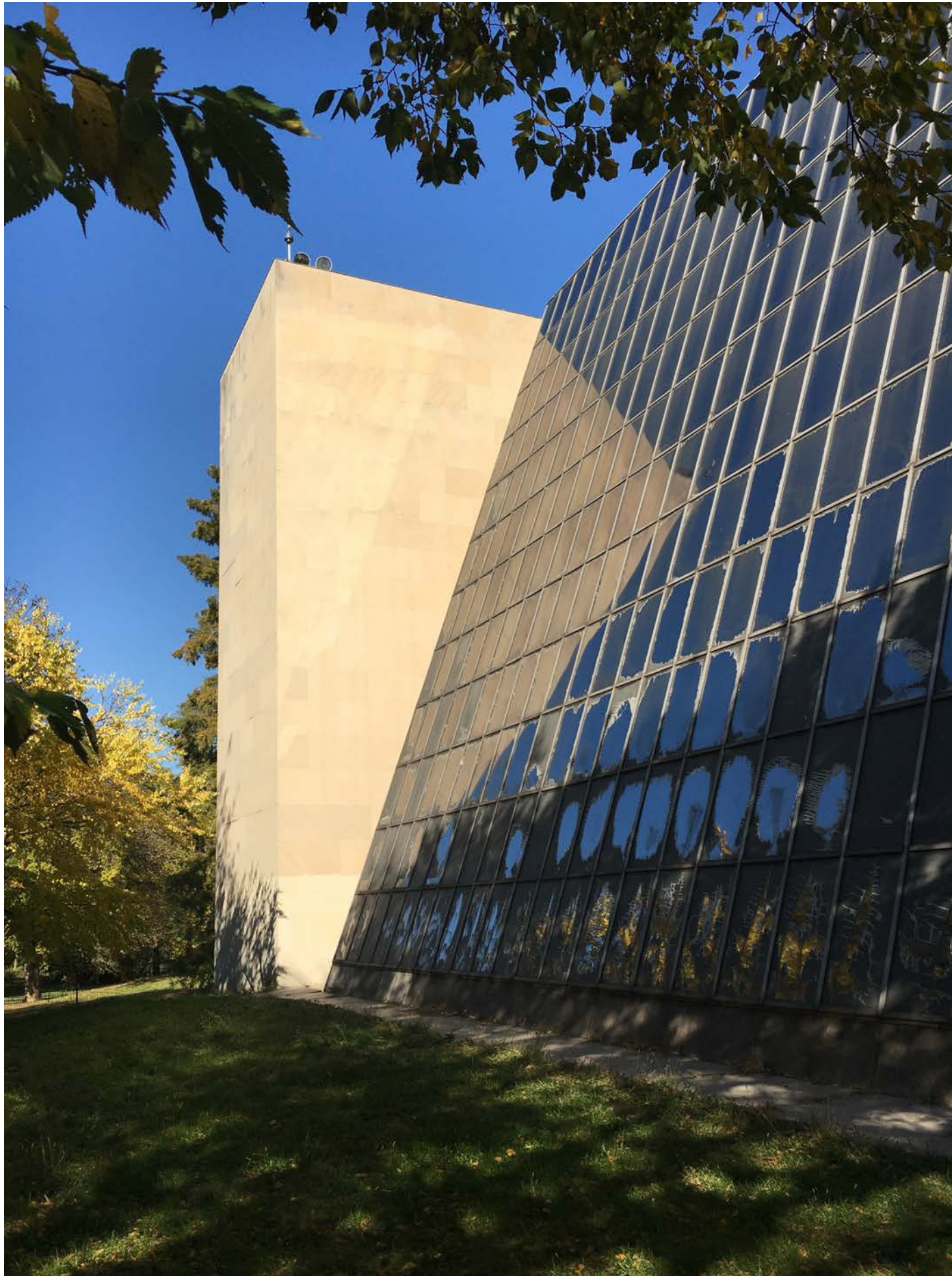
ROCKEFELLER WING - EXISTING CONDITION PHOTOS
