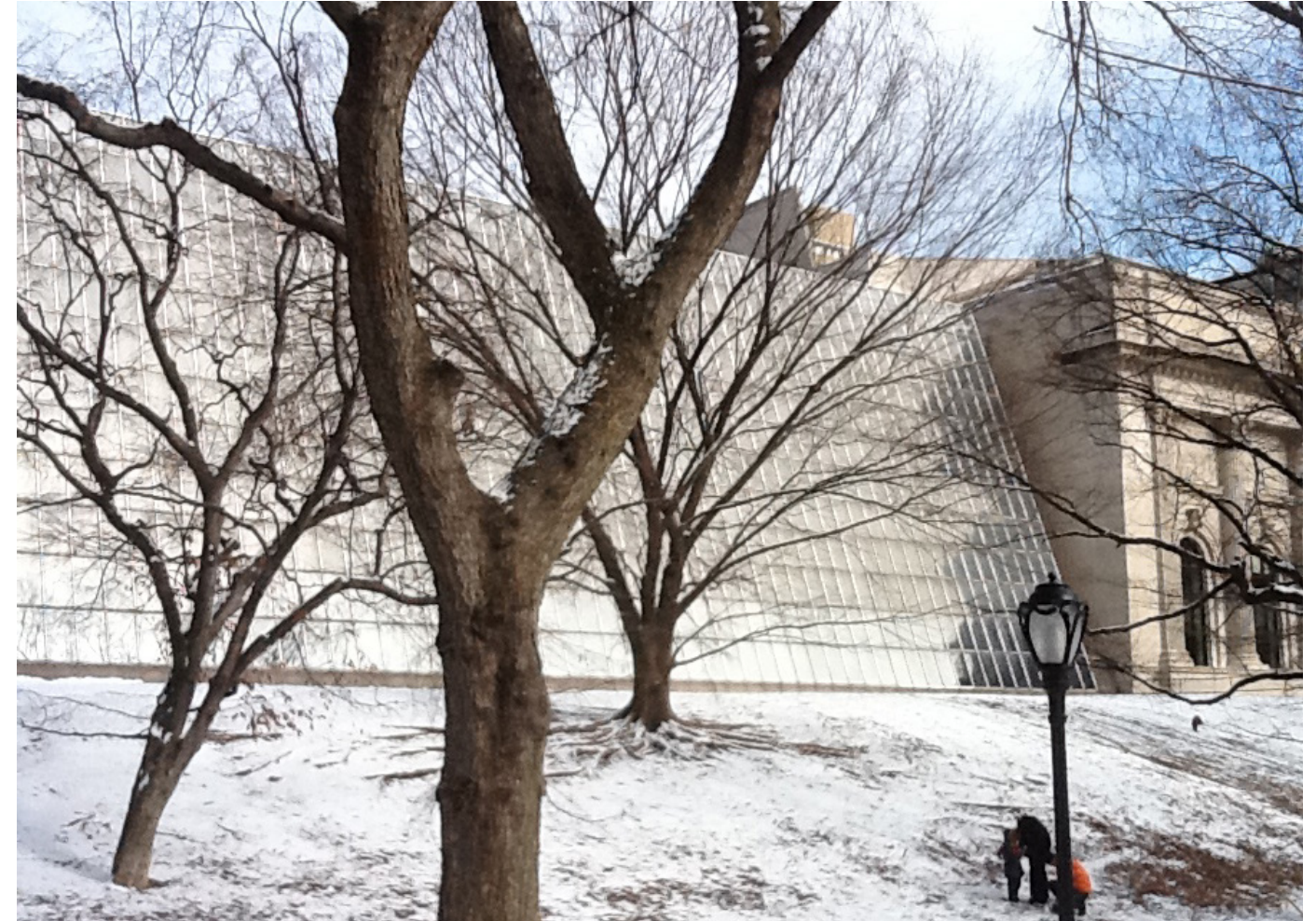
PHOTO OF ORIGINAL CONDITION, 1980'S
