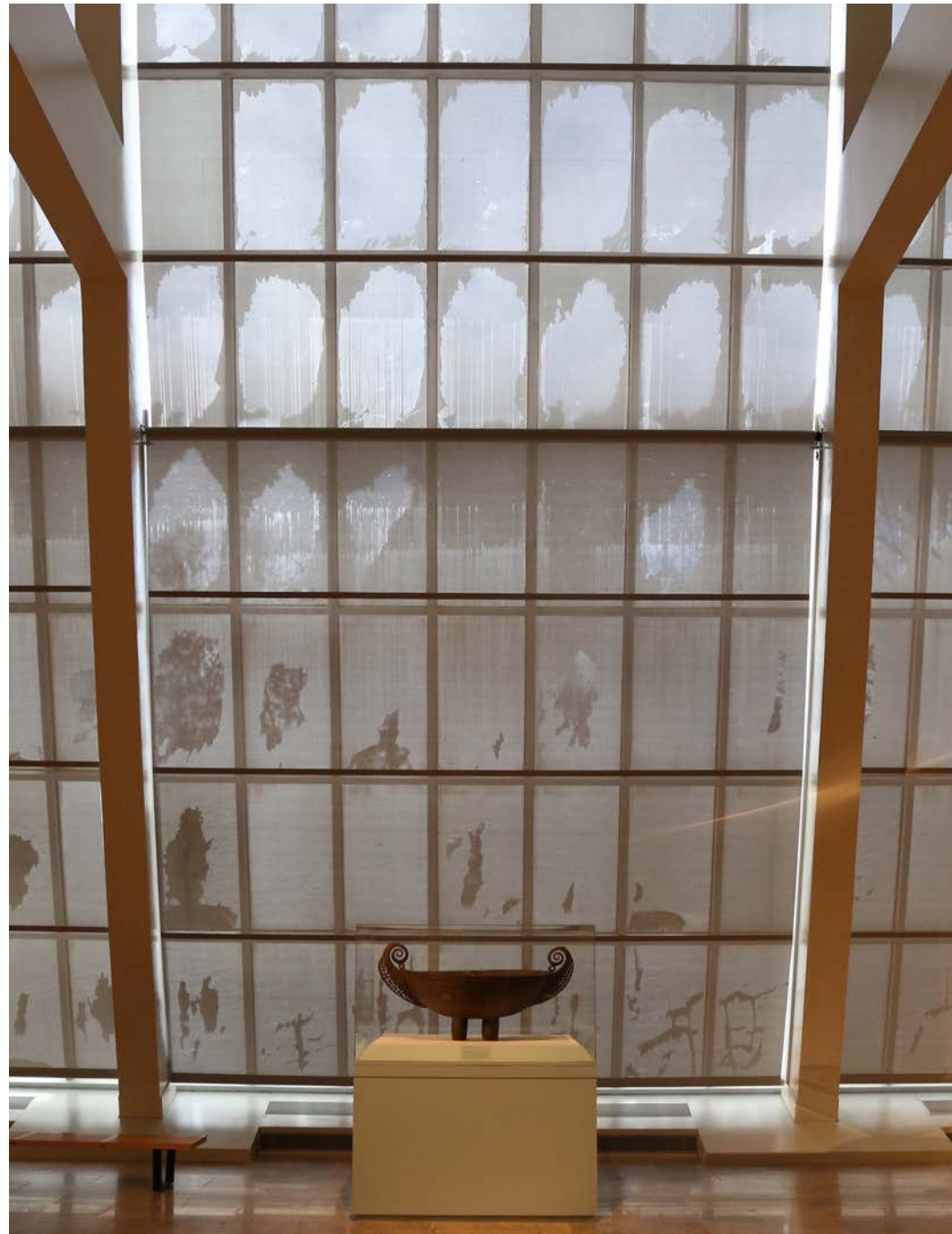
EXISTING CONDITION VIEW FROM FIRST FLOOR INTERIOR OF AAOA GALLERIES
