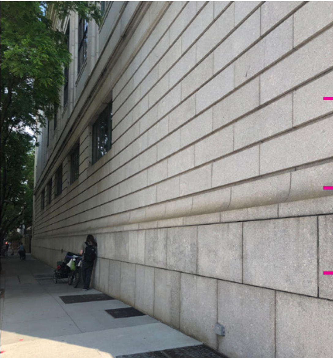
EXISTING SOUTH FACADE AT BUILDING BASE
