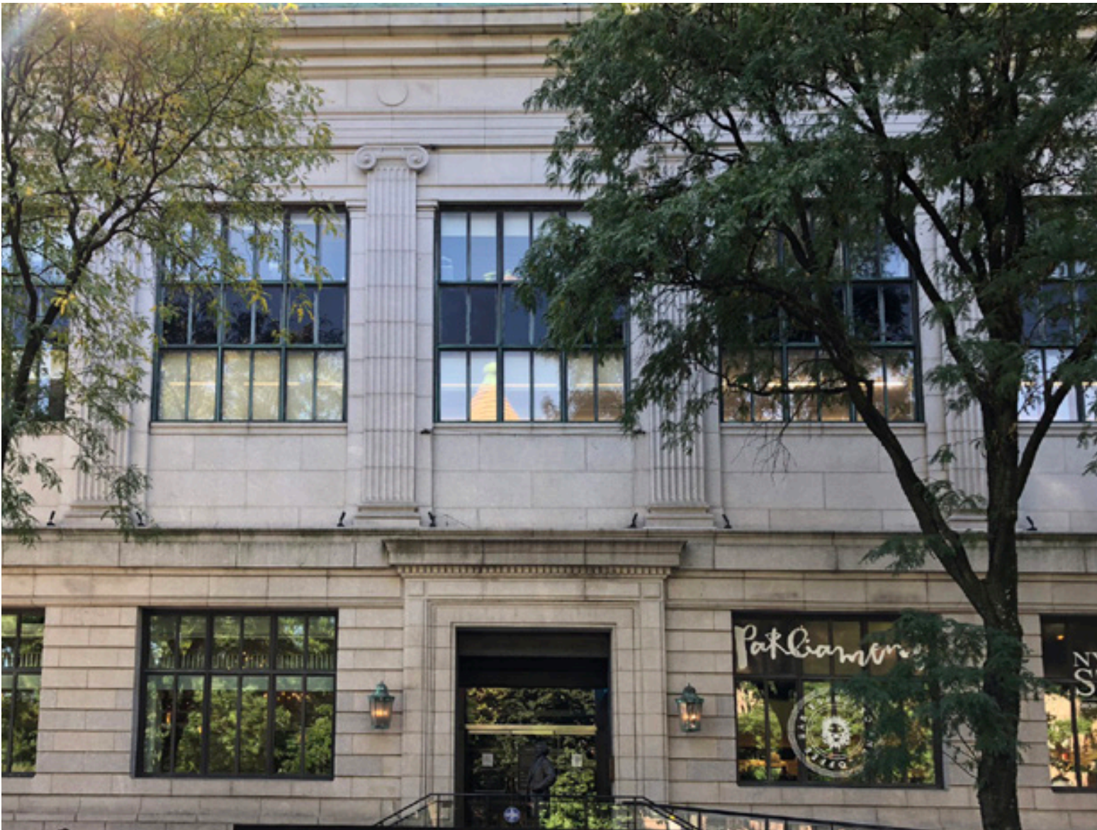
NORTH FACADE ALONG 77TH STREET
