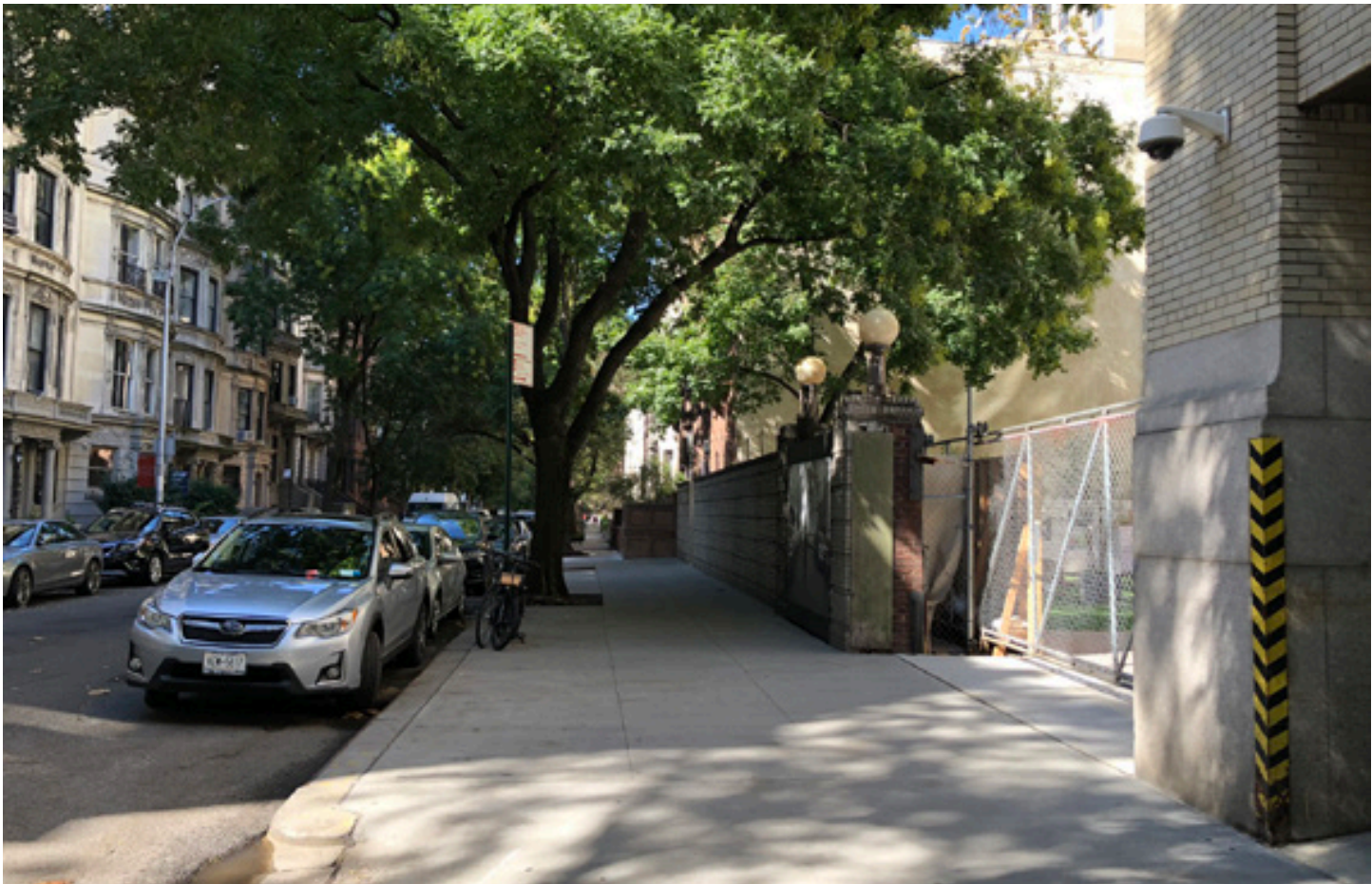
SERVICE YARD WALL AND GATE
