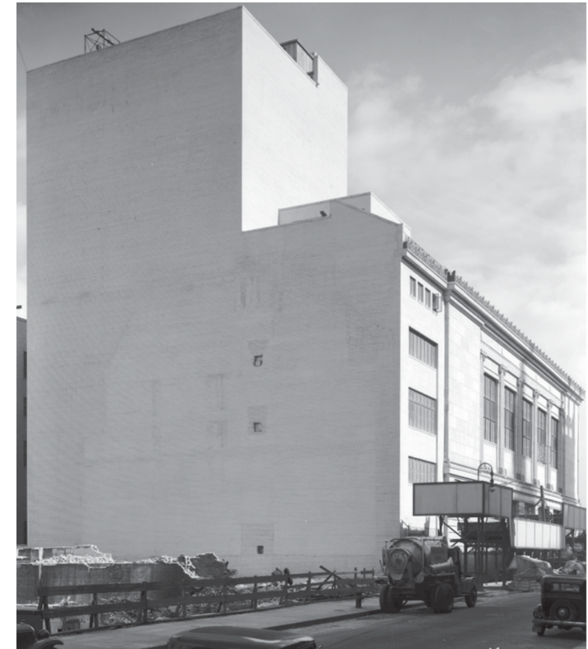
ADDITION UNDER CONSTRUCTION, 1938. N-YHS.
