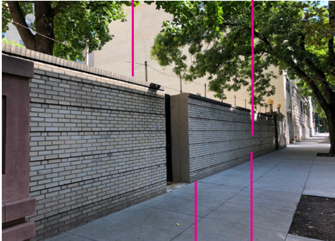
SERVICE YARD WALL, LOOKING EAST
