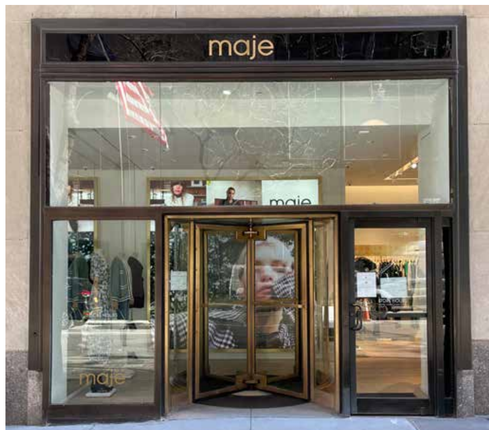
610 5th Ave. 49th St. Entry
