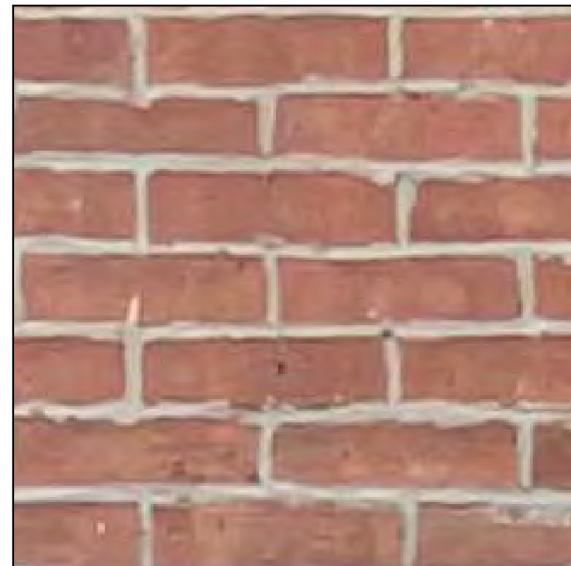
Existing Brick - North
