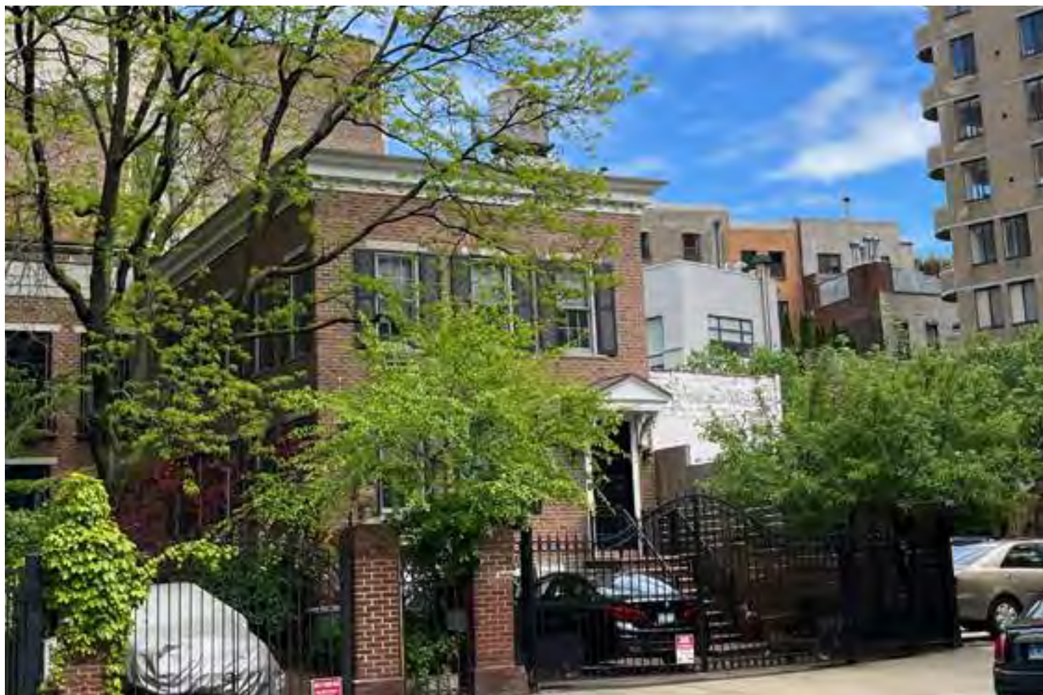
Charles Lane and Washington, looking southeast. Rear and side elevations visible over shorter buildings
