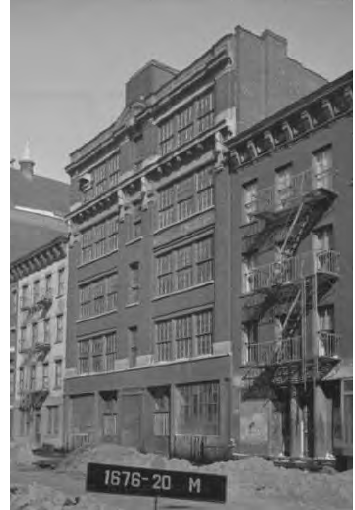
343-345 East 104th Street 1911, Thomas H. Styles ca. 1940 Tax Photo, NYC Municipal Archives
