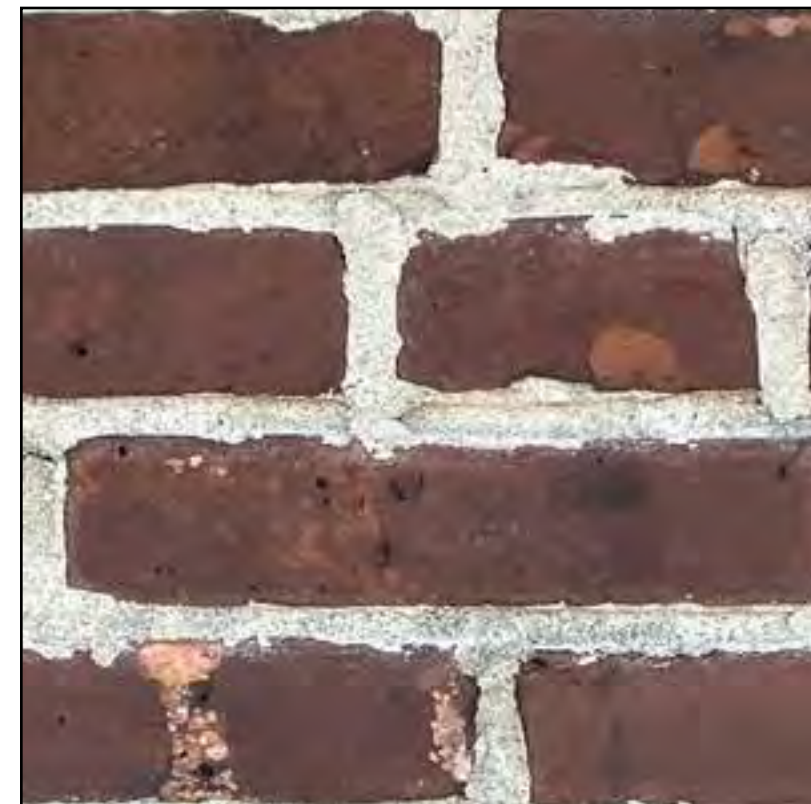
Existing Brick - East & West
