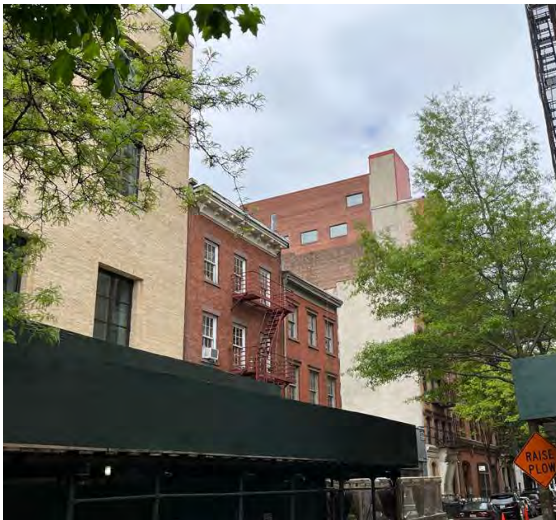
Perry Street, looking east, showing rooftop addition at 131 Perry Street
