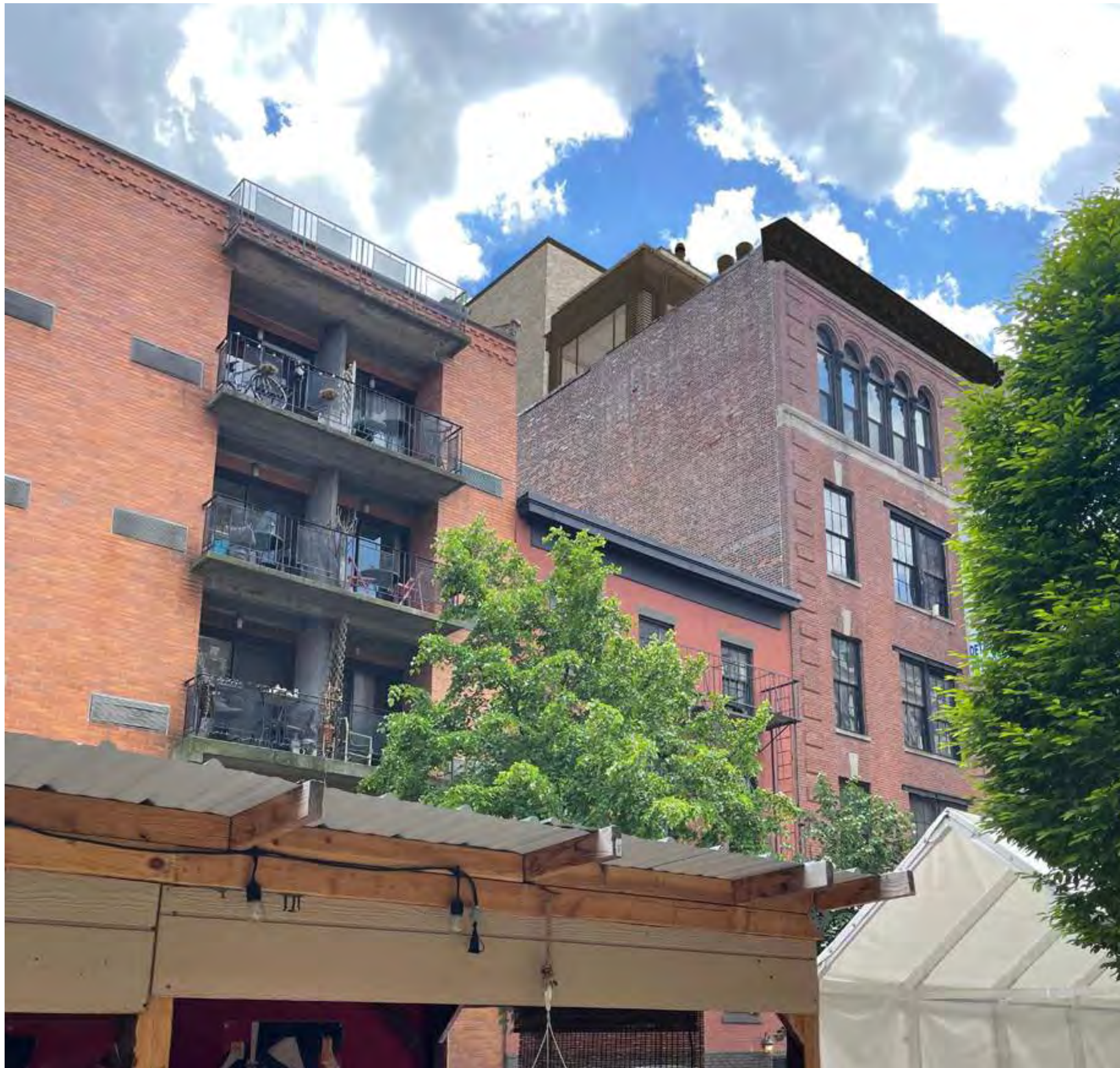
West 11th Street, accross from 330 West 11th . Proposed Addition VIEW 5
