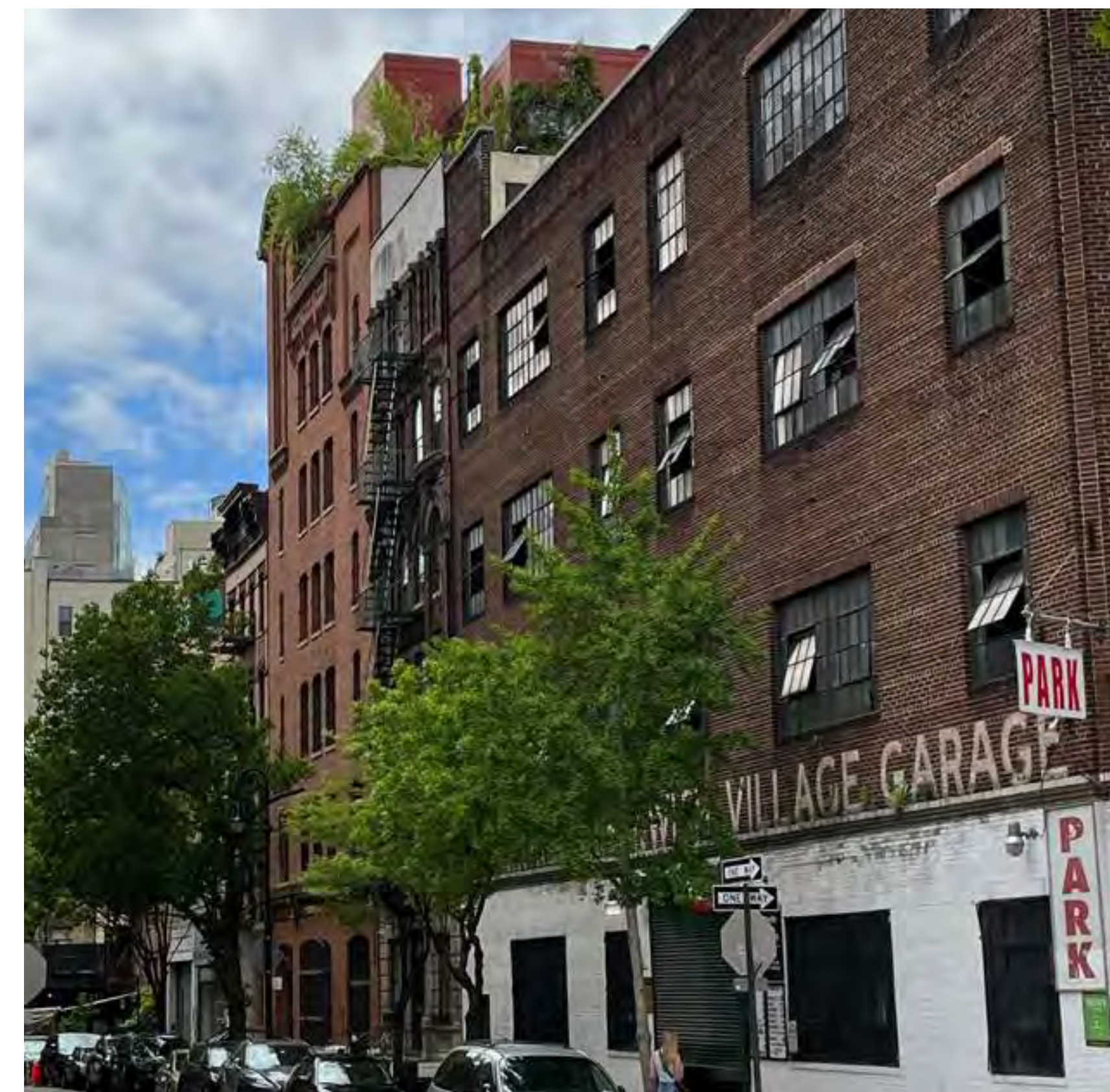
Perry Street, looking west, showing rooftop addition at 131 Perry Street
