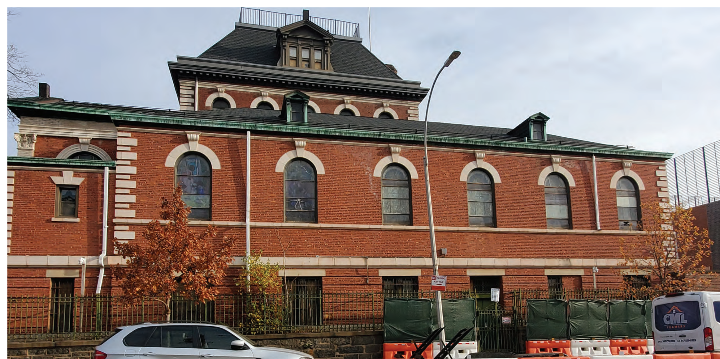
SOUTH SIDE 64TH STREET WING, LOOKING NORTH
