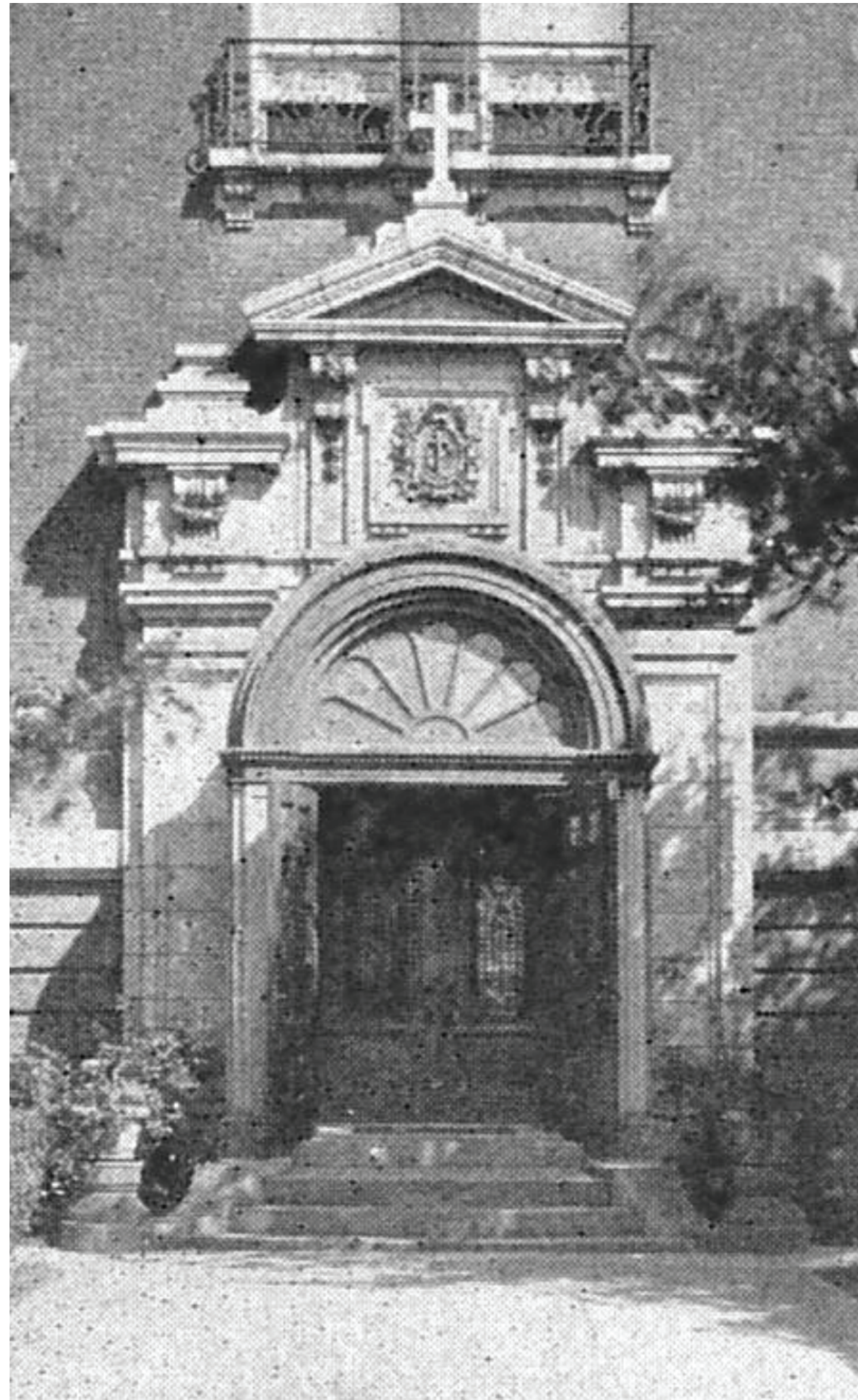
FORMER MAIN ENTRANCE DOUBLE DOORS
