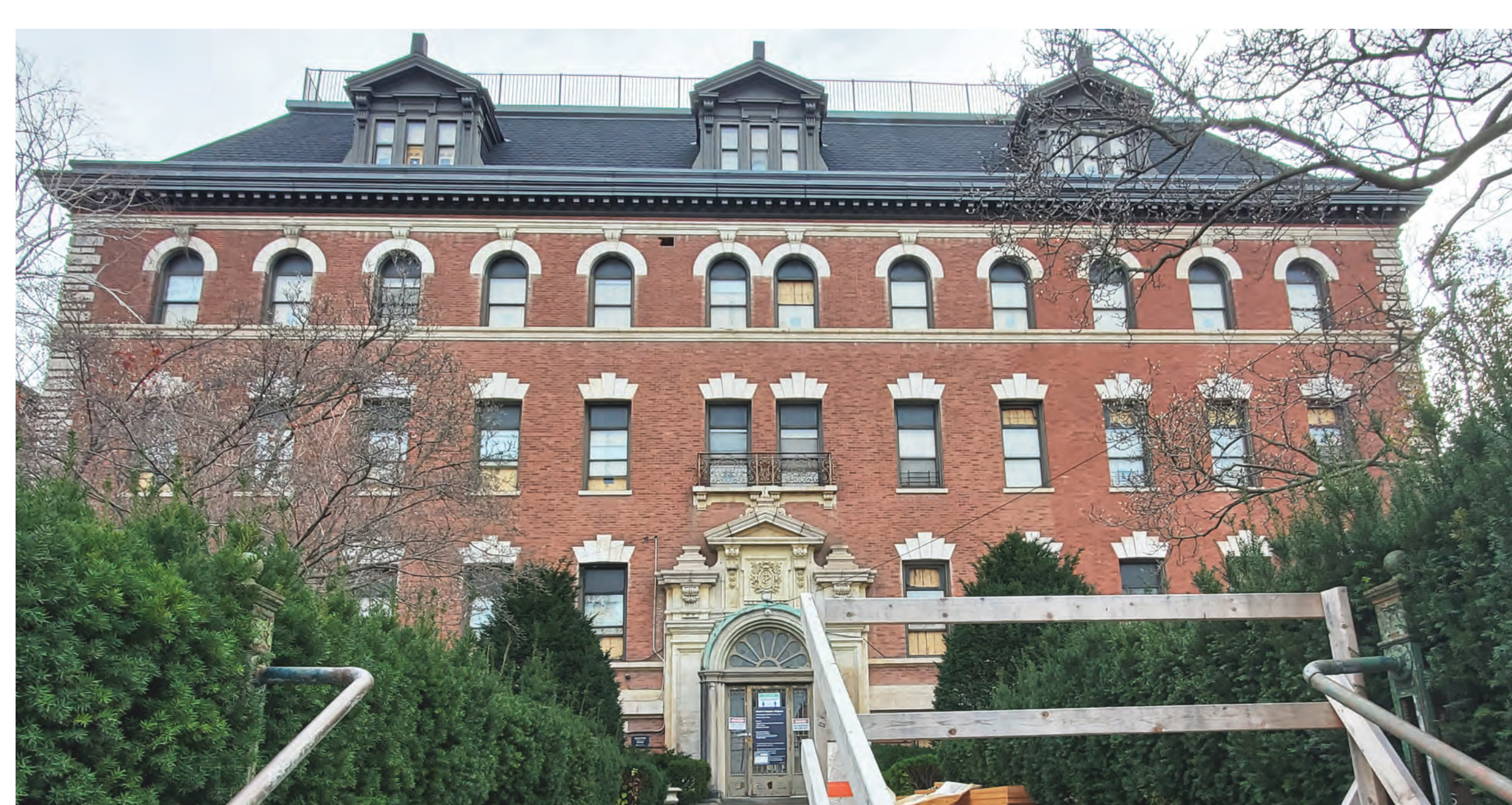
WEST SIDE 12TH AVE MAIN BUILDING, LOOKING EAST
