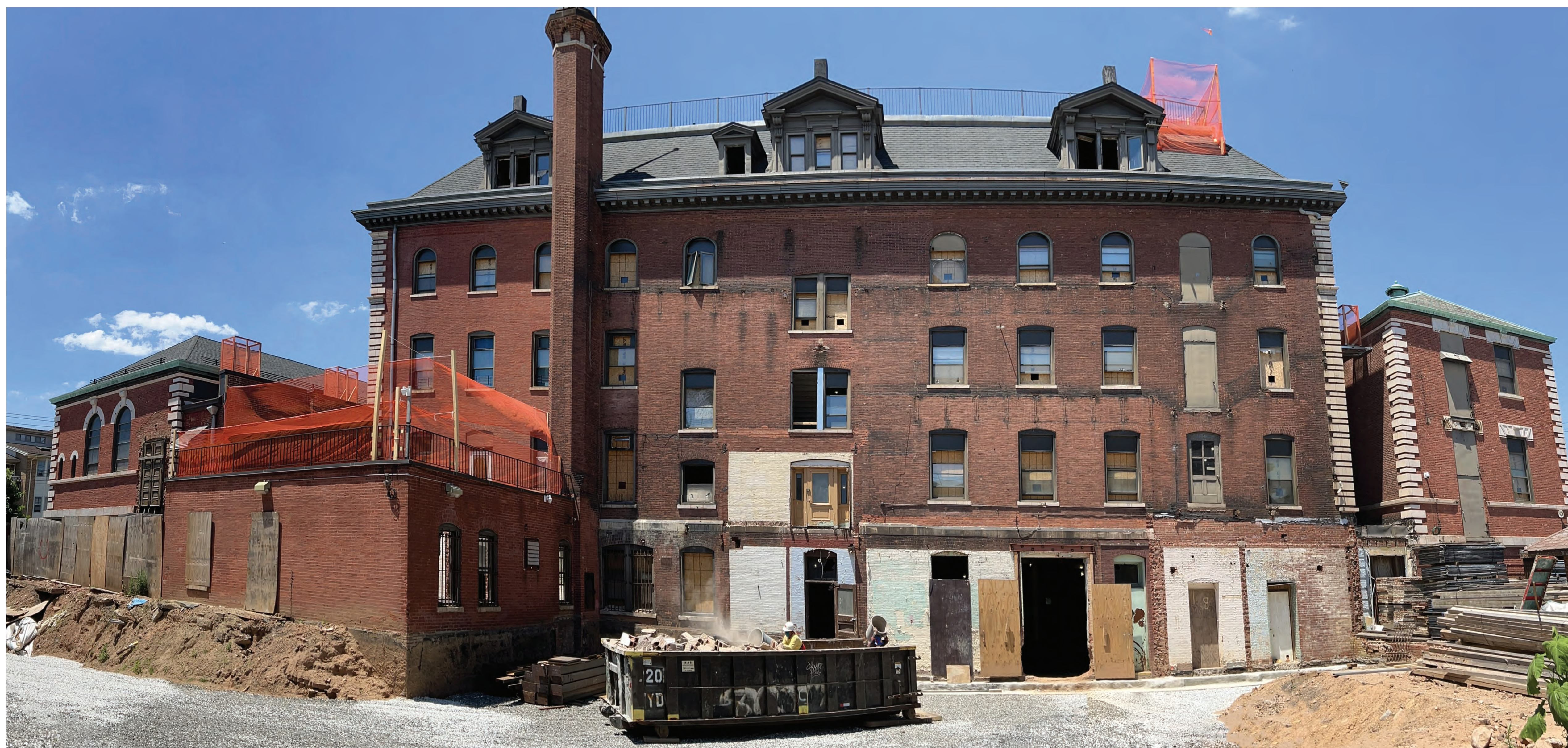
EAST SIDE REAR FACADE, LOOKING WEST
