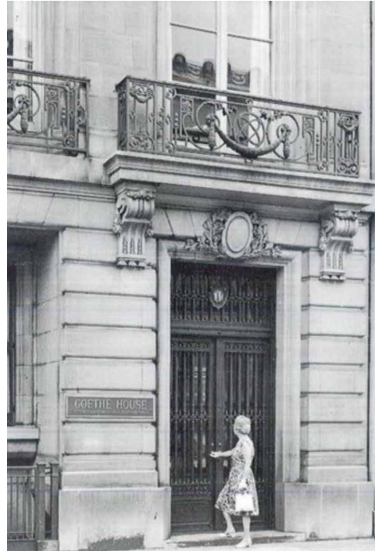
1920s — new door when stoop was removed
