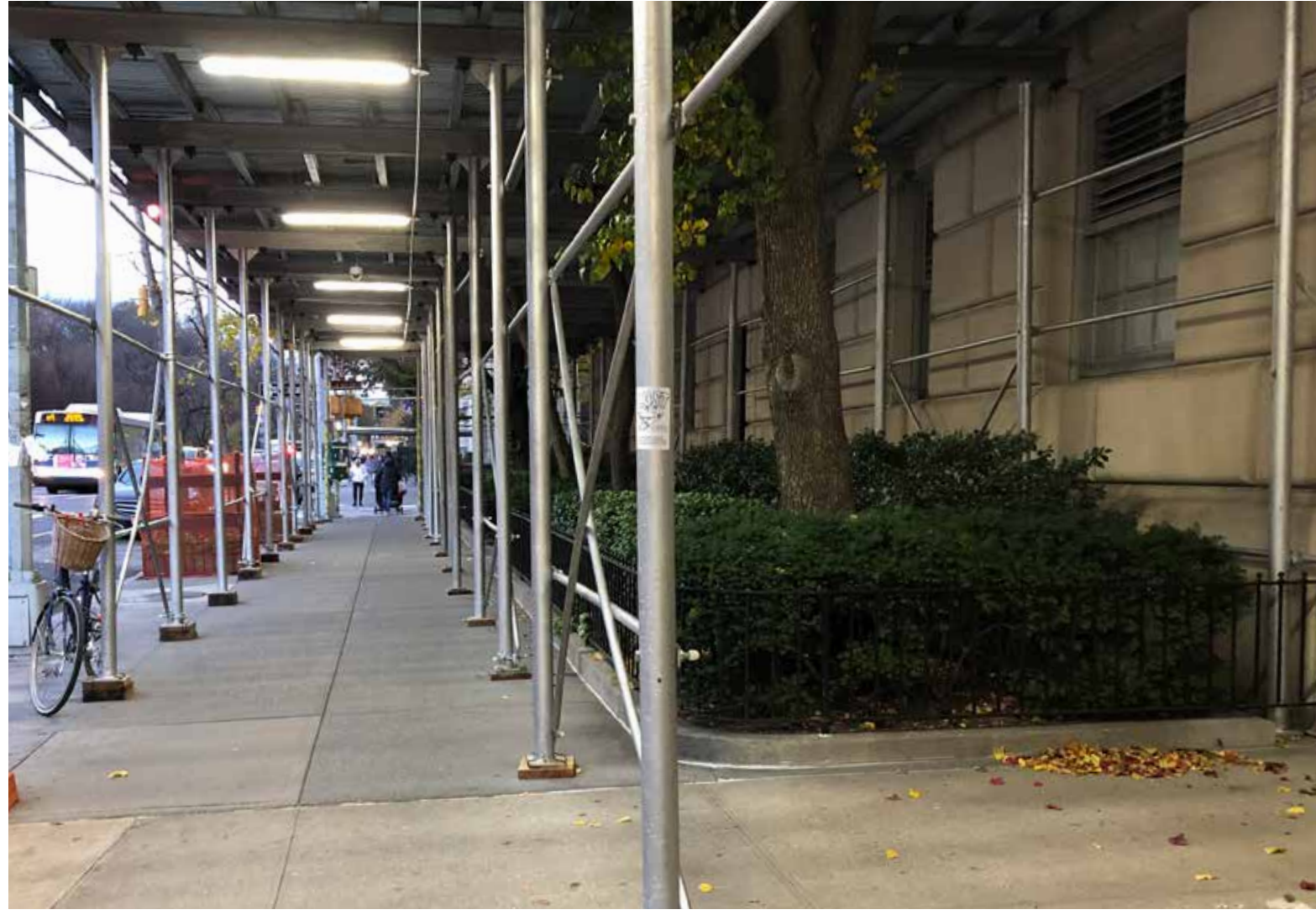
1. 1016 5th Ave planter and fence
