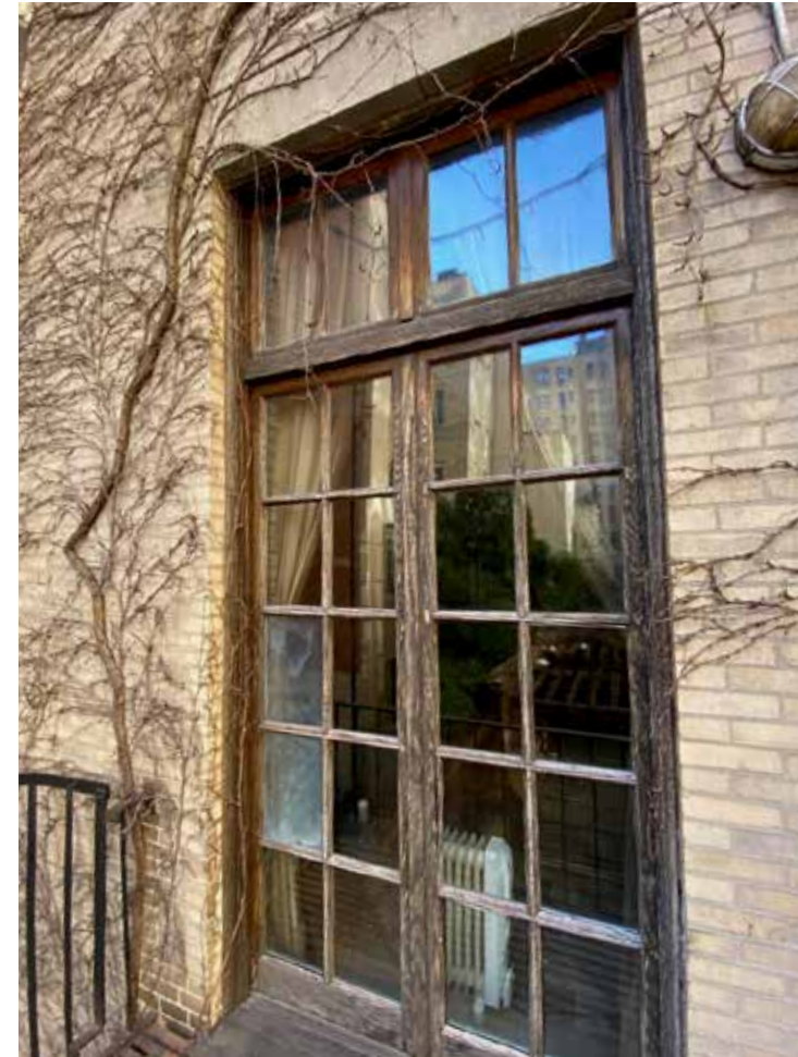
Existing stained clear-coated wood windows to be replaced in kind
