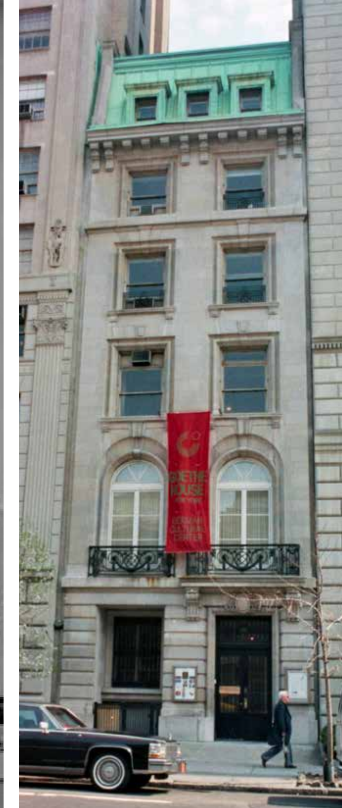
1980 — photograph showing later alterations to upper windows
