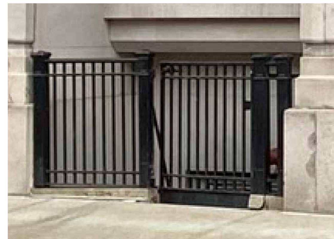
Cellar stairs gate
