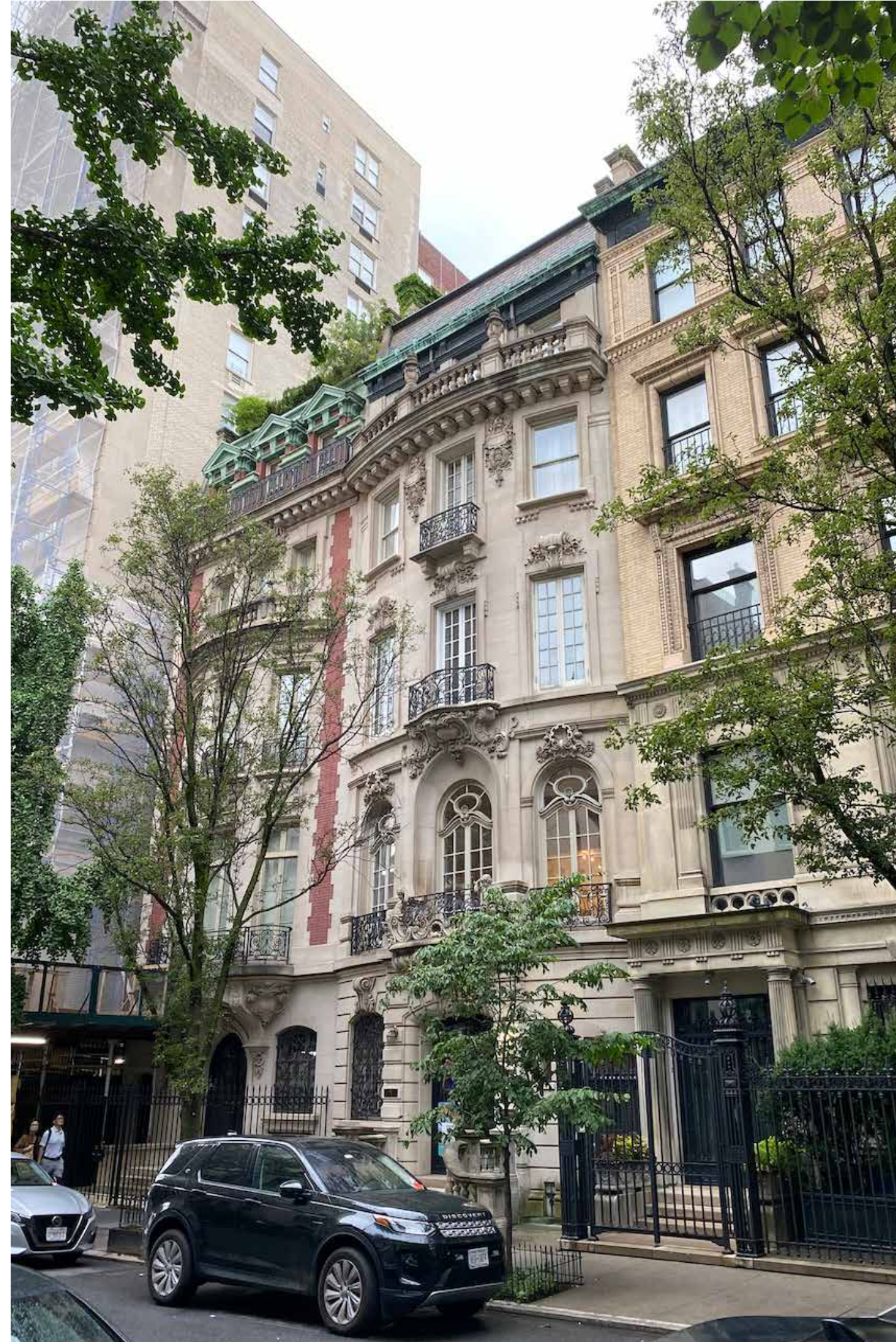
VP2 — View towards Northwest from E82nd street (No's 1, 3, 5 and 7 E82nd street in view)
