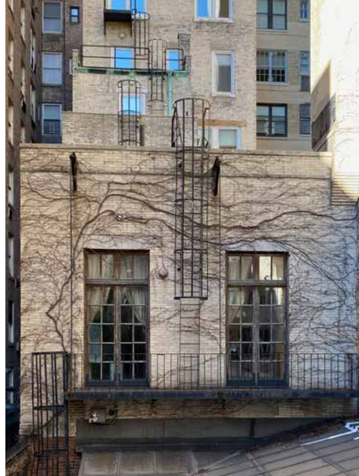
Existing light brick to second floor and above
