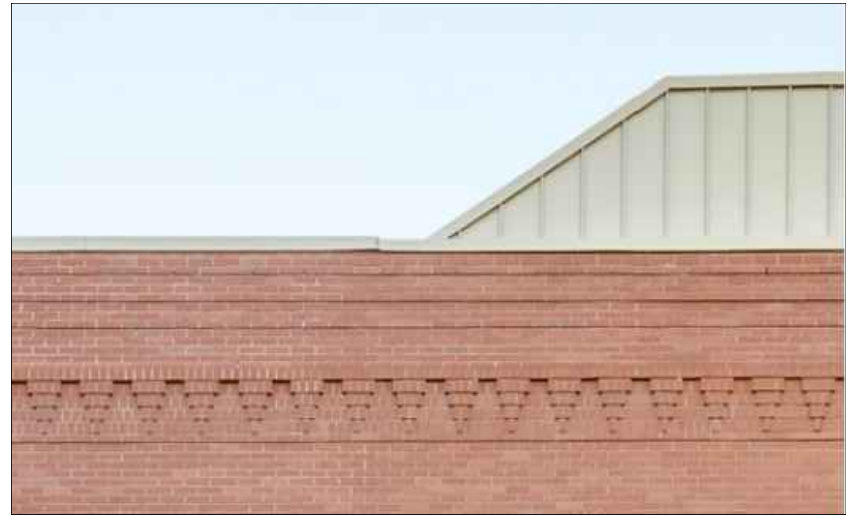
MODERN BRICK STACKED PARAPET, BUILT 2015 259 - 261 BERRY STREET
