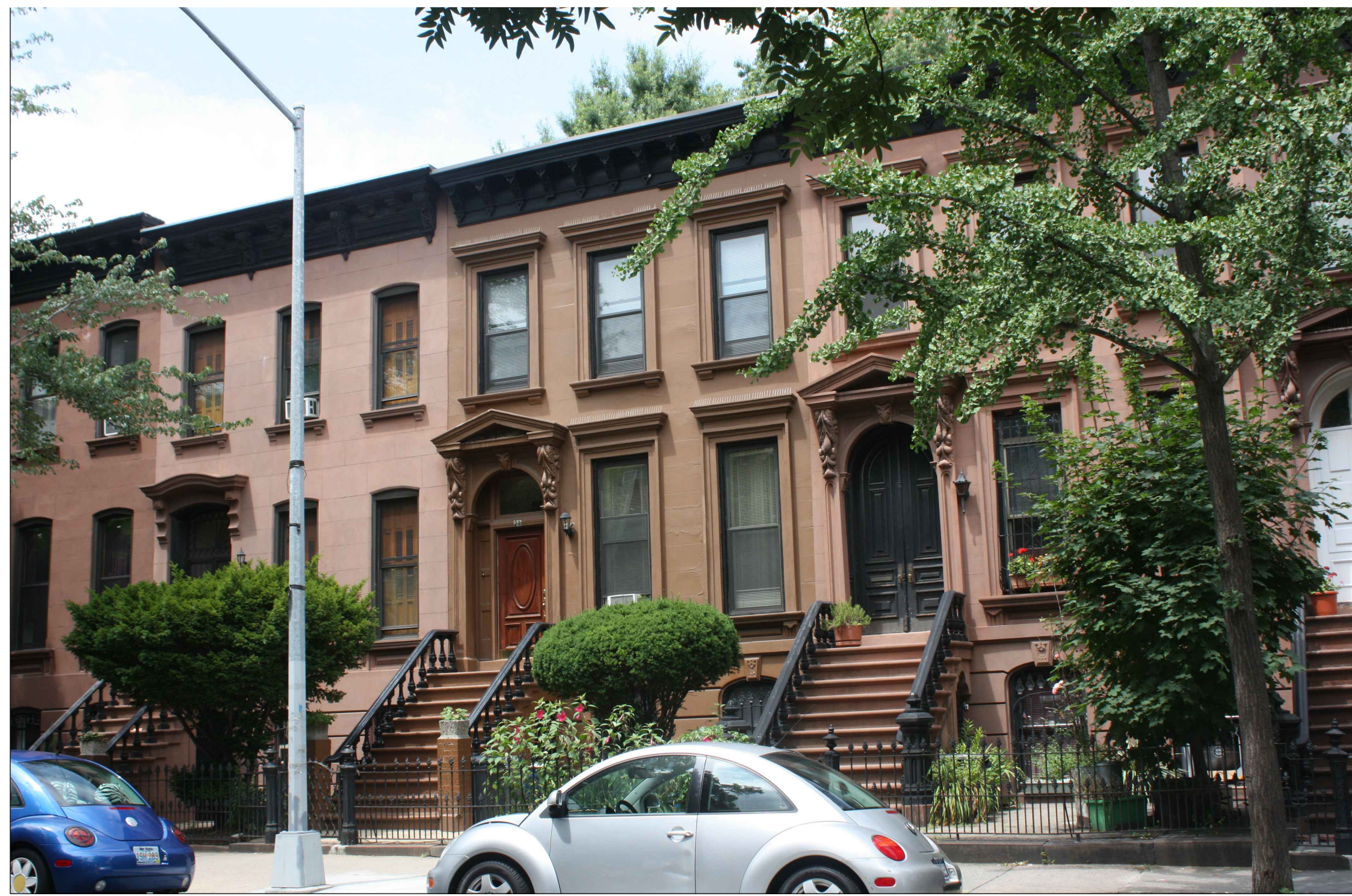
PARAPETS - 29 - 33 CLIFTON PLACE
