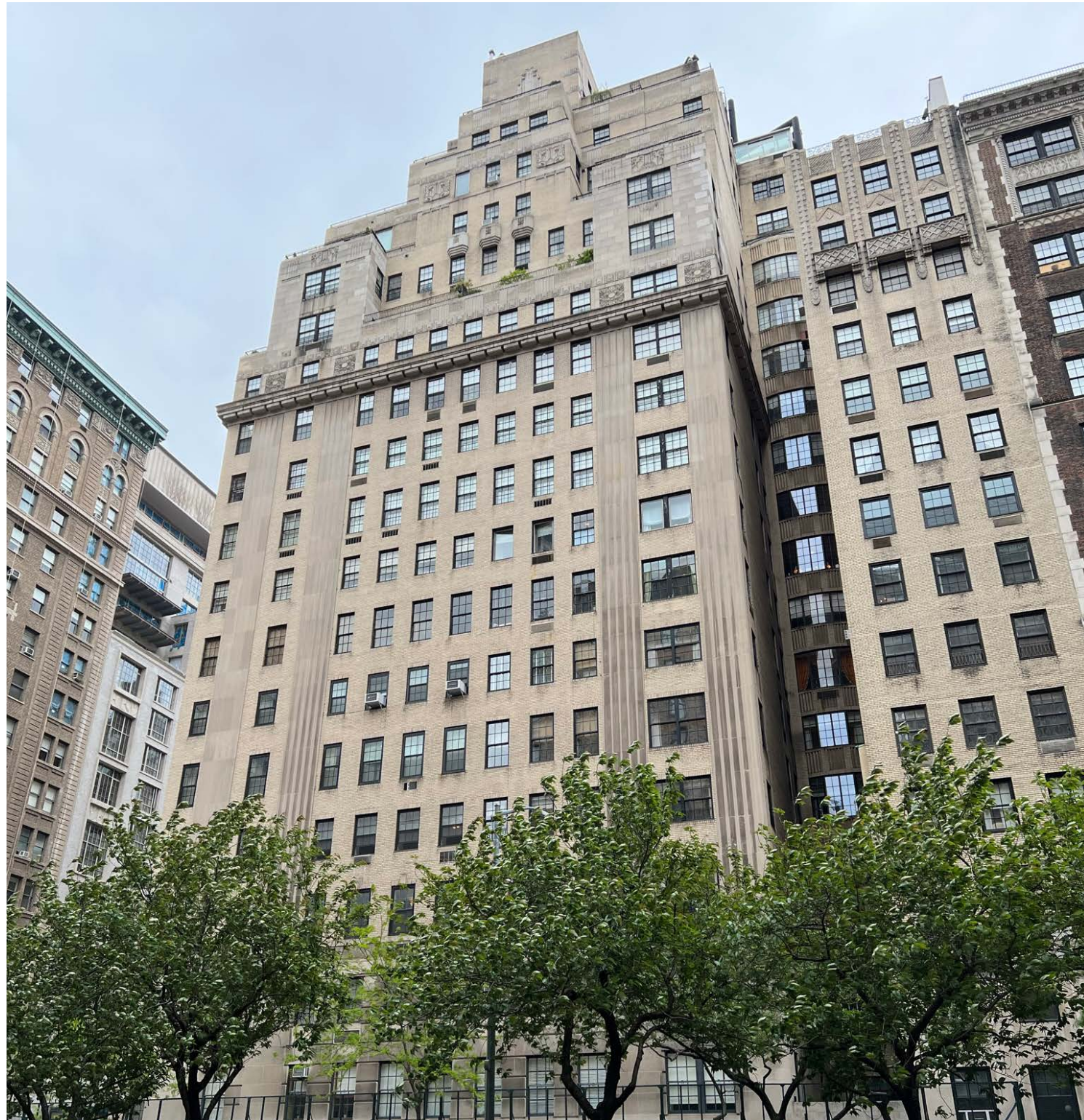
EXISTING WINDOWS AT PARK AVENUE ELEVATION, LOOKING NORTHEAST
