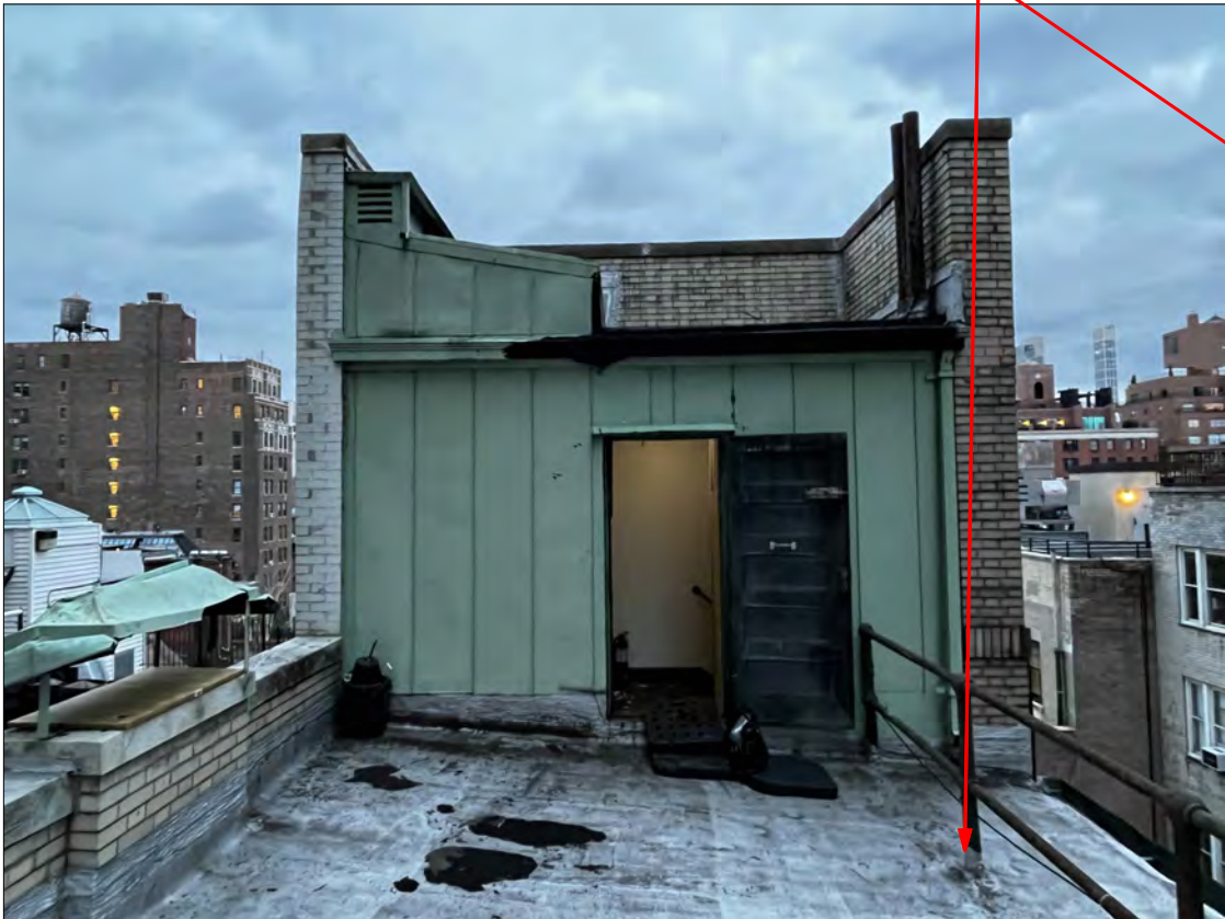
2: ROOF BULKHEAD LEVEL - COPPER CLAD BULKHEAD FOR REAR SERVICE STAIRWELL
