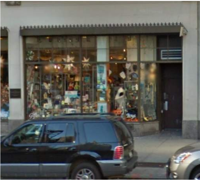
WEST ENTRANCE - EXISTING CONDITION (TAKEN OCTOBER 2014)
