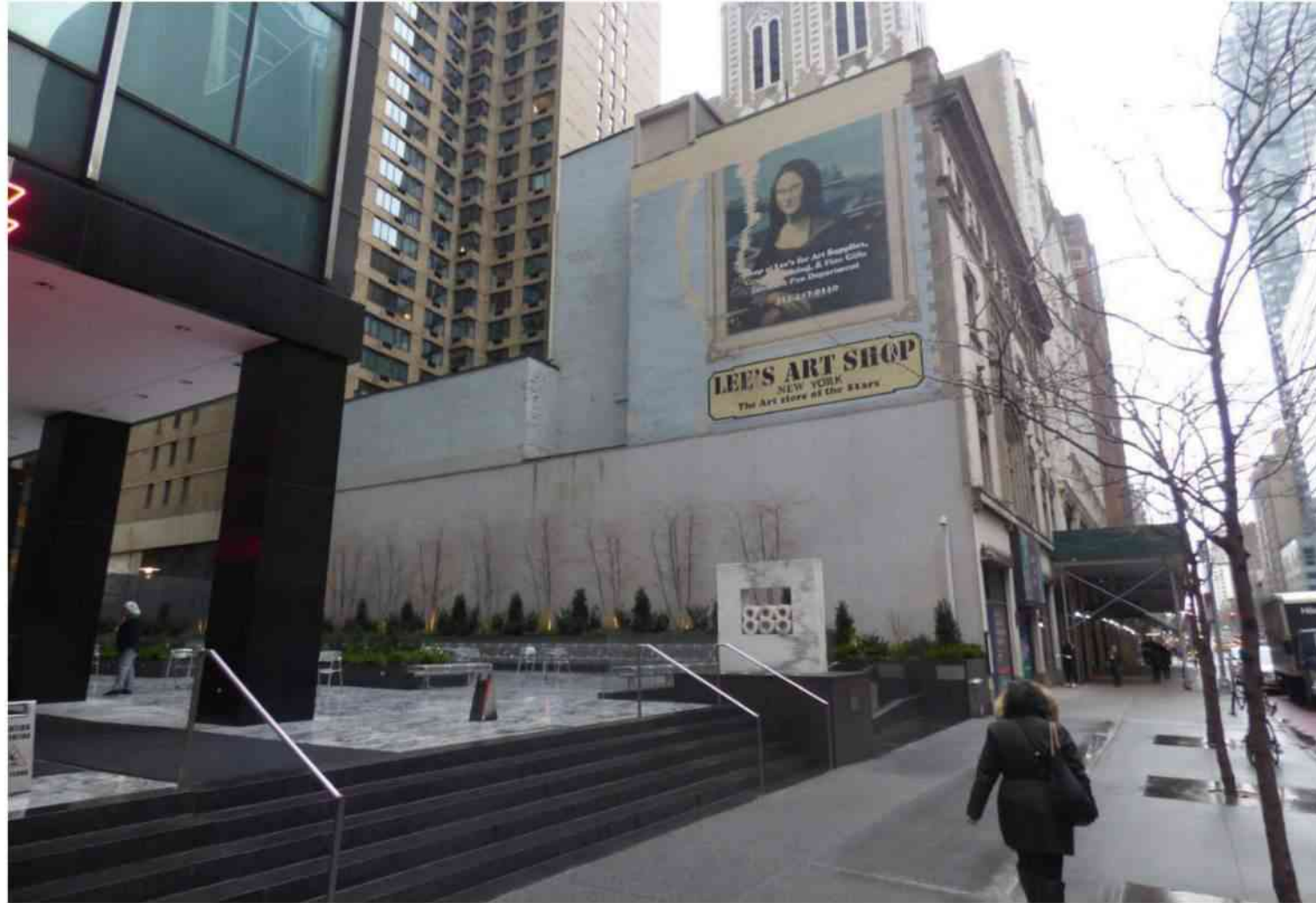
EXISTING CONDITIONS 218 WEST 57TH STREET
