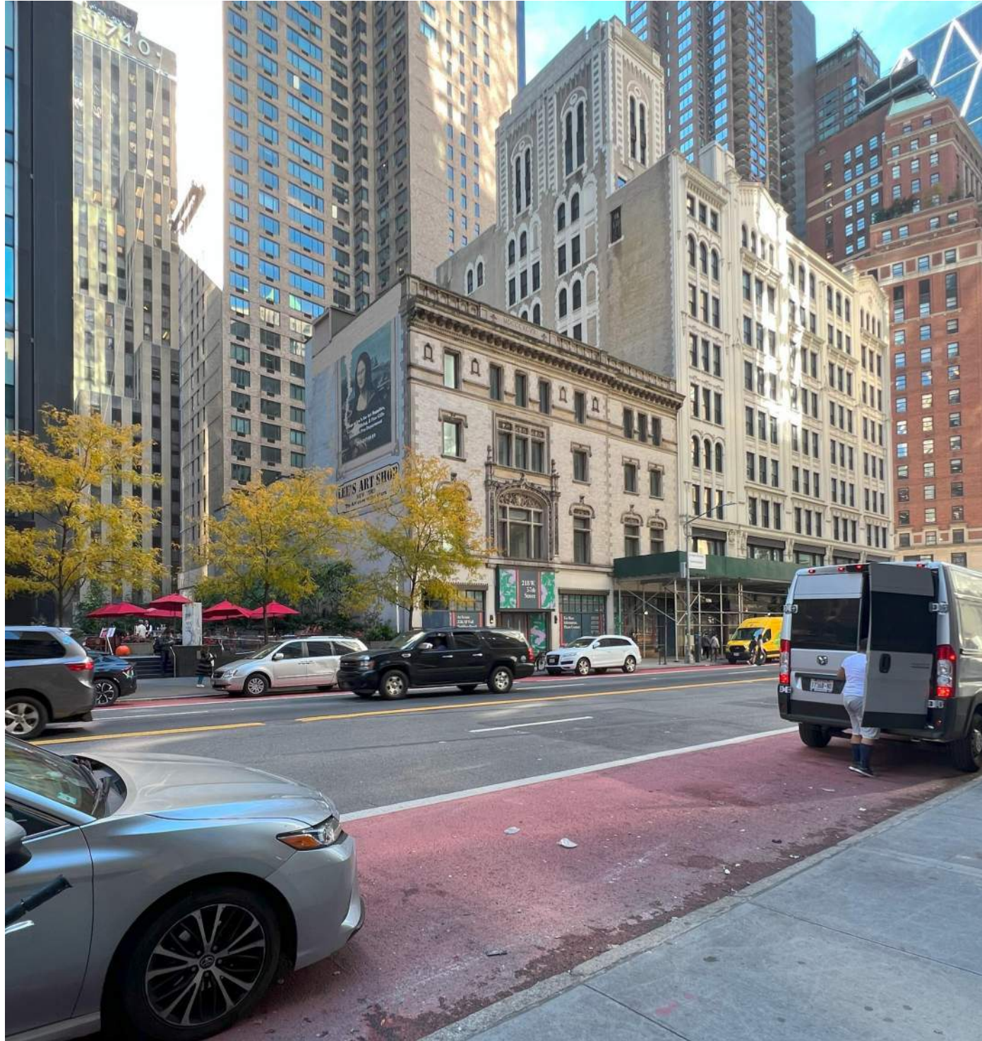
EXISTING CONDITIONS 218 WEST 57TH STREET
