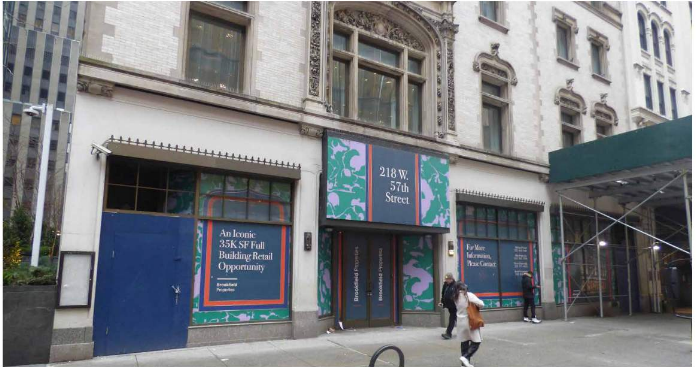
EXISTING CONDITIONS 218 WEST 57TH STREET
