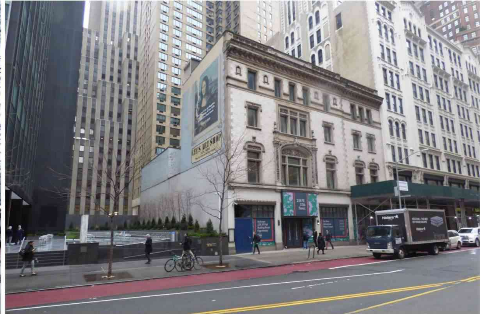
EXISTING CONDITIONS 218 WEST 57TH STREET
