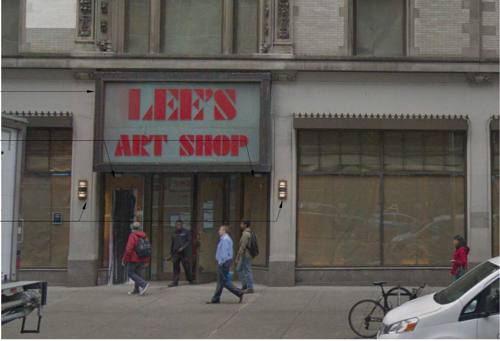
PRIMARY SIGN BOARD - EXISTING CONDITION (TAKEN AUGUST 2018)
