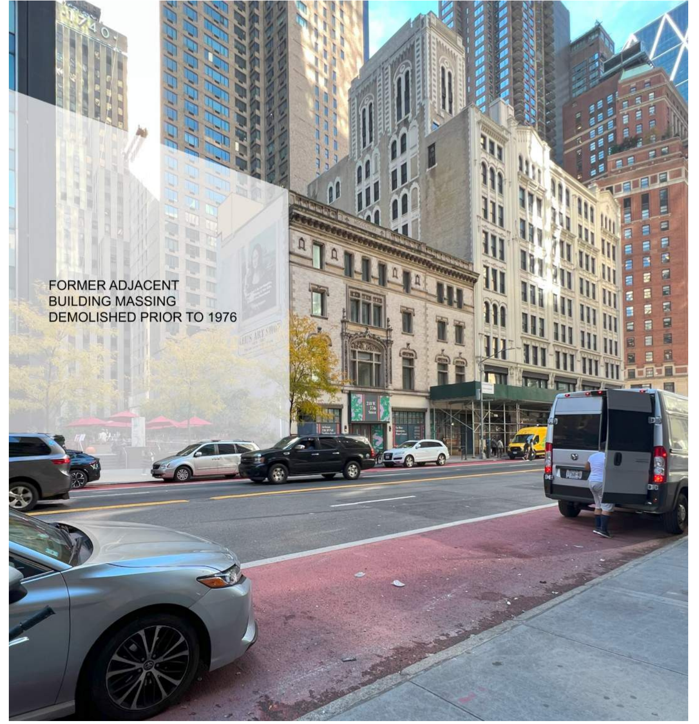
HISTORIC CONDITIONS 218 WEST 57TH STREET
