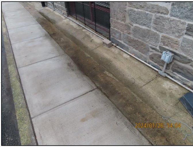
Existing walkway at south side of courtyard
