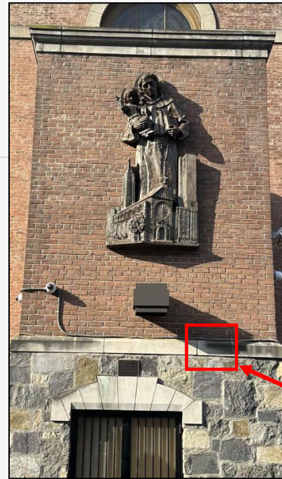
Existing Sign at Elevator Bulkhead
