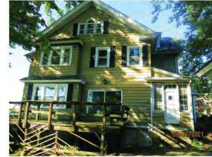
② EXISTING SIDE VIEW OF PORCH FROM SHORE ROAD SCALE: \frac{1}{4}"=1'-0"
