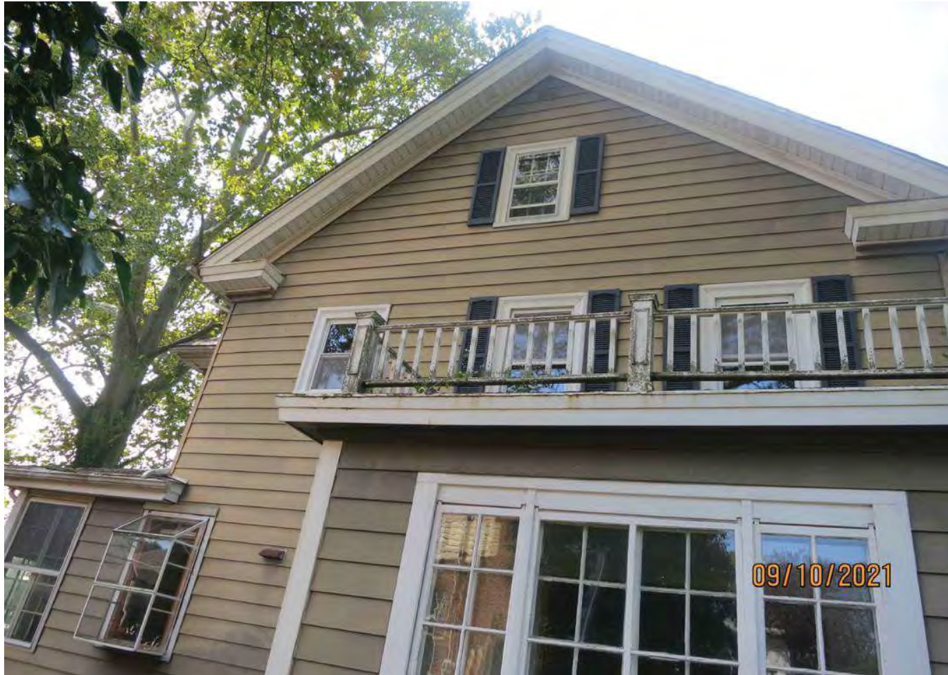
④ EAST SIDE VIEW FROM DRIVEWAY SCALE: N.T.S.
