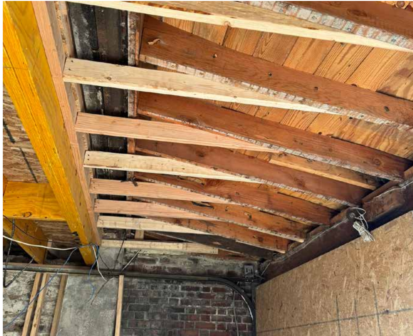
EXISTING EXTENSION AREA FROM BELOW
