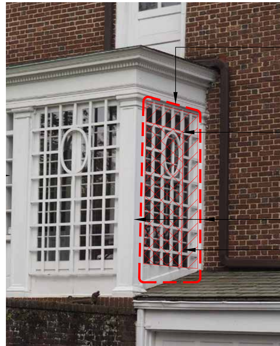
PHOTO - AREA OF EXTERIOR WORK
