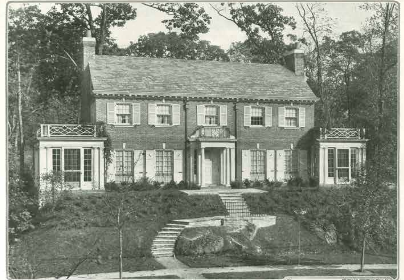
A combination of Georgian and New England Colonial has been used in the home of John W. Griffin, at Fieldston, New York City. It is executed in brick and the roof is slate of varied sizes and colors. Cream white paint has been used on the exterior woodwork. To lend a touch of contrast, wrought iron is employed on the balcony over the entrance and at the lower windows. As in the case of the other two houses in this group, Dwight James Baum was the architect
