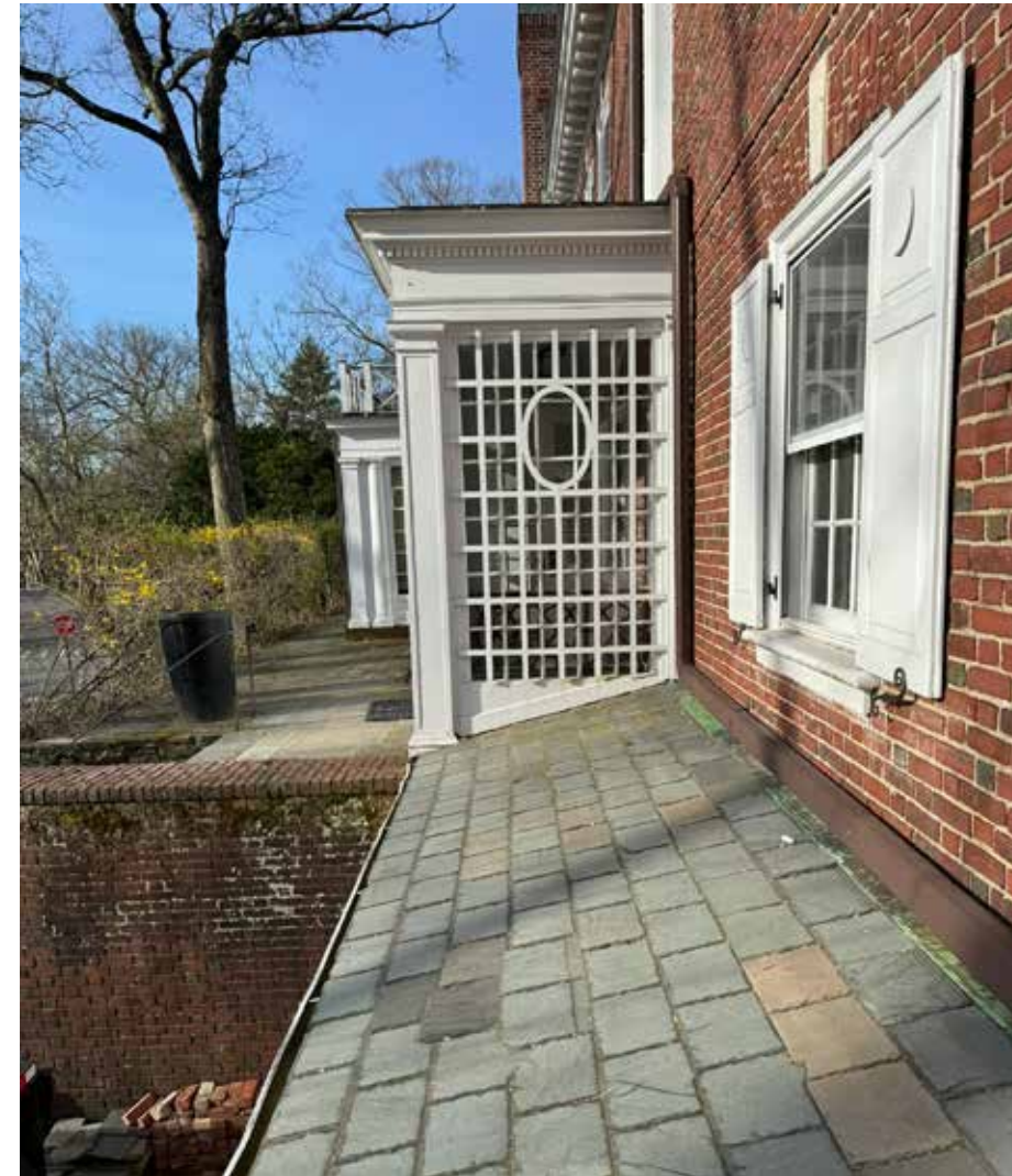
EXISTING SLATE ROOF OVER GARAGE
