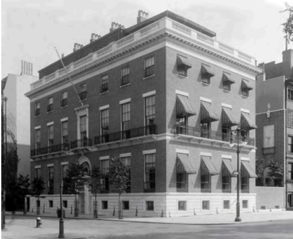
Knickerbocker Club, 2 East 62 nd Street Delano & Aldrich, 1915. (Individual Landmark)
