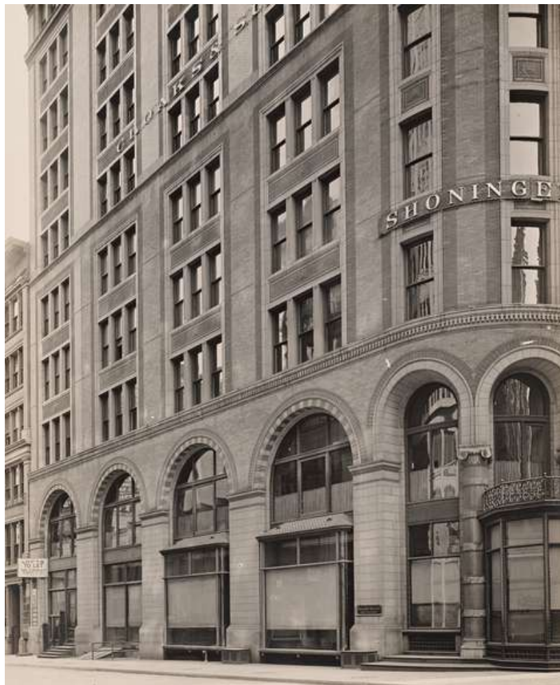
1913: Partial East 20th Street elevation, showing altered storefront bays. (NYPL)
