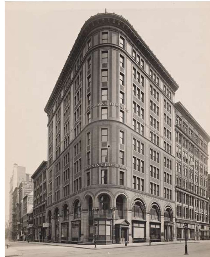
1913: Storefront bays have been altered. (NYPL)
