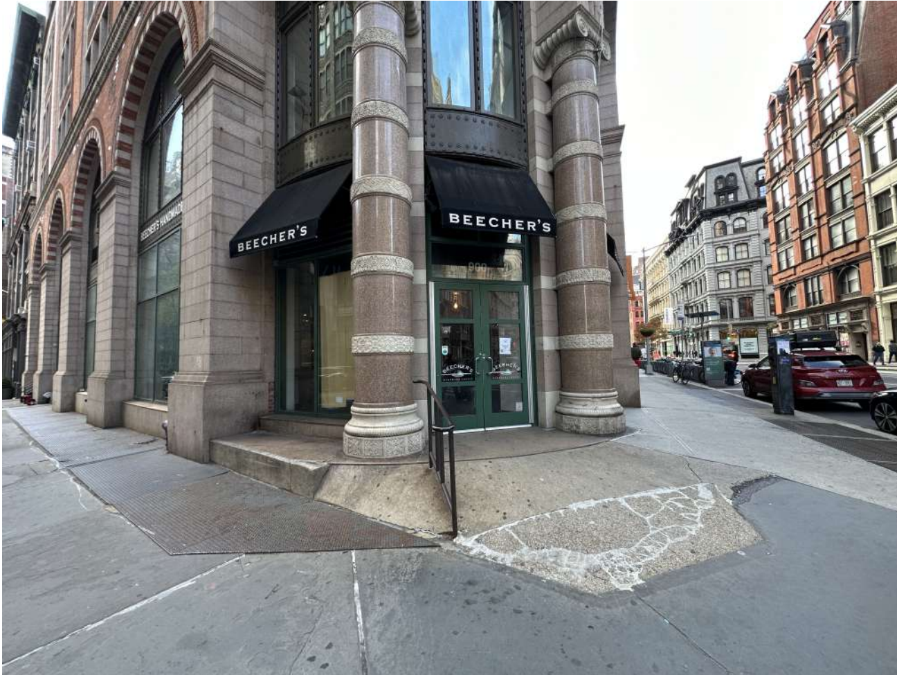
Existing corner condition.
