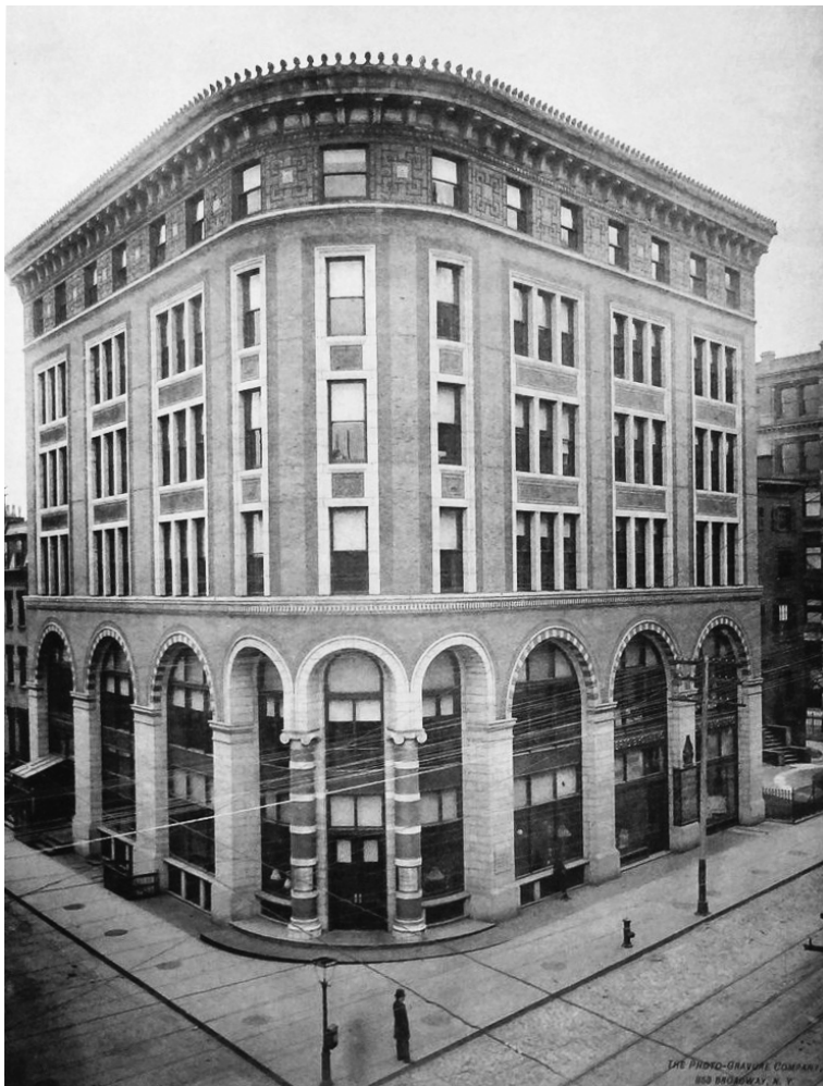
1886: 900 Broadway at southeast corner of Broadway and East 20th Street. (MCNY)
