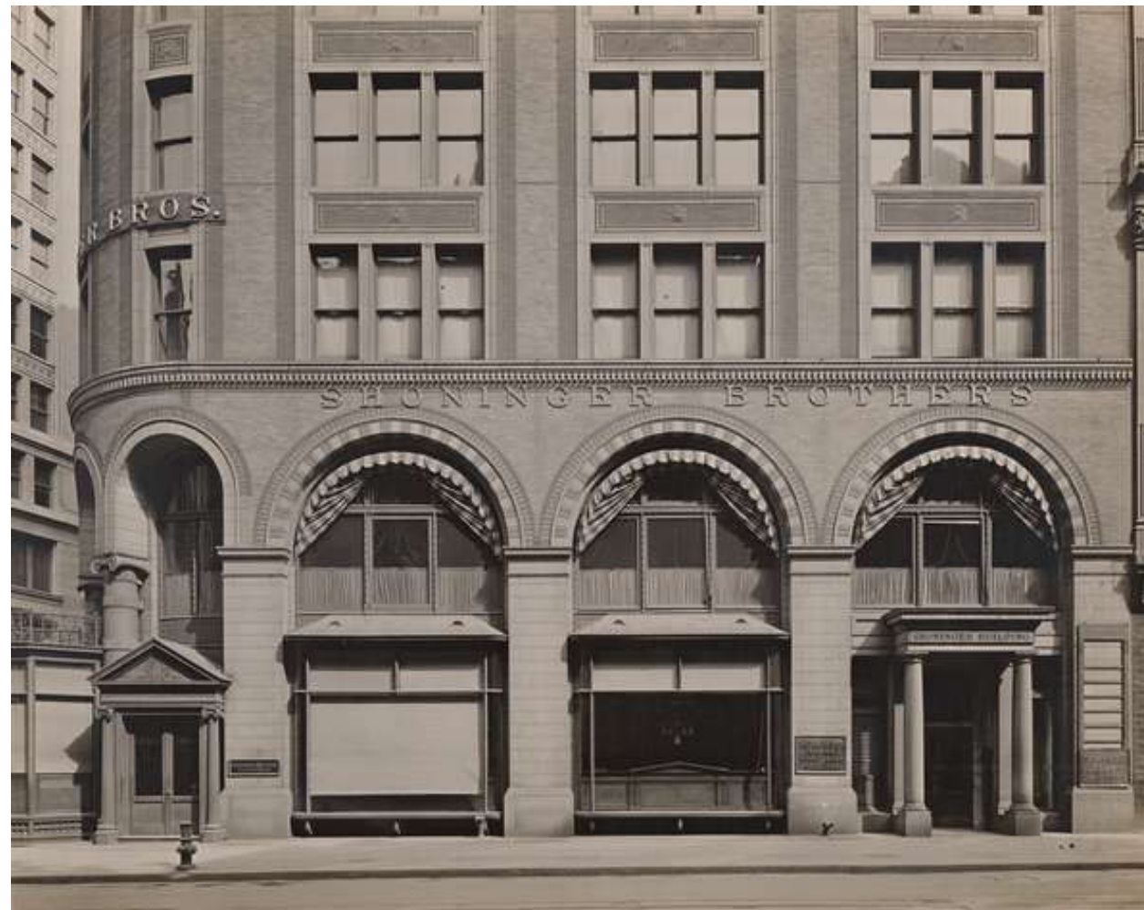
1913: Partial Broadway elevation showing altered storefronts. (NYPL)
