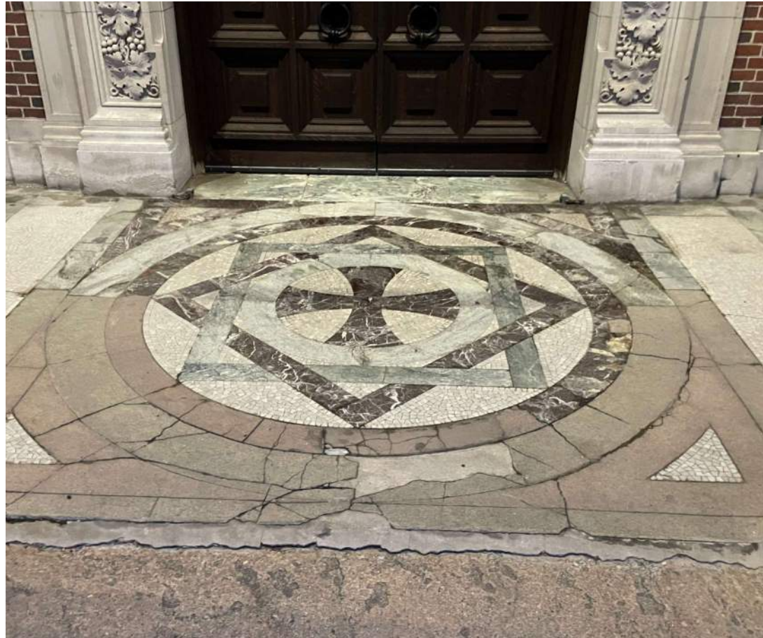
PORTICO LOOKING EAST
