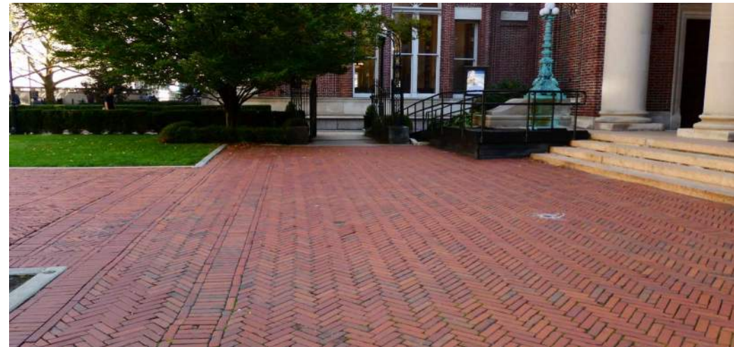
WEST PLAZA LOOKING NORTH
