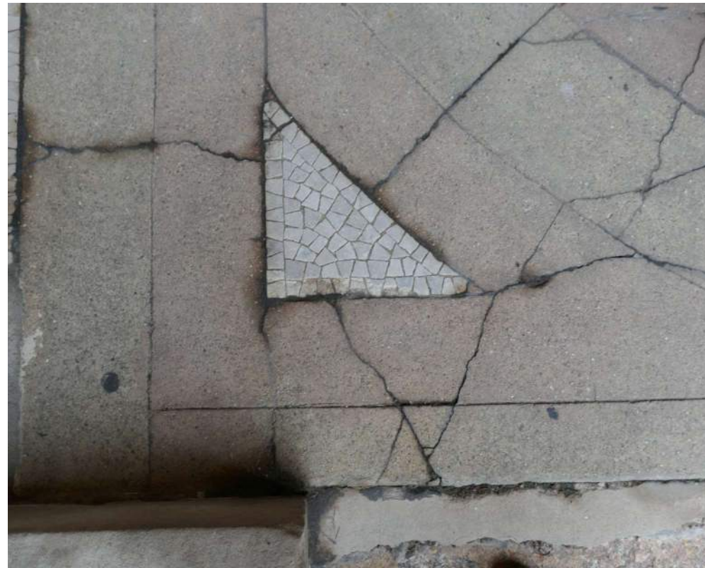
CENTER BAY MISSING STONE REPLACED WITH CEMENTITIOUS FILL
