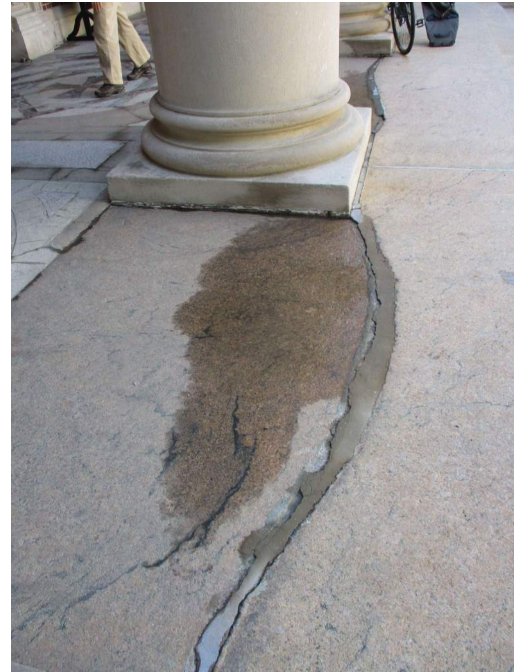
PARGED FILLET AT CHAPEL ENTRANCE STEPS
