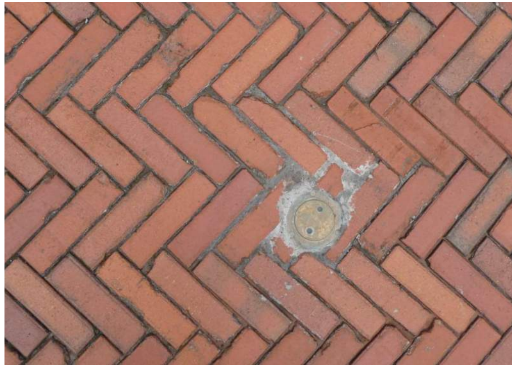
BRICK PAVERS - GROUTED METAL SOCKET
