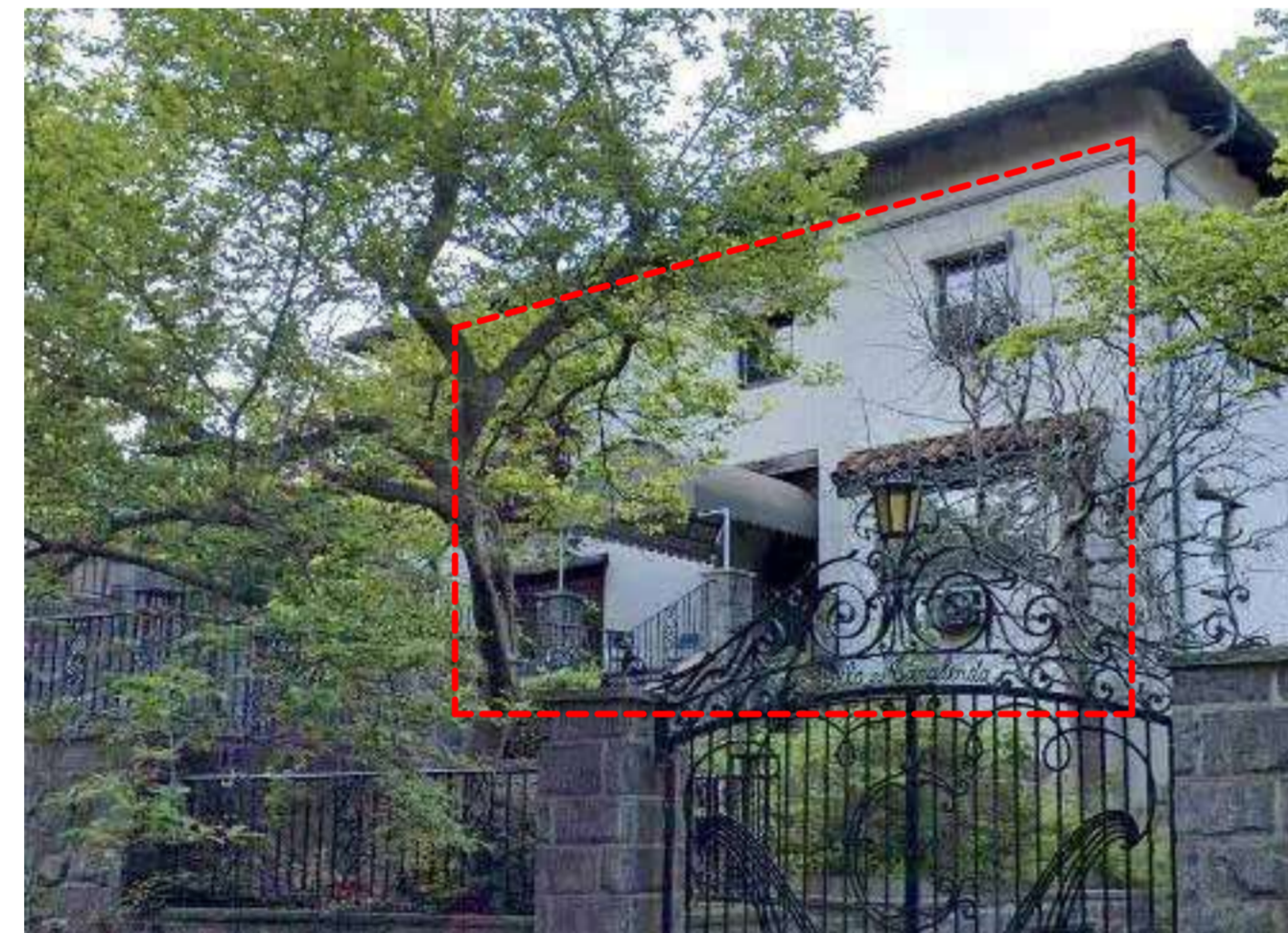
(2) ORIGINAL WINDOWS AND DOOR ON FRONT FACADE (SOUTH FACADE)
