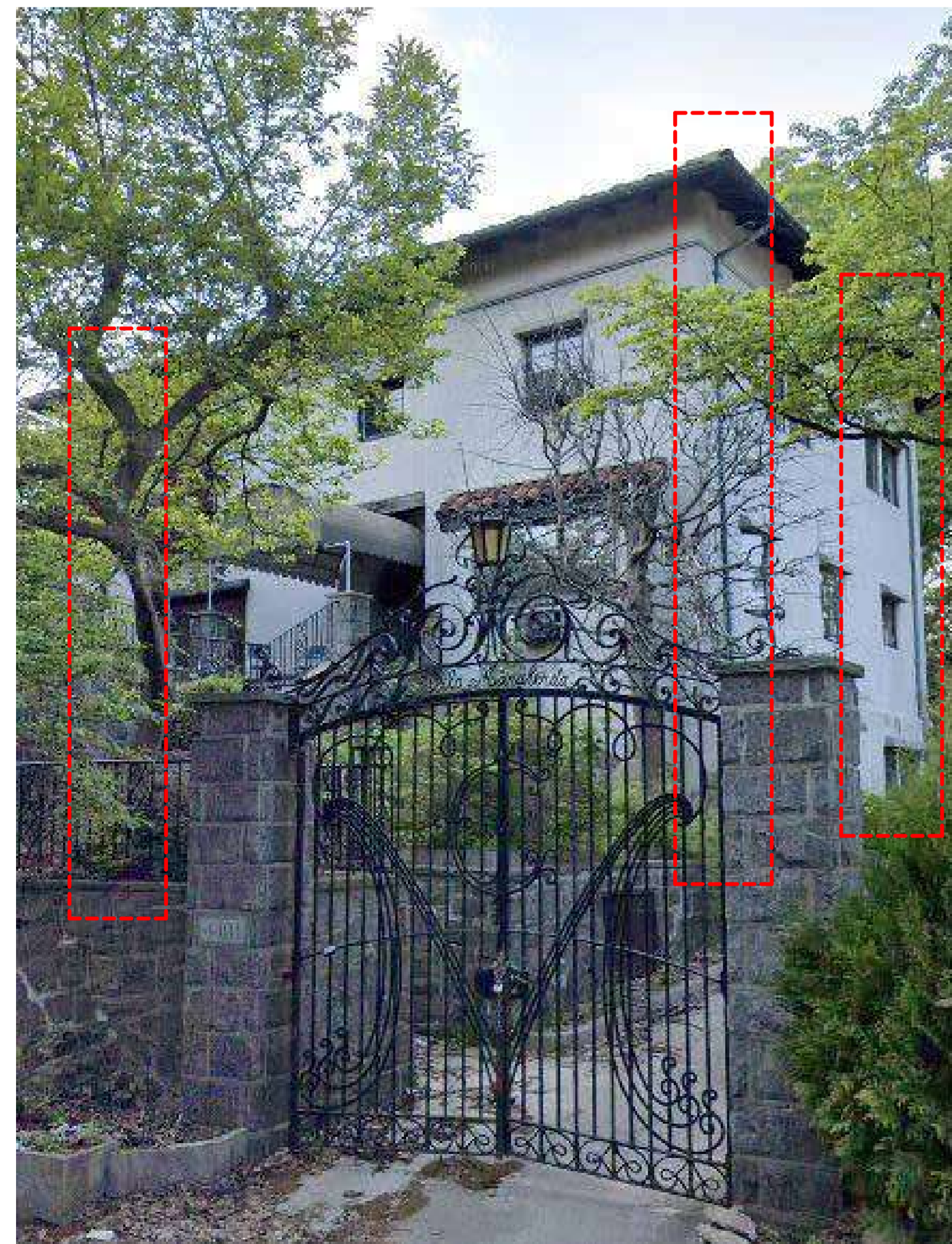
(1) ORIGINAL COPPER GUTTERS
