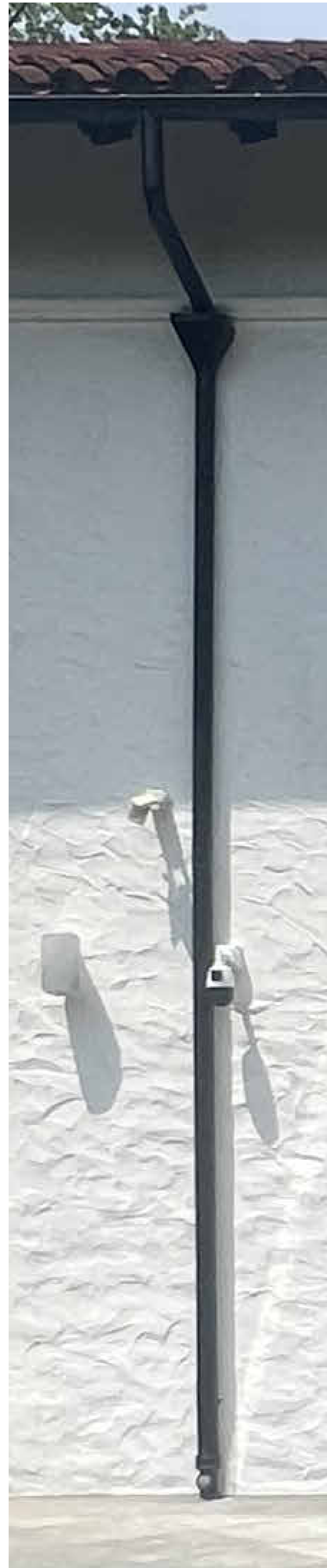
NEW GUTTERS AND DOWNPIPES IN ALUMINUM COL. BLACK
