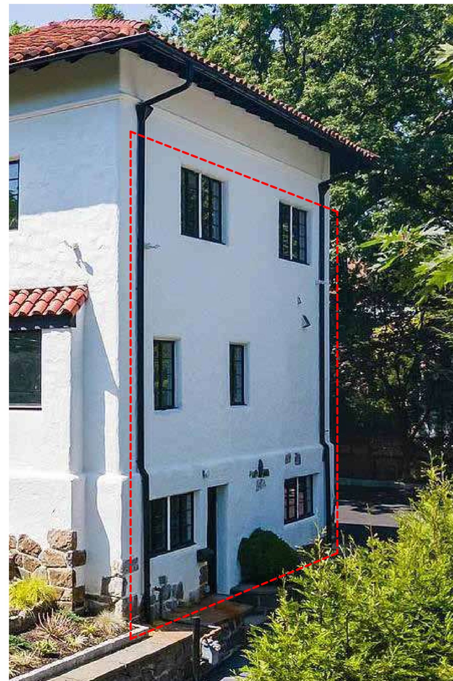
(1) EXISTING WINDOWS AND DOOR ON SIDE YARD (EAST FACADE)
