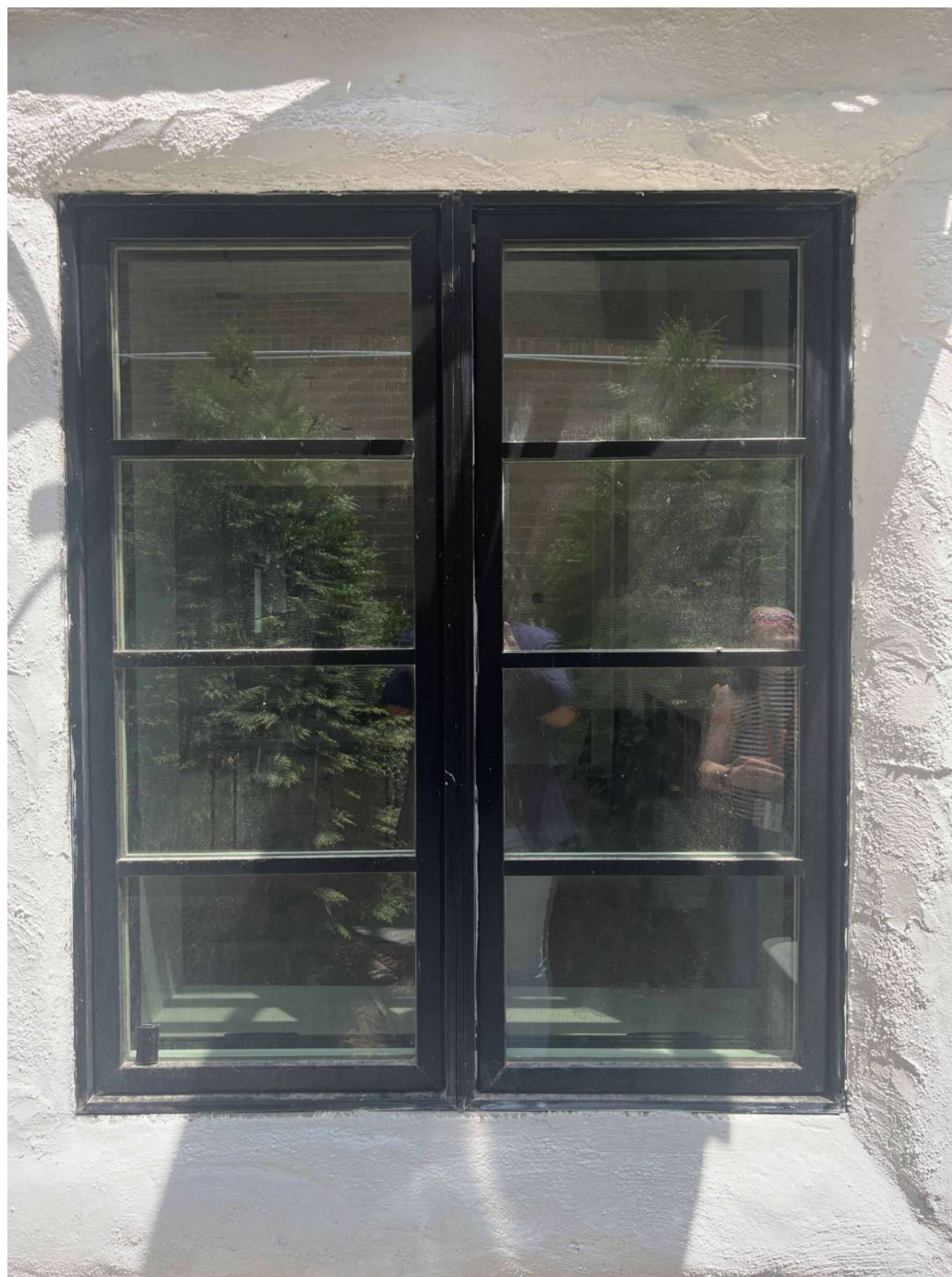
EXISTING ALUMINUM FRAME WINDOWS WITH GRILLES (COL. BLACK).
