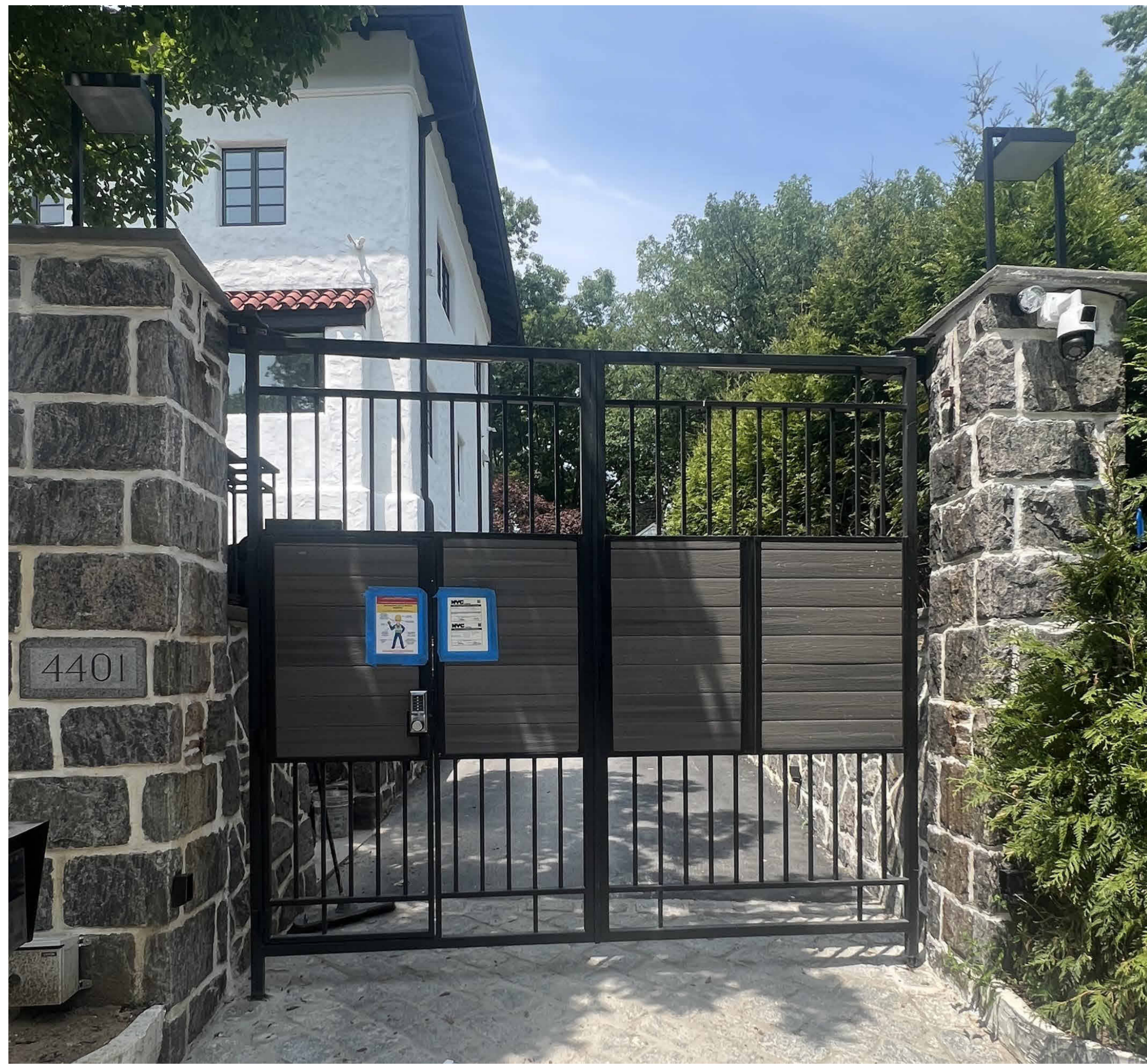
EXISTING MAIN GATE - FRONT AND REAR - STEEL (COL. BLACK), COMPOSITE PANELS, METAL LIGHT FIXTURES ON ORIGINAL STONE POSTS
