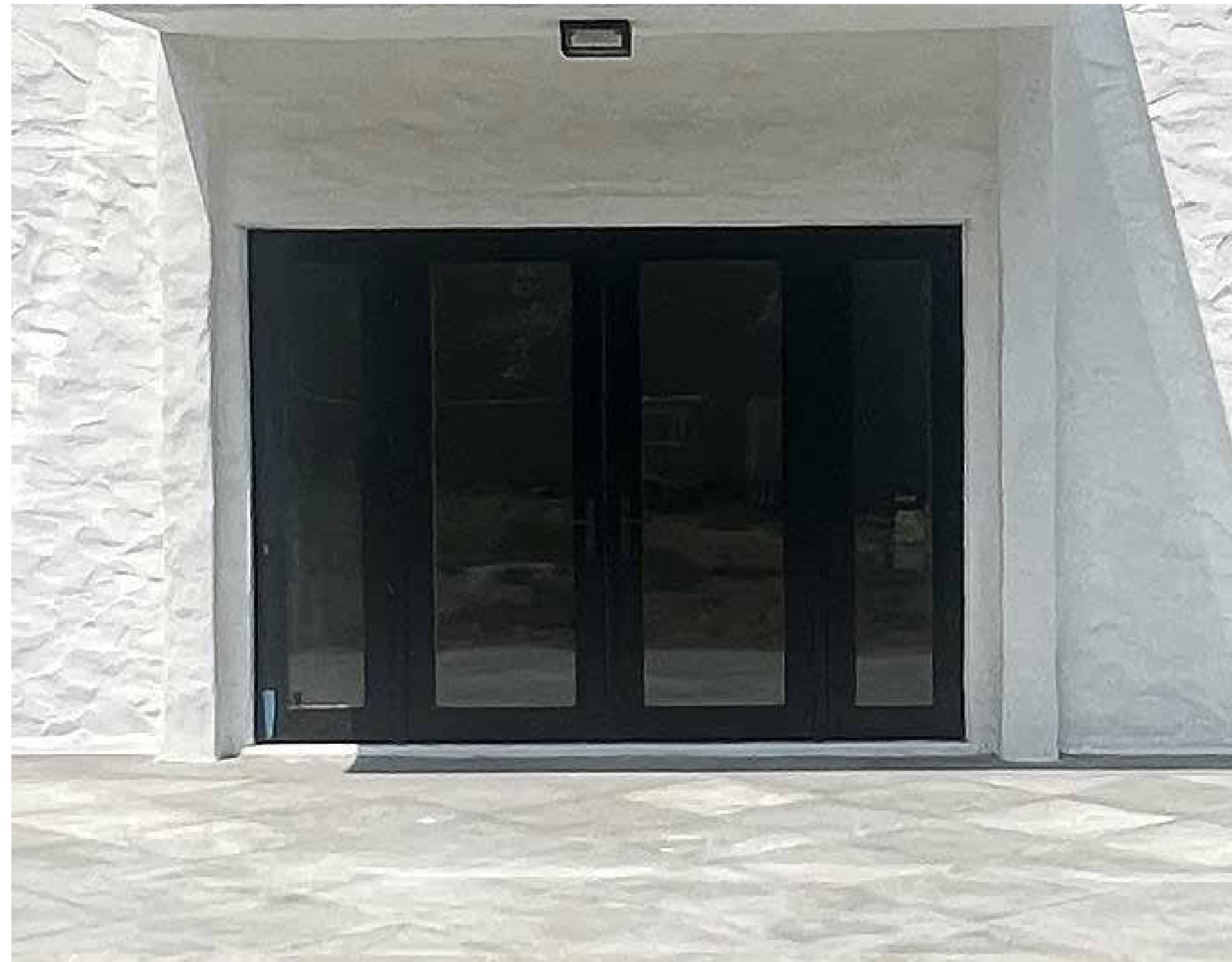
EXISTING ALUMINUM FRAME FOLDING DOOR WITH (COL. BLACK).
