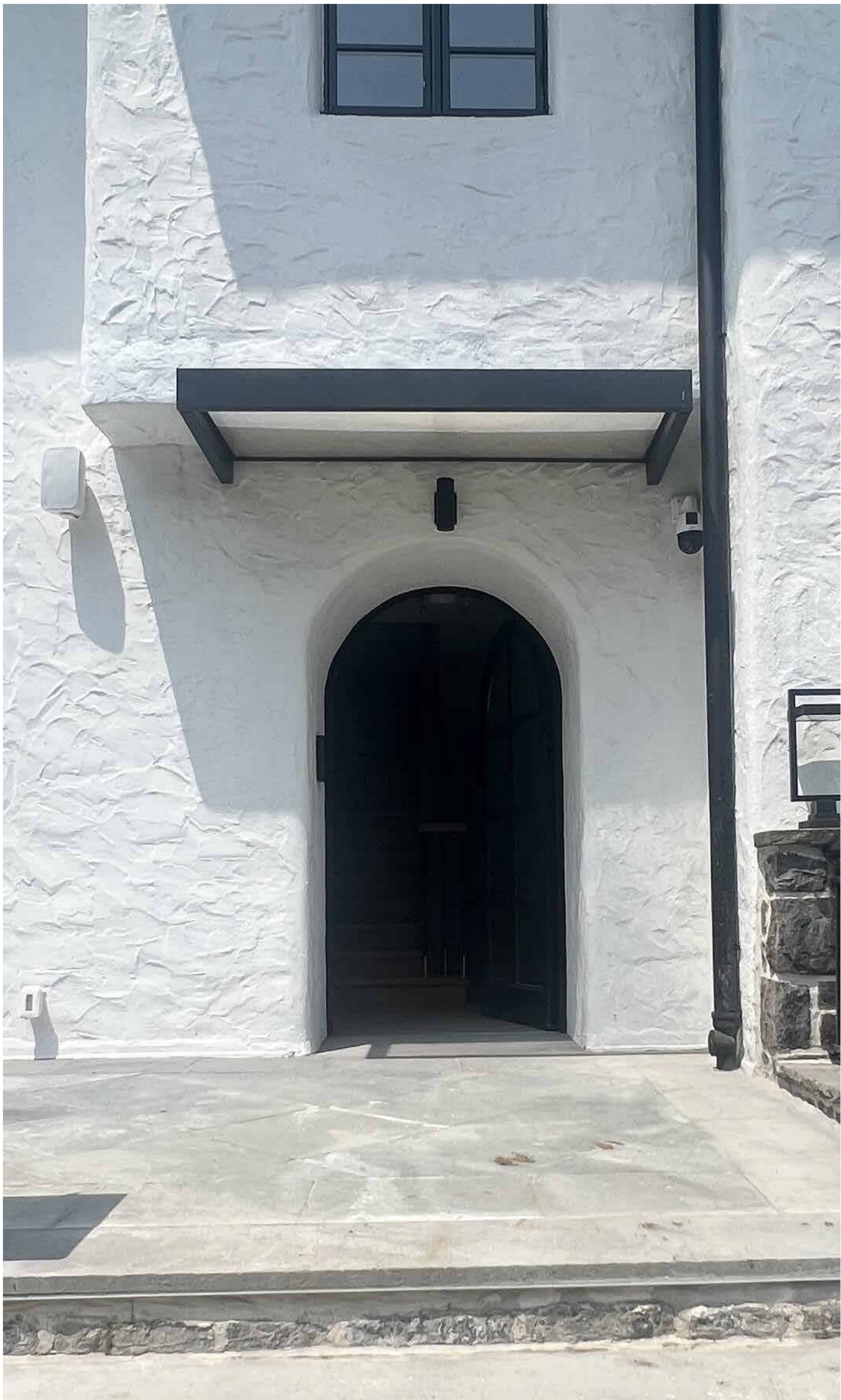
EXISTING MAIN ENTRY AWNING - STEEL PROFILE (COL. BLACK), GLASS PANEL.
