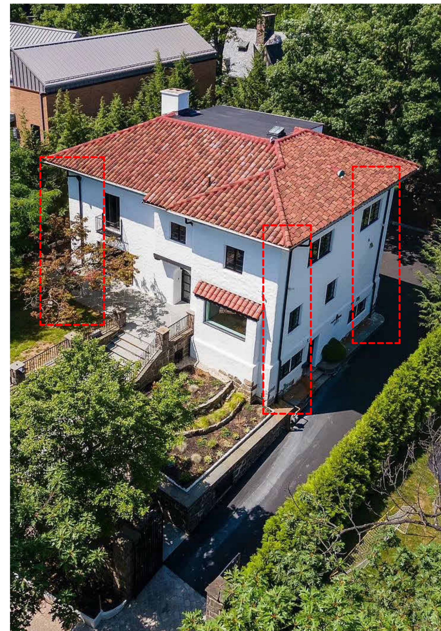
(1) EXISTING ALUMINUM GUTTERS
