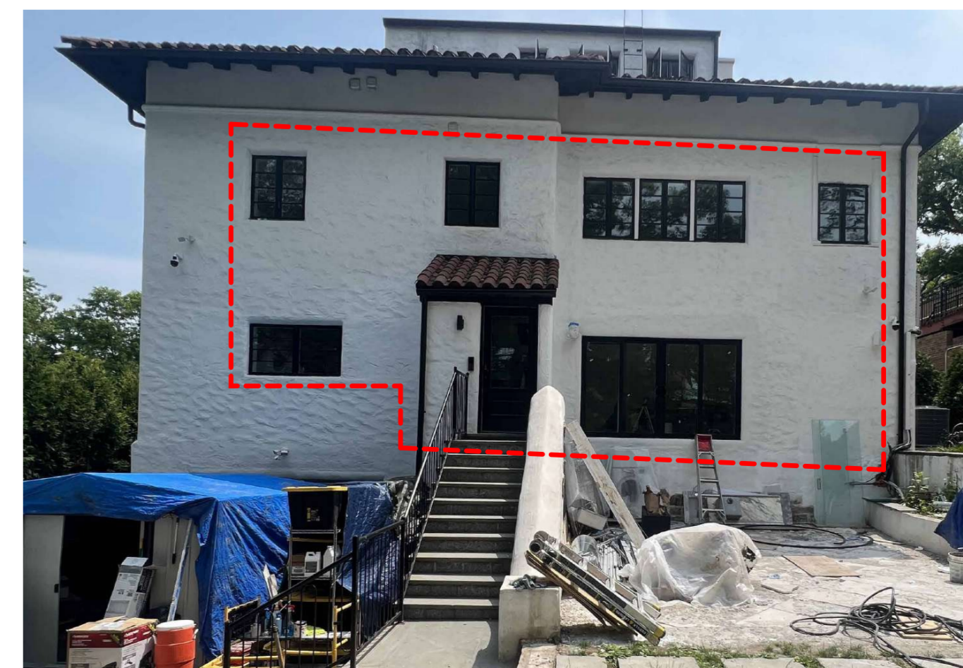
(3) EXISTING WINDOWS AND DOORS ON REAR FACADE (NORTH FACADE)
