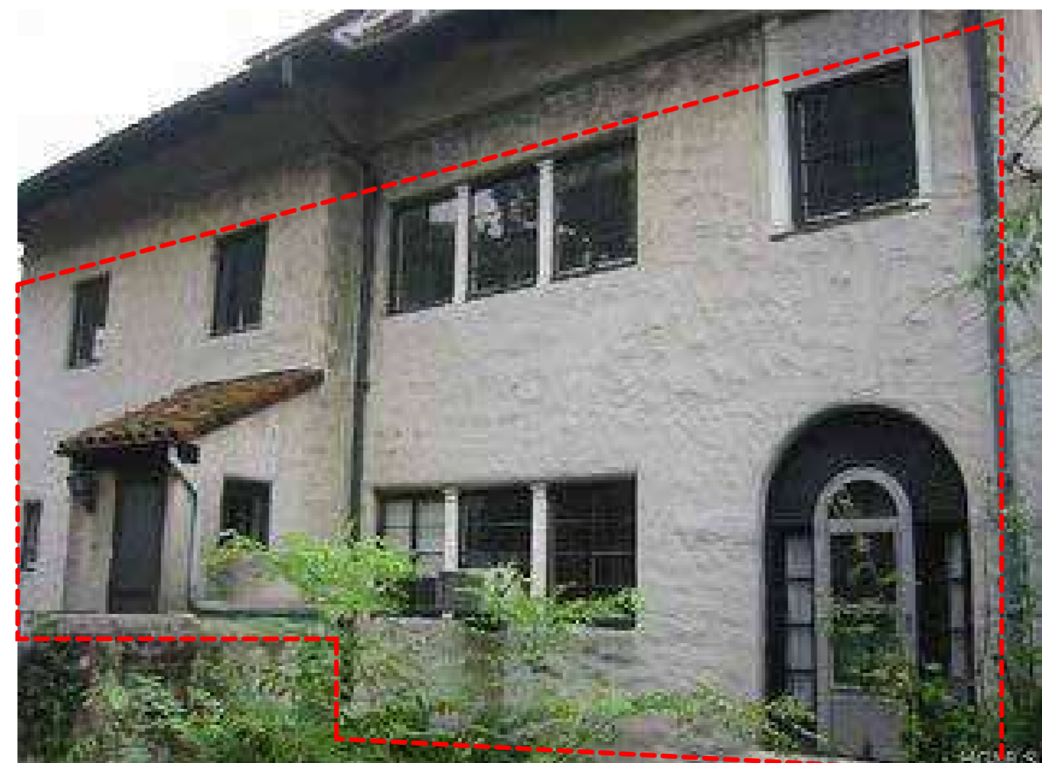
(3) ORIGINAL WINDOWS AND DOORS ON REAR FACADE (NORTH FACADE)
