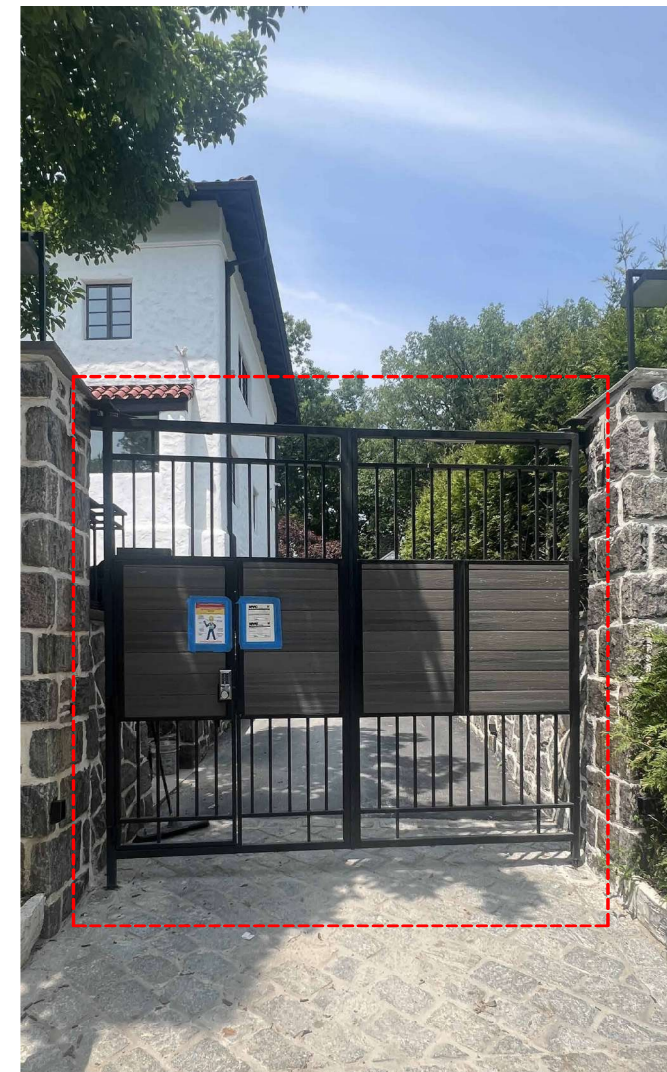
(1) EXISTING STEEL DRIVEWAY GATE
