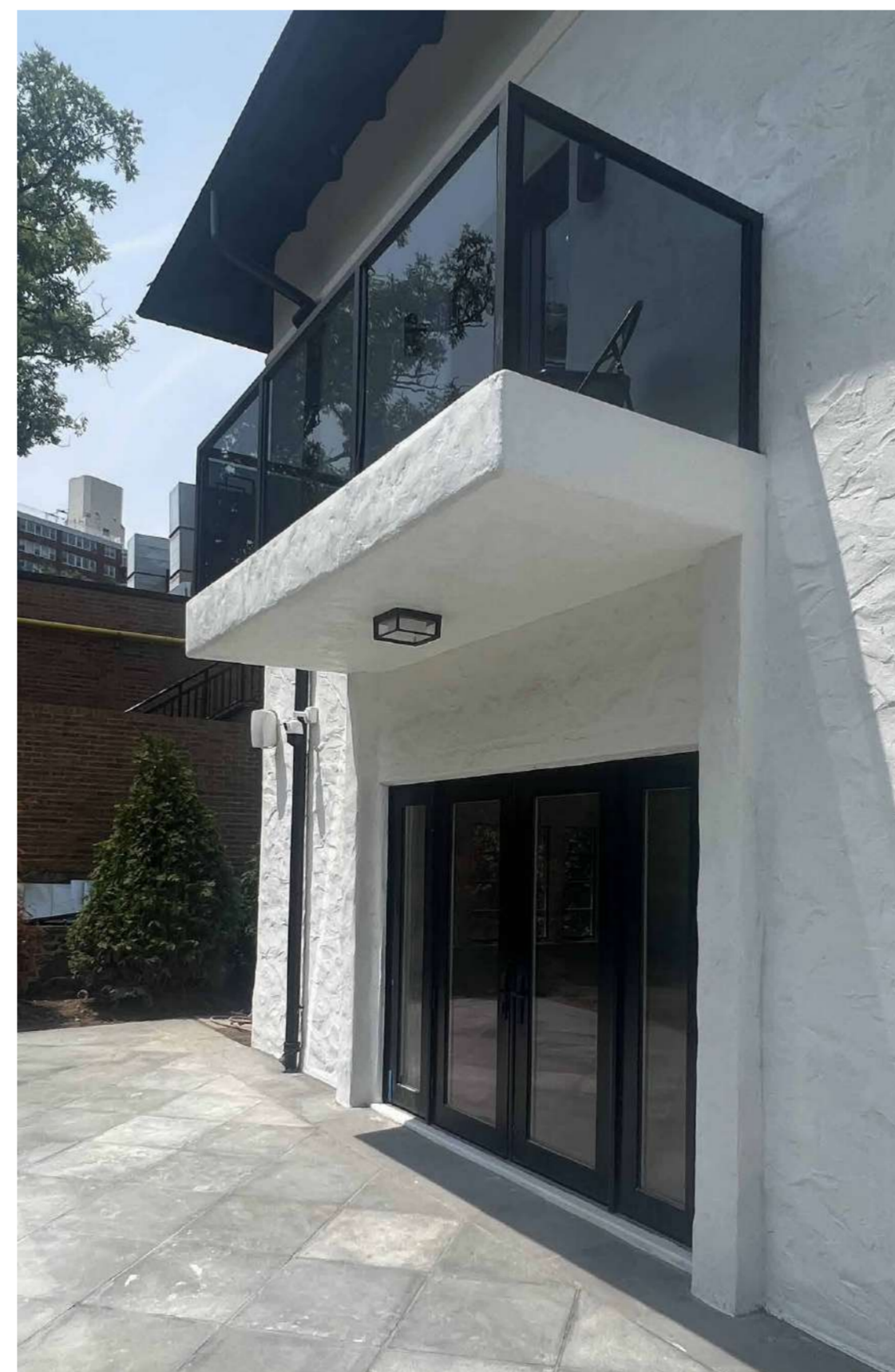
EXISTING BALCONY - STEEL PROFILES (COL. BLACK), GLASS PANELS (TINTED).
