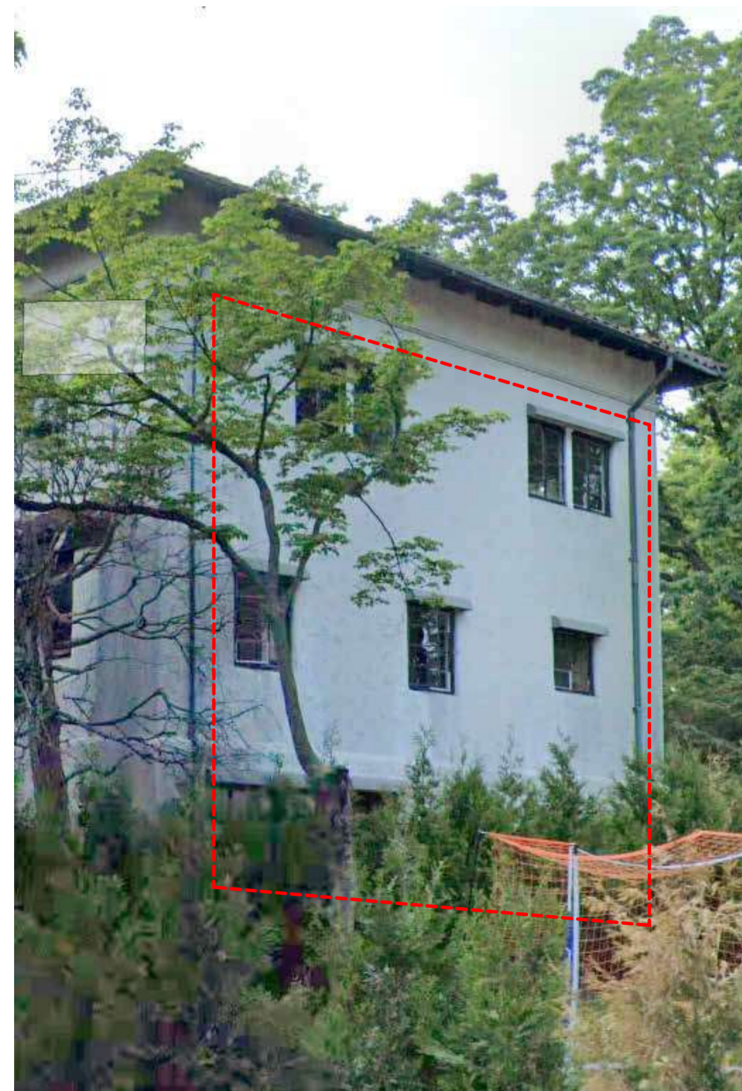
(1) ORIGINAL WINDOWS AND DOOR ON SIDE YARD (EAST FACADE)
