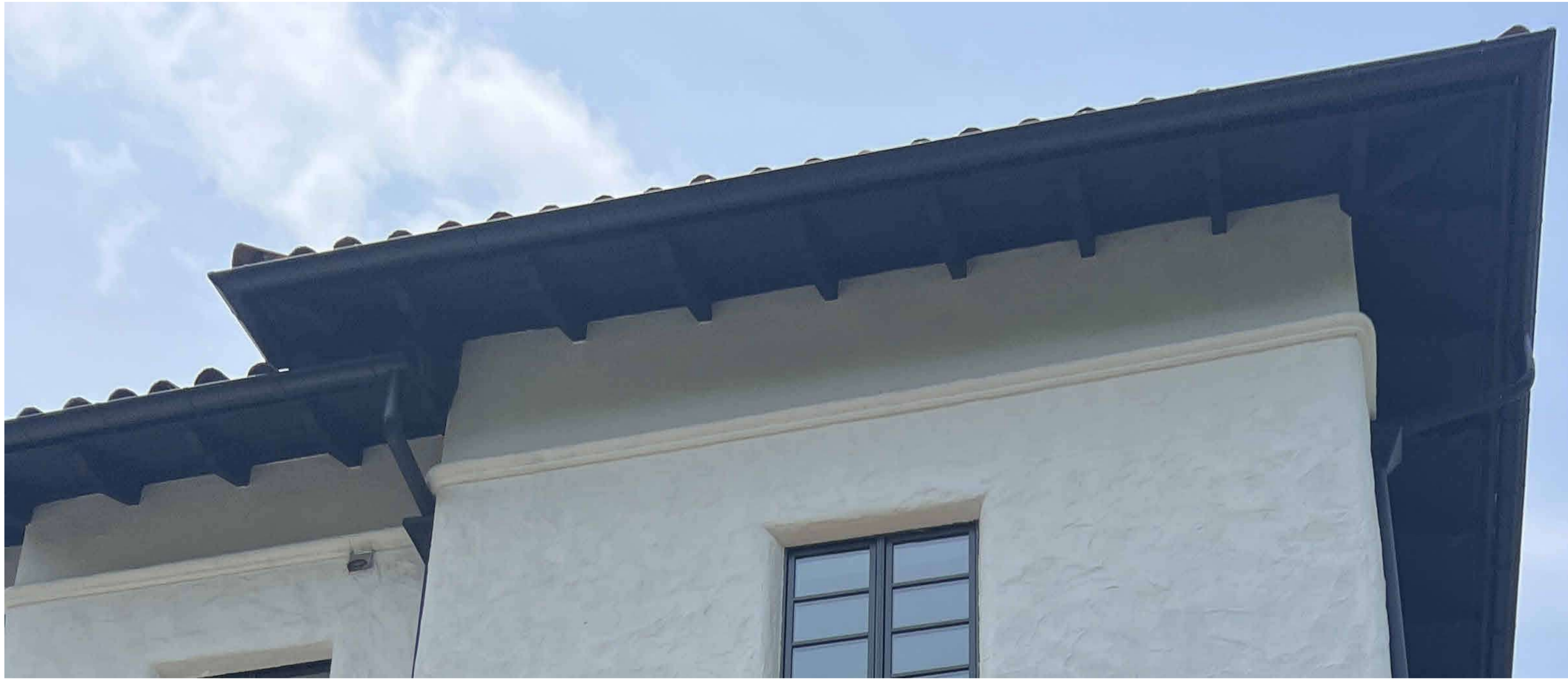
NEW GUTTERS AND DOWNPIPES IN ALUMINUM COL. BLACK
