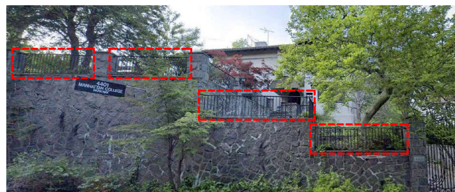
(3) REPLACEMENT OF ORIGINAL AREAWAY IRONWORK
