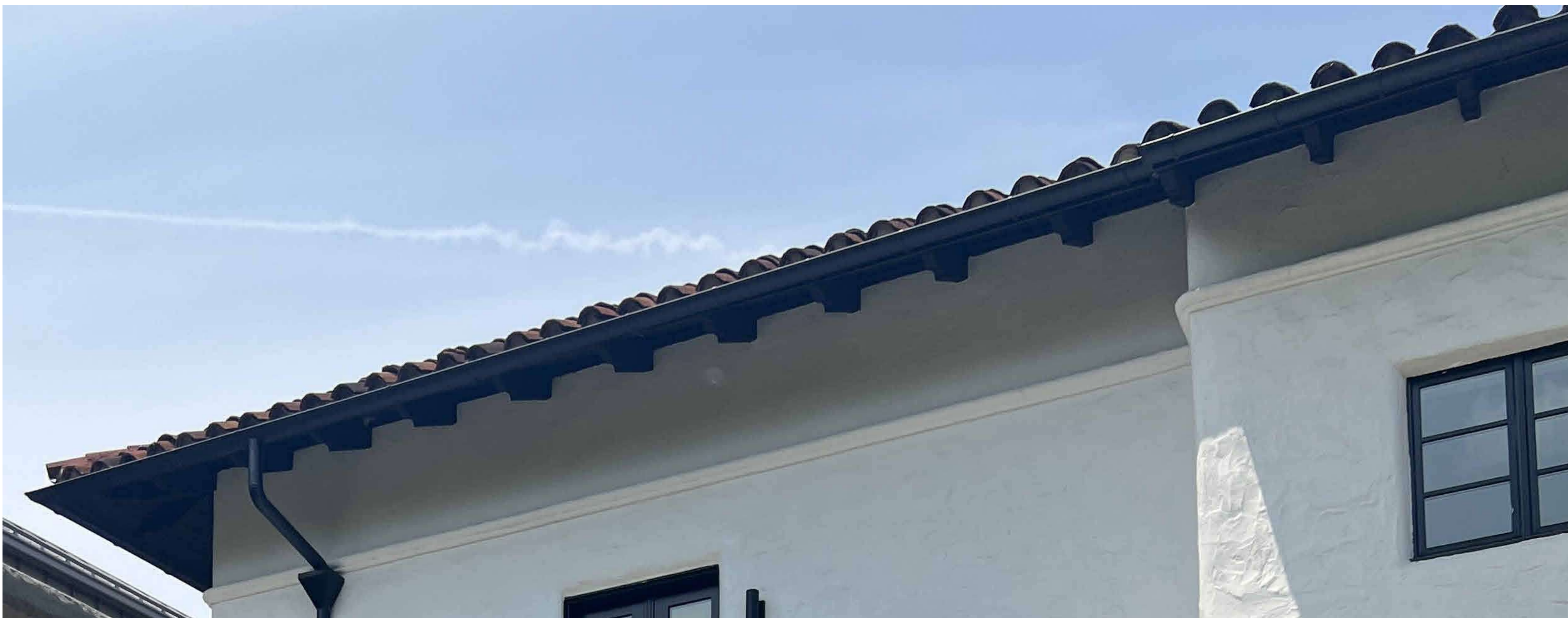
NEW GUTTERS AND DOWNPIPES IN ALUMINUM COL. BLACK
