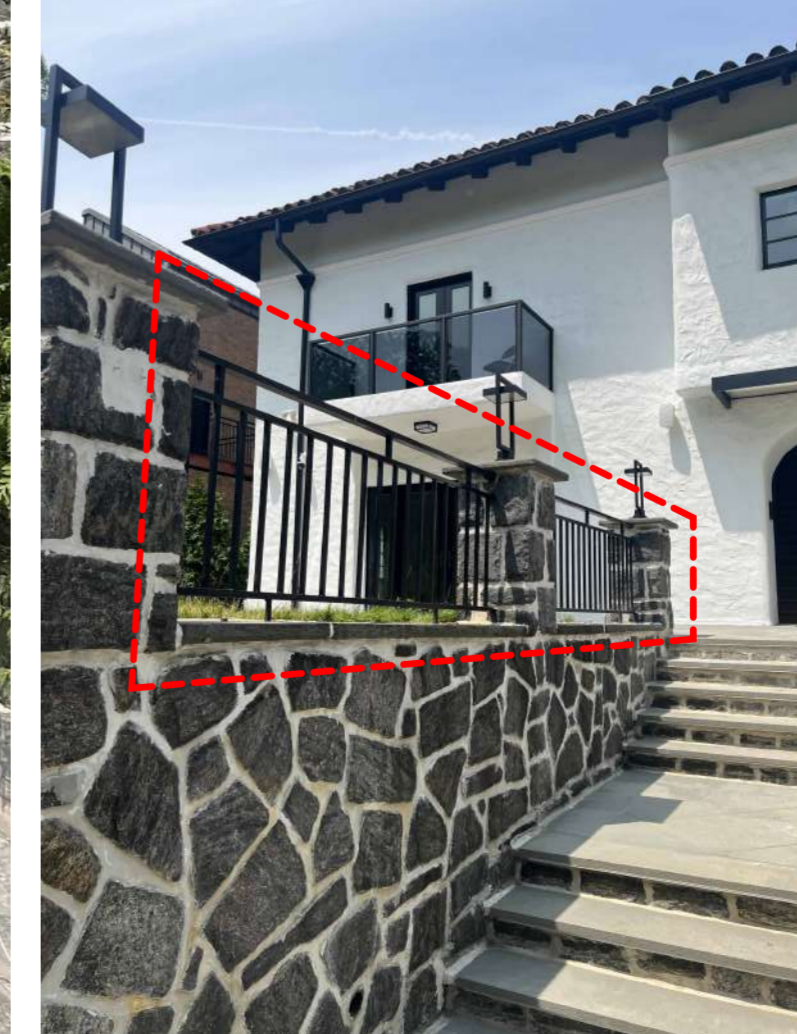
(4) EXISTING STEEL RAILING
