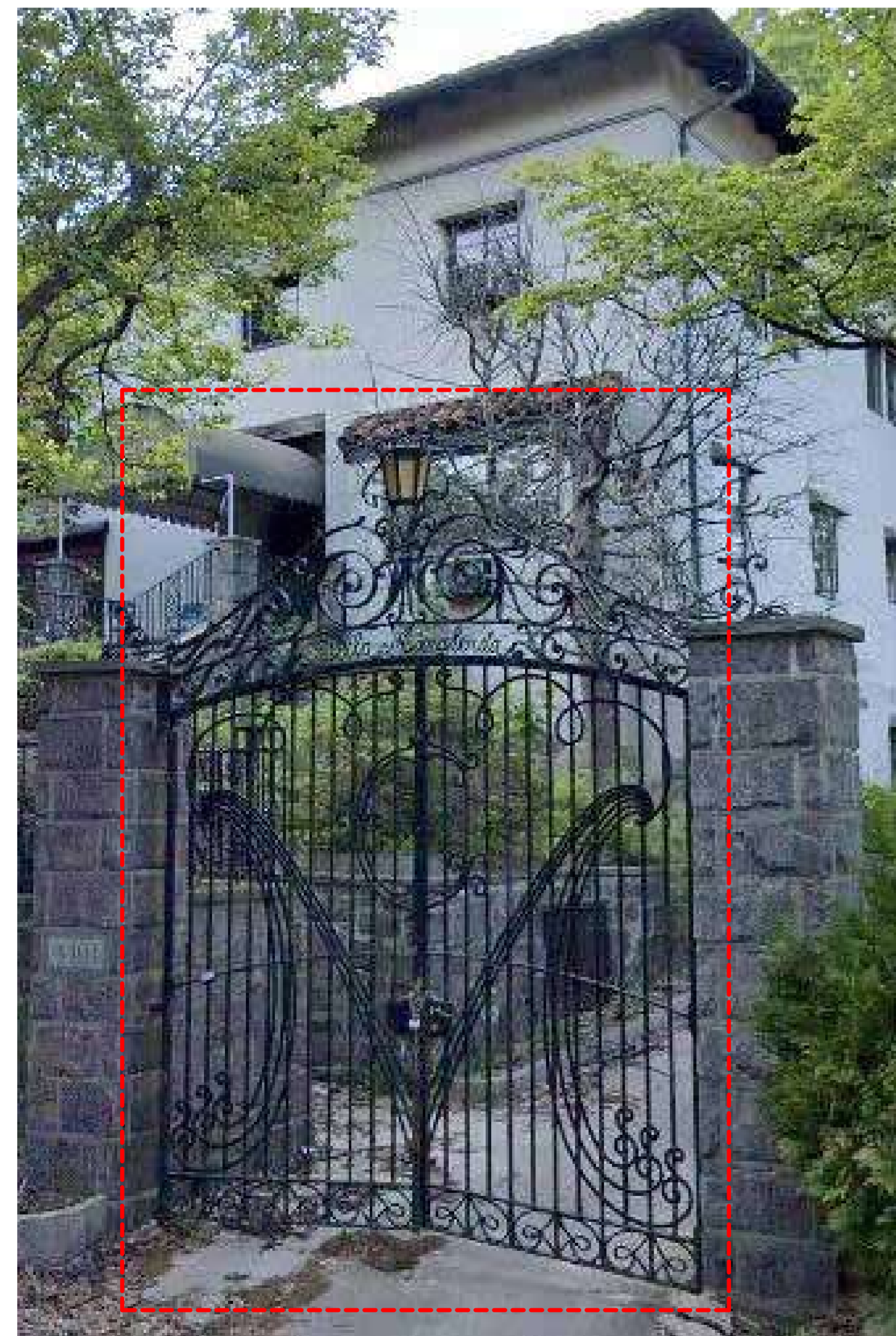
(1) ORIGINAL WROUGHT-IRON GATE
