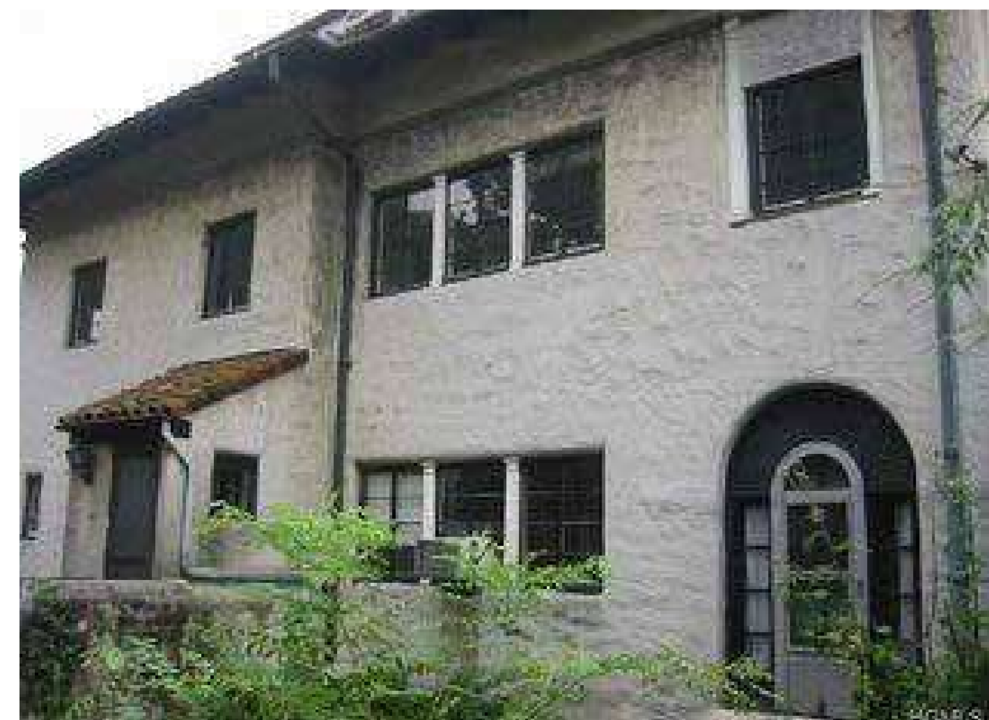
(2) ORIGINAL REAR FACADE (NORTH FACADE)
