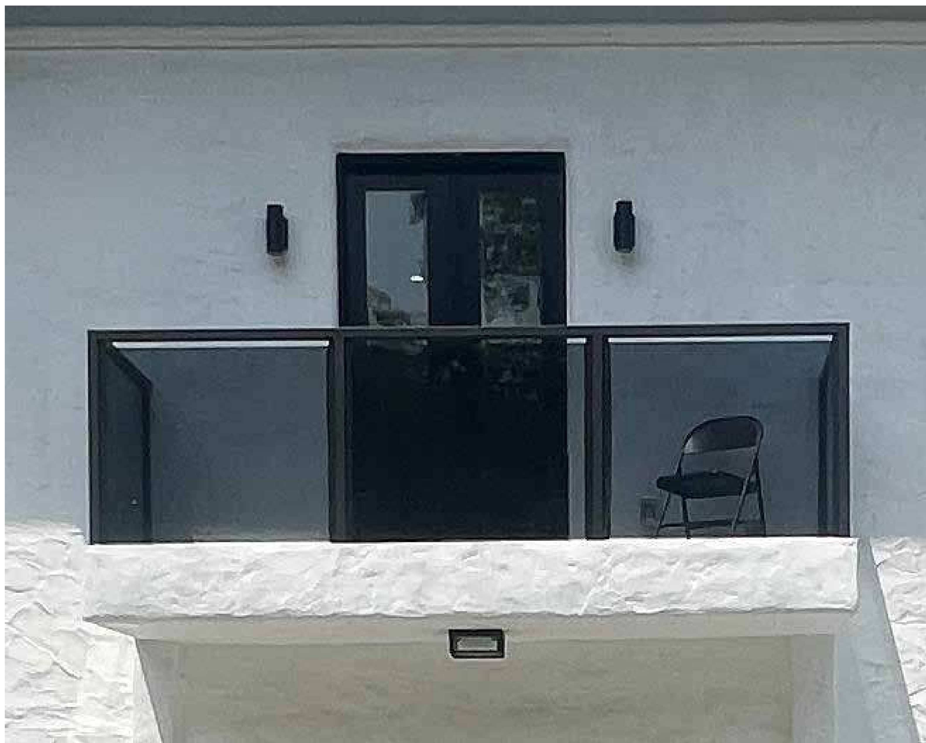
EXISTING BALCONY - STEEL PROFILES (COL. BLACK), GLASS PANELS (TINTED).
