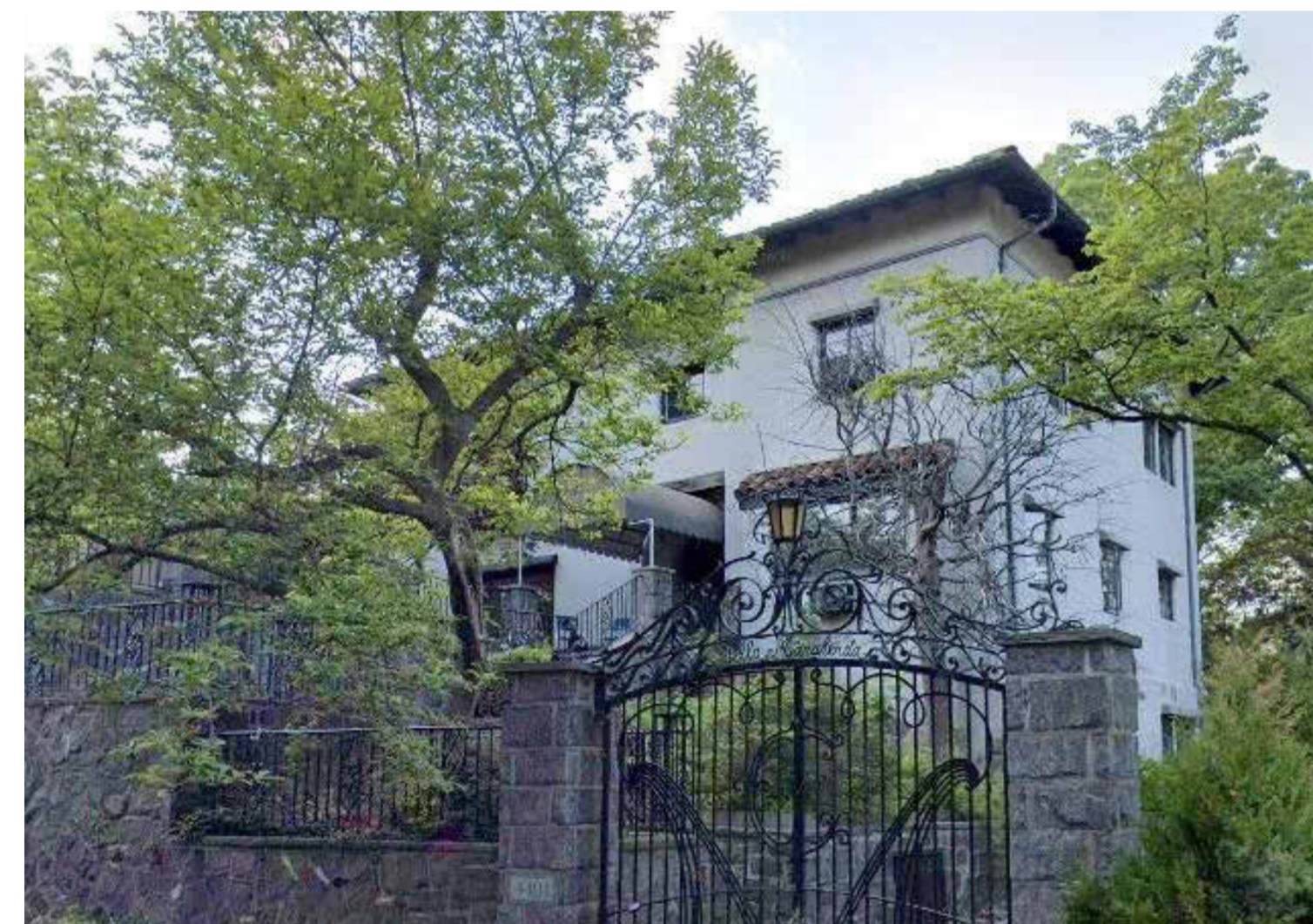
(1) ORIGINAL FRONT FACADE (SOUTH FACADE)
