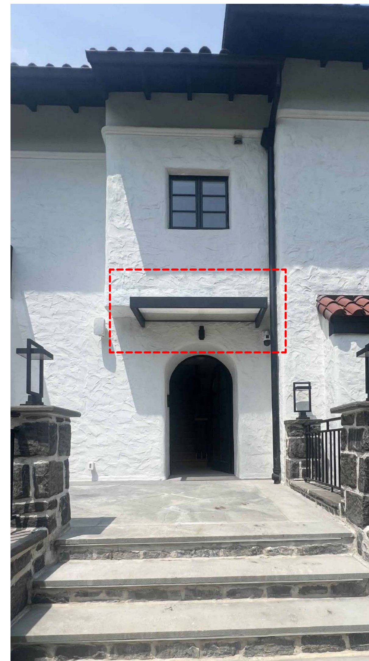
(1) EXISTING MAIN ENTRANCE STEEL FRAME CANOPY
