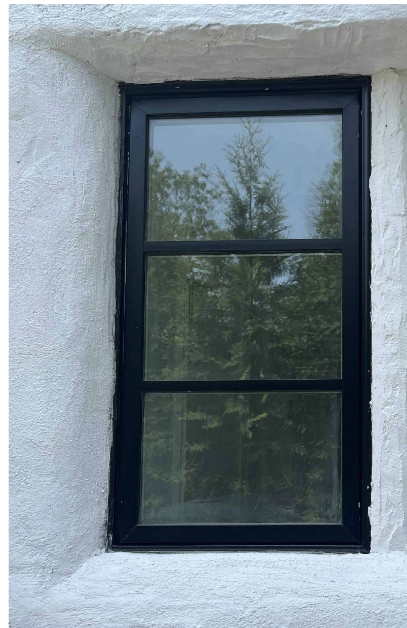
EXISTING ALUMINUM FRAME WINDOWS WITH GRILLES (COL. BLACK).
