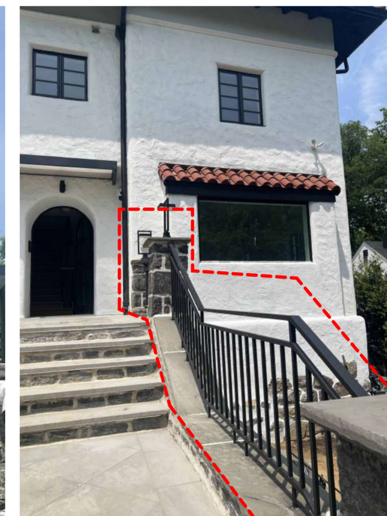
(2) EXISTING STEEL RAILING
