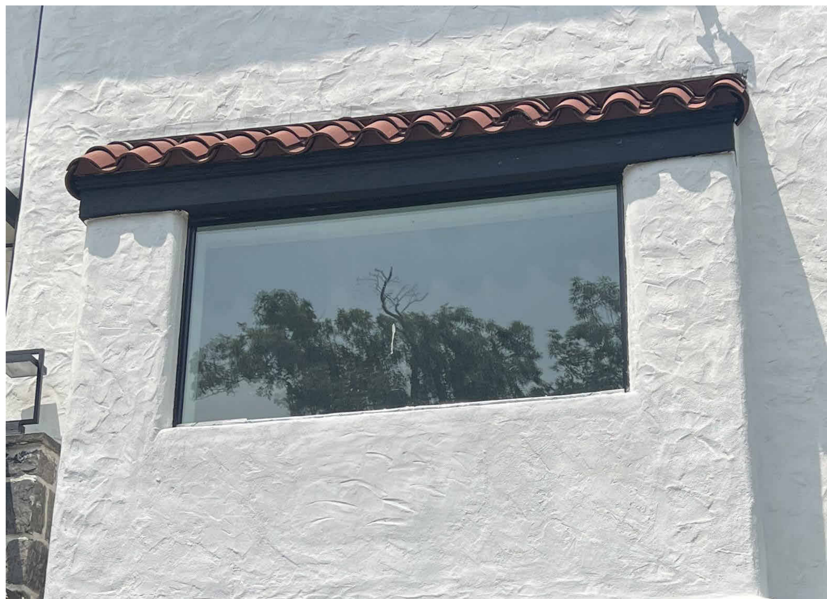
EXISTING FIXED ALUMINUM FRAME WINDOW (COL. BLACK).
