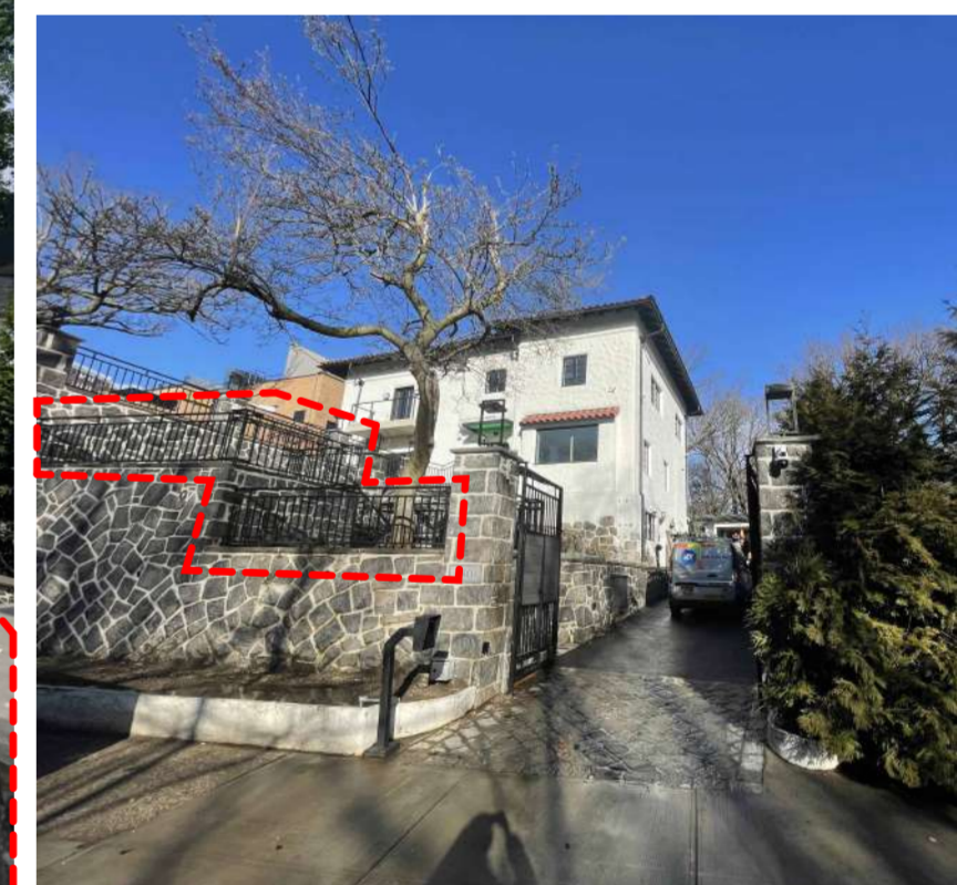
(3) EXISTING STEEL RAILING
