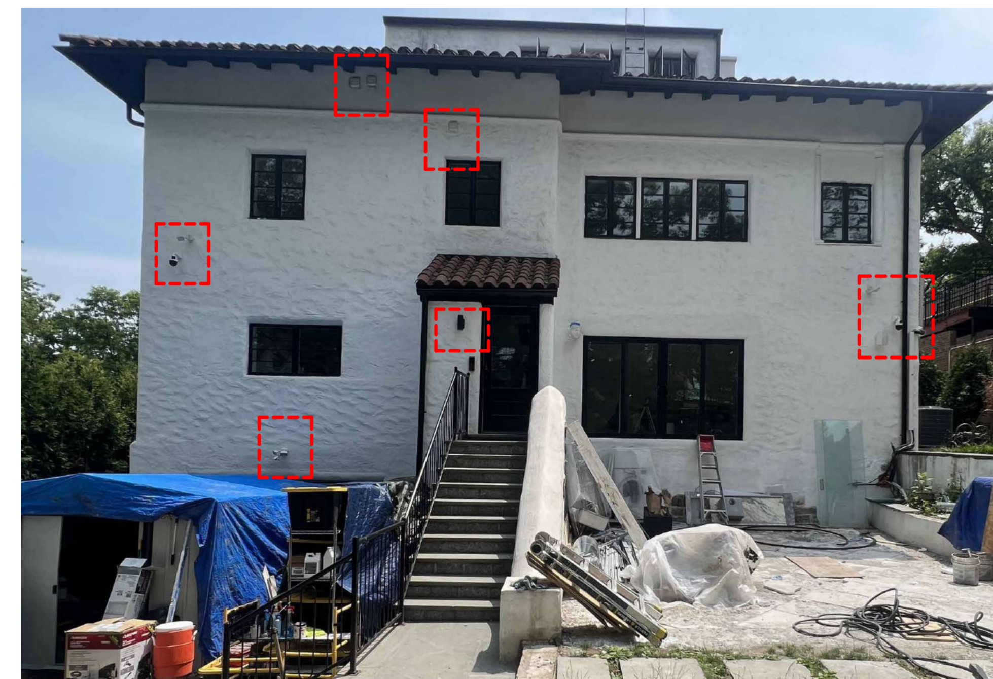
(2) EXISTING REAR FACADE W/ NEW CAMERAS AND LIGHTING FIXTURES
