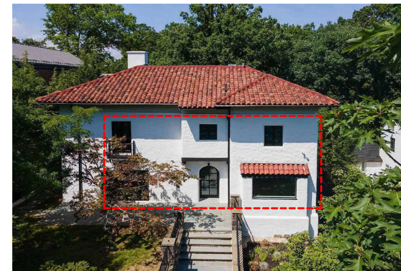
(2) EXISTING WINDOWS AND DOOR ON FRONT FACADE (SOUTH FACADE)
