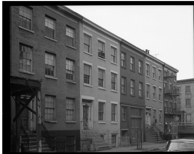
58-66 HORATIO STREET HORATIO STREET SIDE
