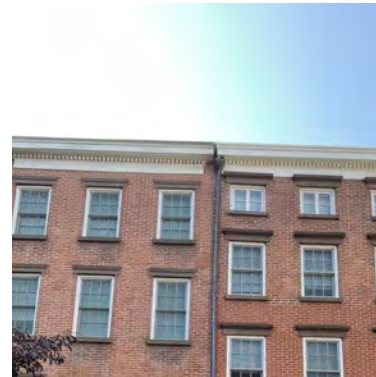
BUILT MOCK UP
