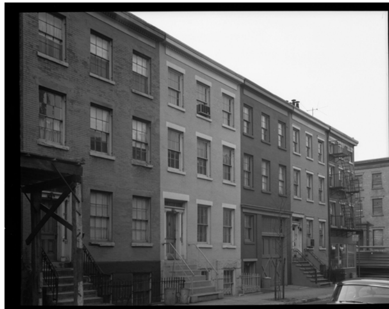
58-66 HORATIO STREET HORATIO STREET SIDE
