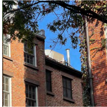
EXISTING (CLOSE UP)
