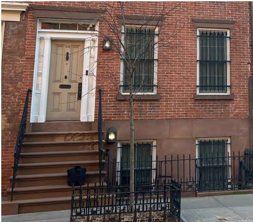
EXISTING FRONT FACADE
