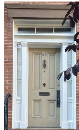
EXISTING FRONT DOOR
