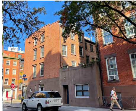
EXISTING STREET VIEW
