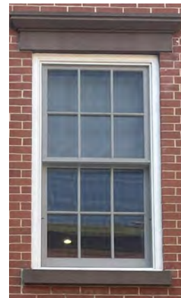
EXISTING FRONT WINDOWS
