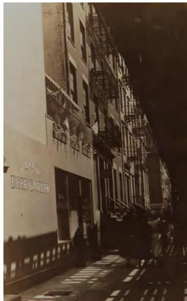
66 HORATIO STREET GREENWICH STREET SIDE
