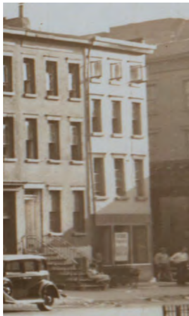
64 & 66 HORATIO STREET HORATIO STREET SIDE
