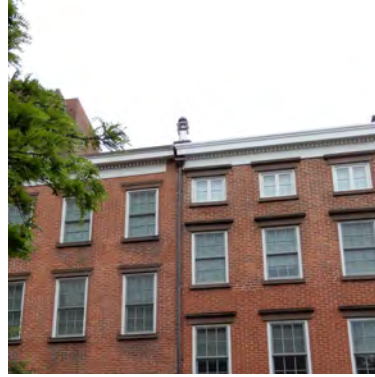
EXISTING (CLOSE UP)
