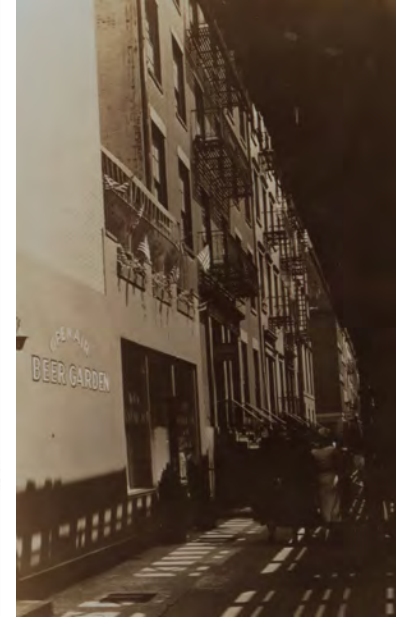
66 HORATIO STREET GREENWICH STREET SIDE
