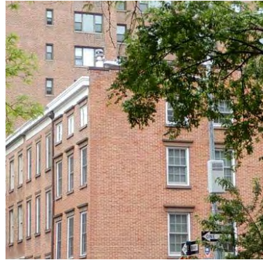
EXISTING (CLOSE UP)
