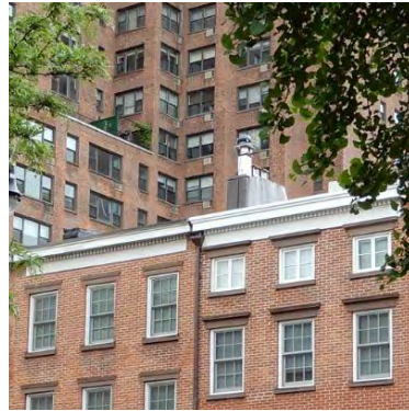
EXISTING (CLOSE UP)
