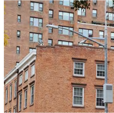
BUILT MOCK UP
