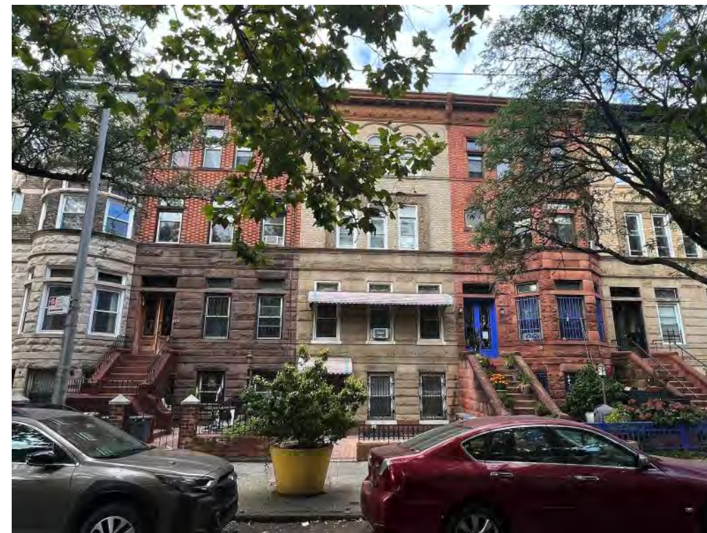
Attached 3-Story Row Houses:
