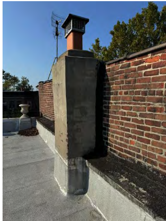
Existing Chimney to Remain ( Active )
