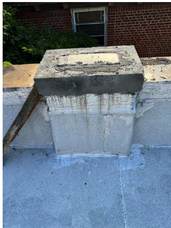
Existing Capped Chimney to Remain ( Not Active )
