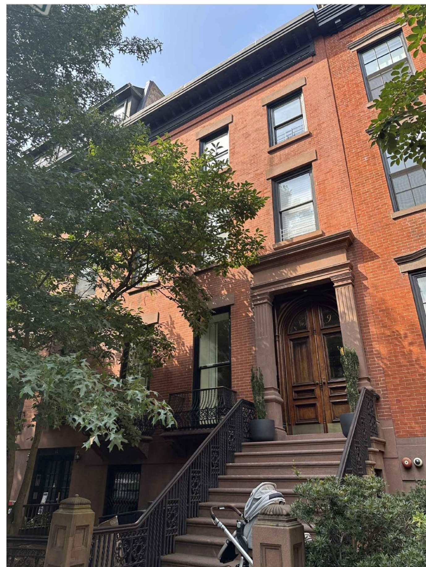
9 MONROE PL - GREEK REVIVAL 1845 2006 permit to replace (6) 1 over 1 with (6) 1 over 1
