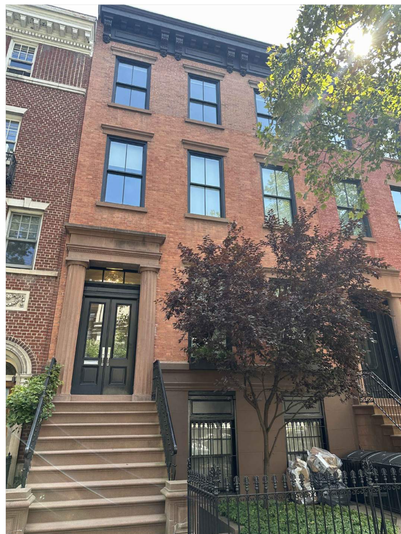
44 MONROE PL - GREEK REVIVAL 1837 2015 permit to replace (8) 12 over 1 with (8) 2 over 2
