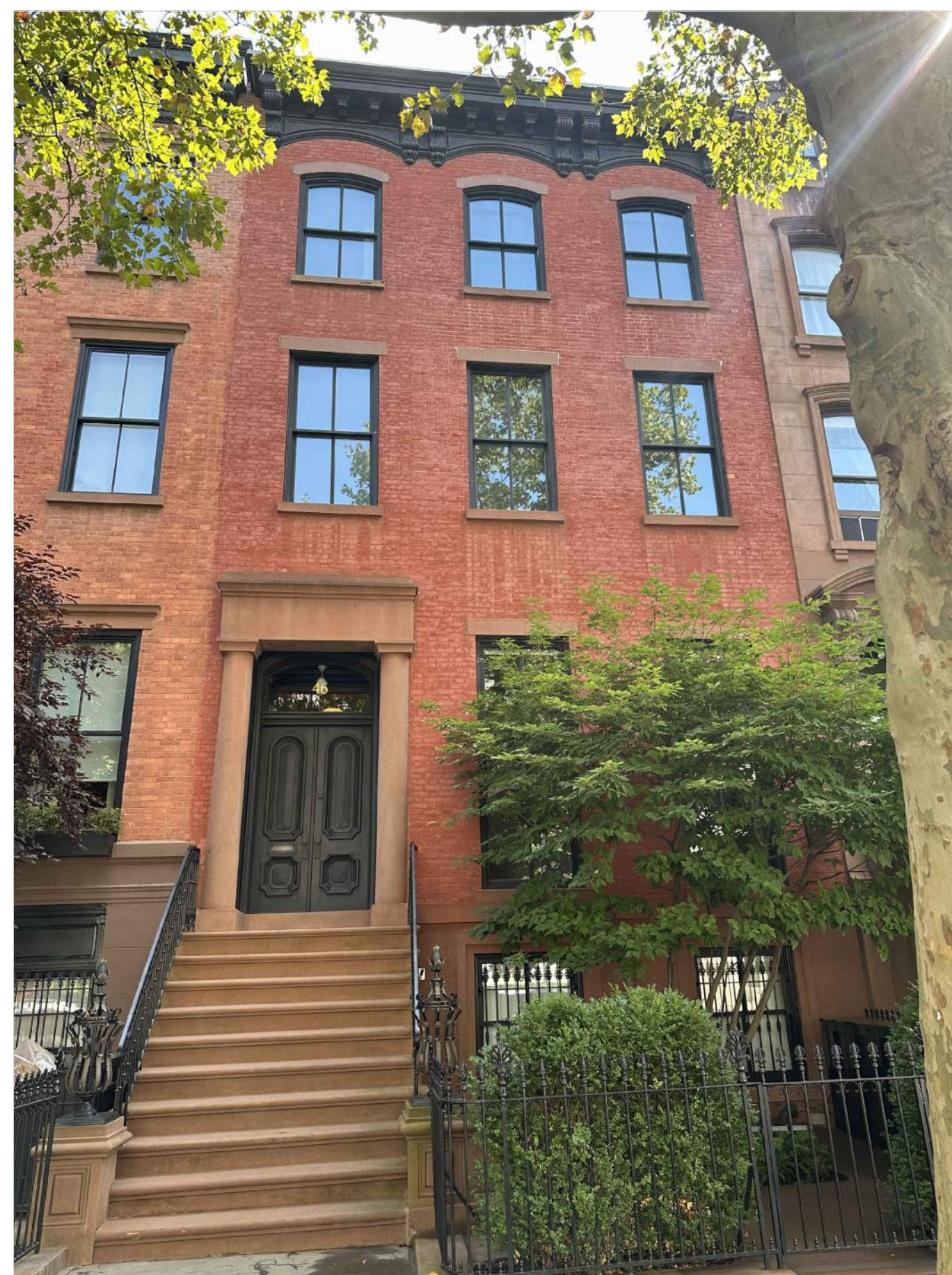
46 MONROE PL - GREEK REVIVAL 1835 2006 permit to replace (10) 1 over 1 with (10) 2 over 2
