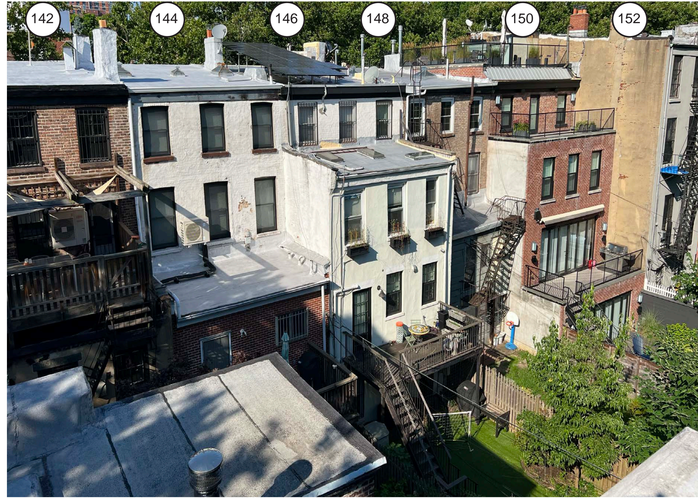
(B) NEIGHBORING REAR FACADES WITH HORIZONTAL EXTENSIONS - LOOKING EAST
