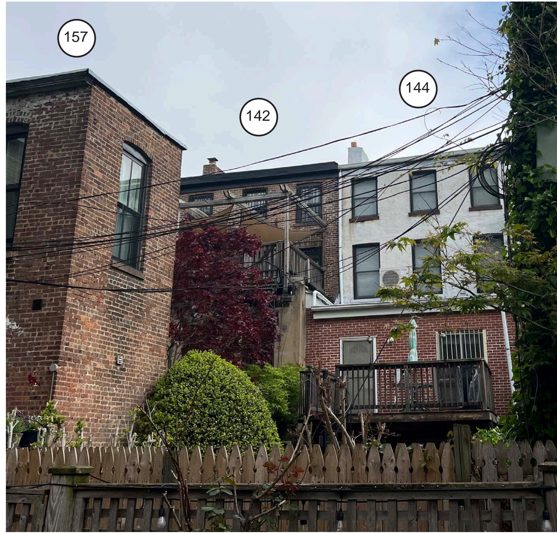
(A) EXISTING NEIGHBORING ADDITION - LOOKING NORTH
