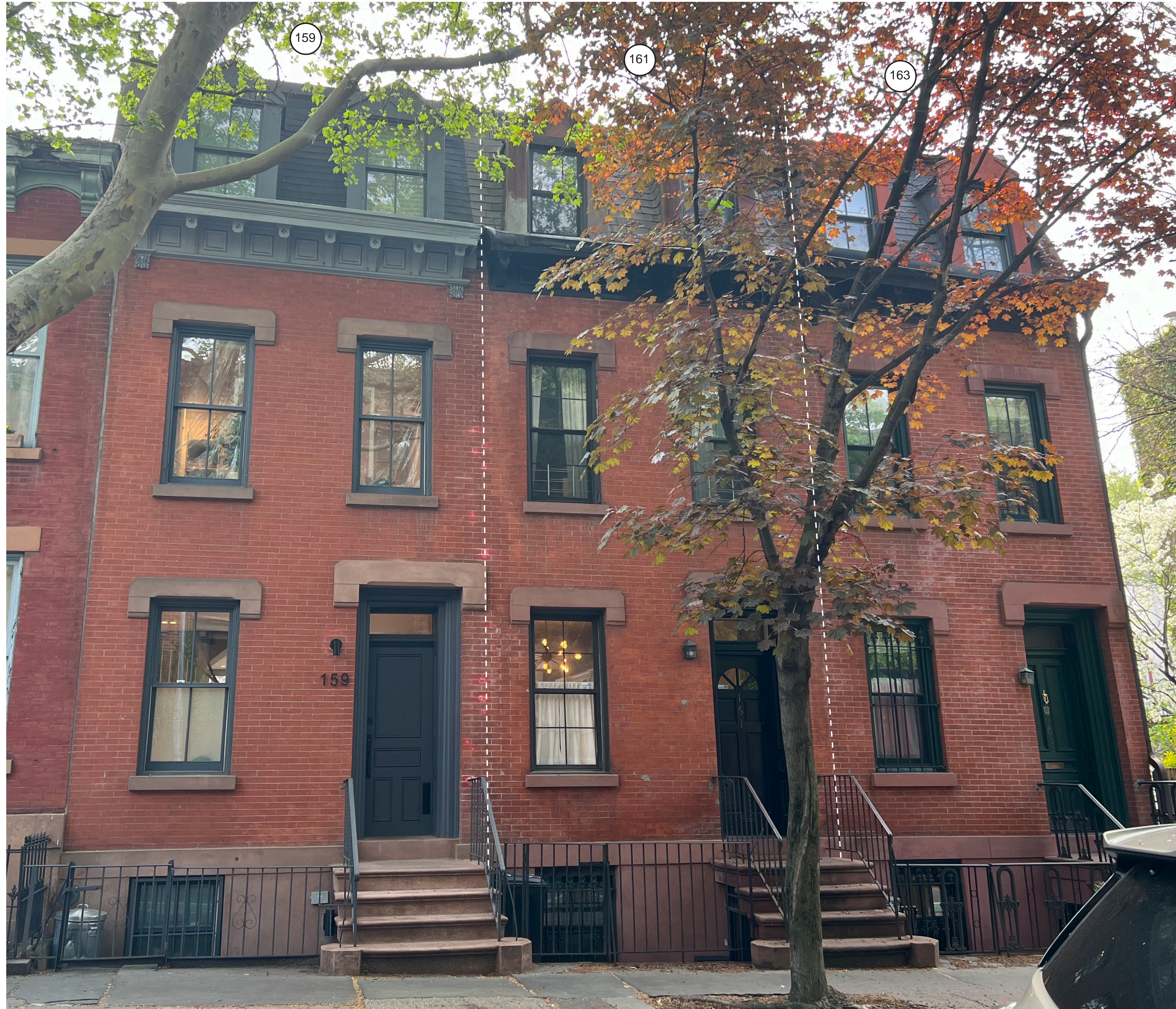
EXISTING FRONT FACADE - LOOKING EAST
