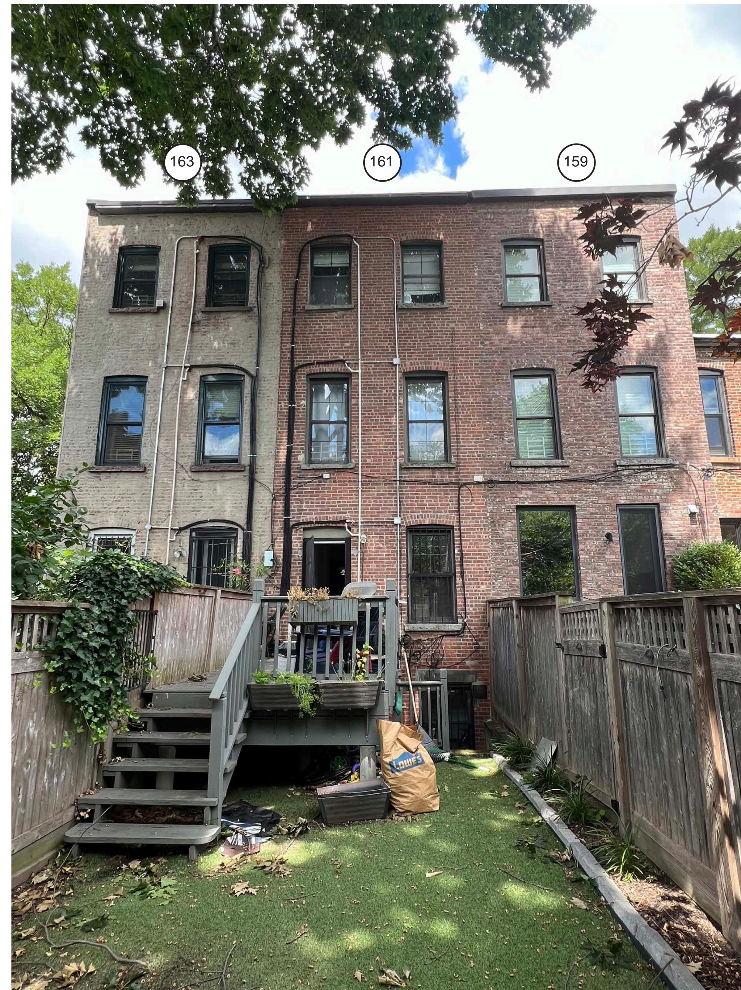
EXISTING REAR FACADE
