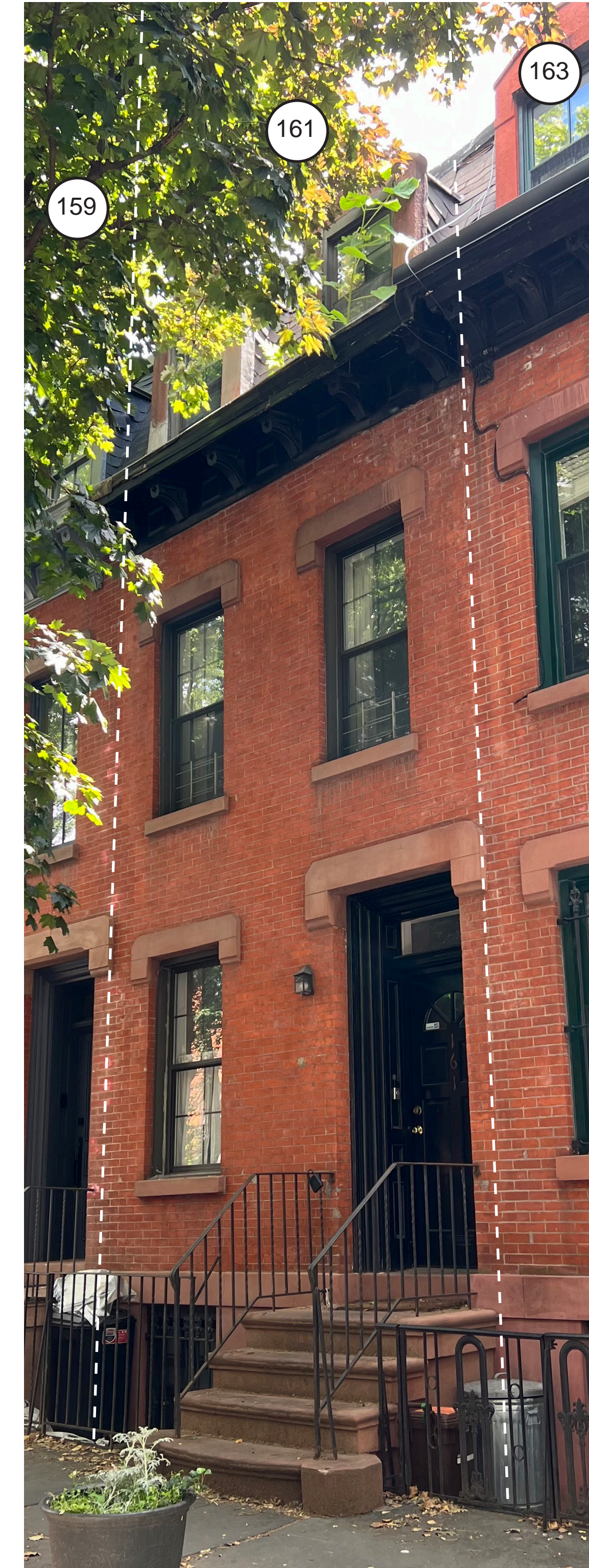
EXISTING FRONT FACADE - LOOKING EAST
