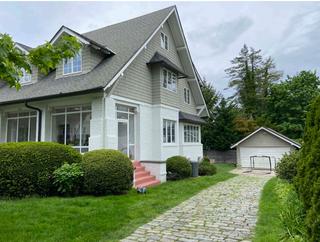
EXISTING CONDITIONS, LOOKING NW FROM PARK LANE
