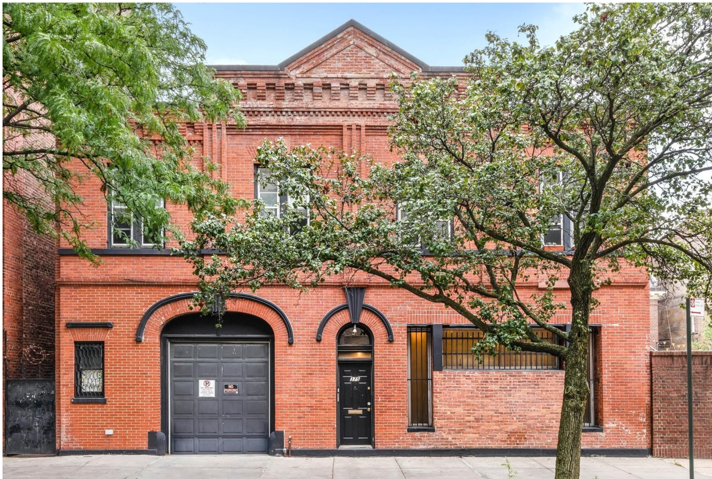
375 Vanderbilt Avenue - Existing Condition
