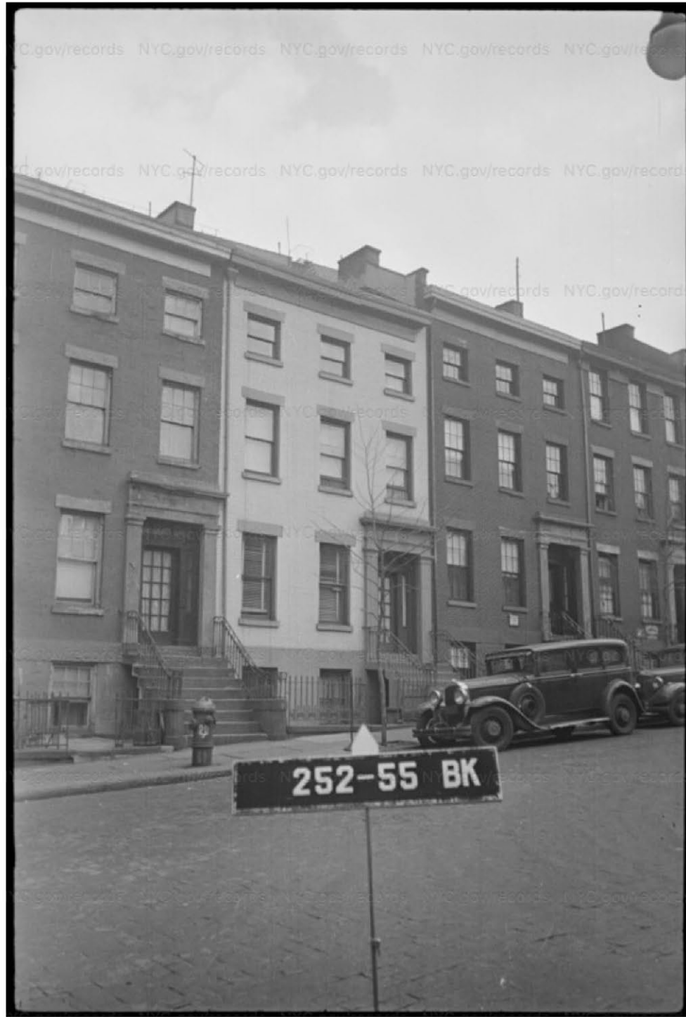
1940s TAX PHOTO 1-OVER-1 WINDOWS #39 SHOWS 6-OVER-1 #43 SHOWS 6-OVER-6
