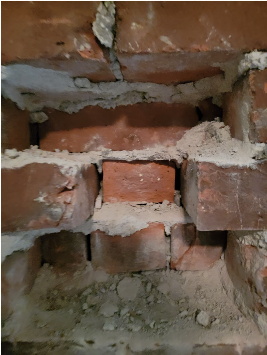
REAR WALL PROBE, 2ND FLOOR, INTERIOR
