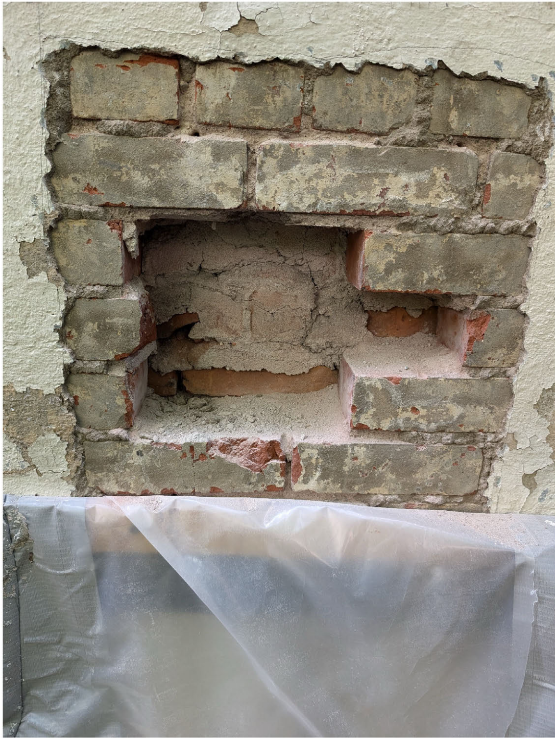
REAR FACADE PROBE, PARLOR LEVEL, EXTERIOR
