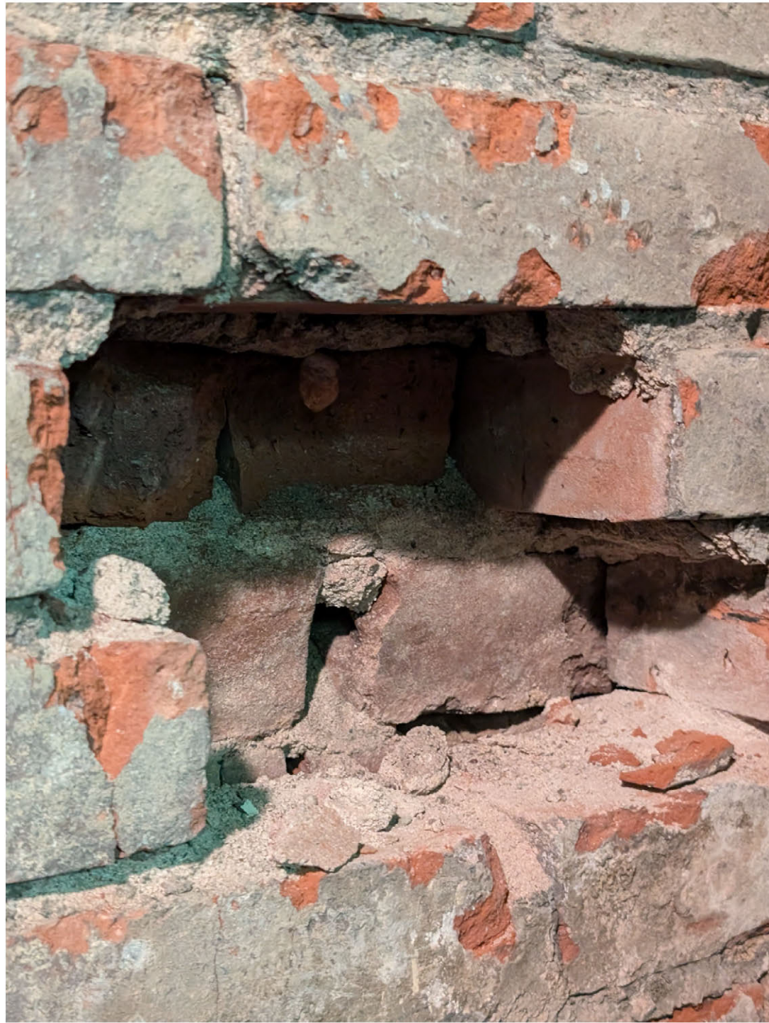
REAR FACADE PROBE, BASEMENT LEVEL, EXTERIOR
