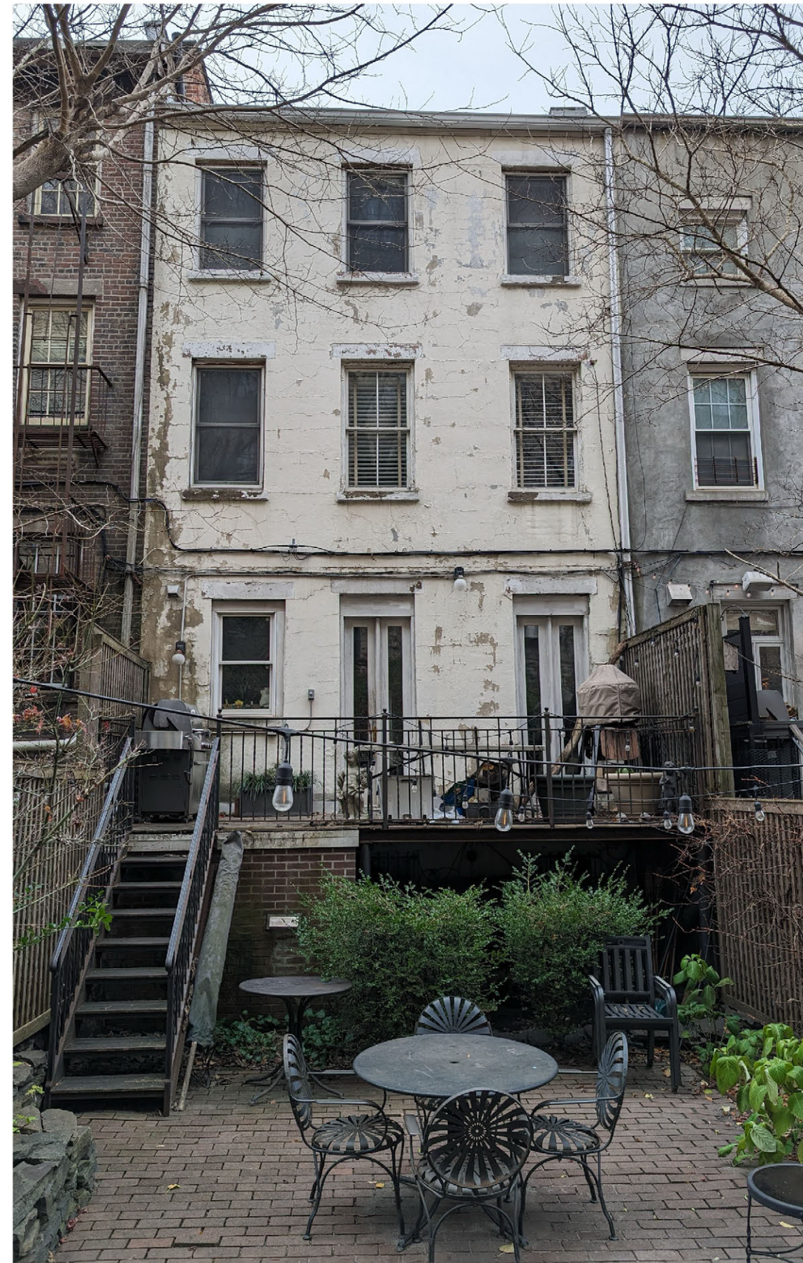
PHOTO OF EXISTING REAR FACADE
