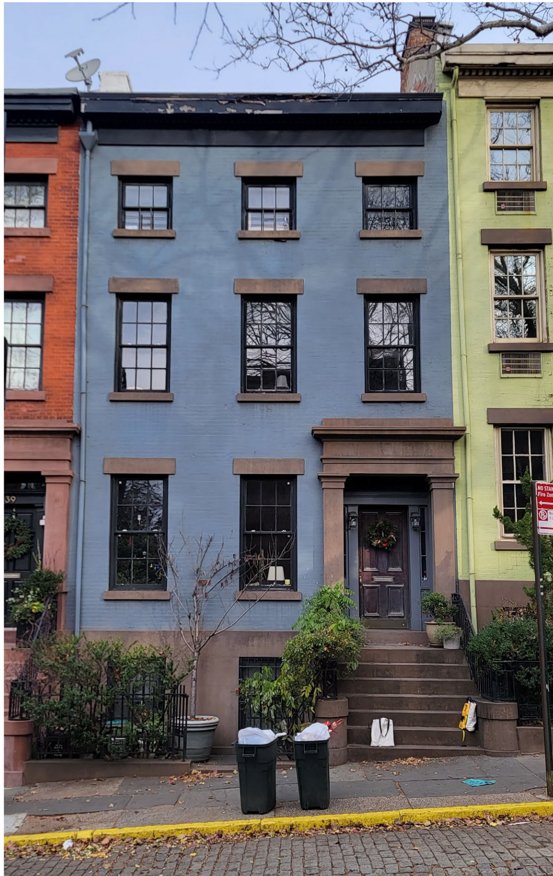
PHOTO OF EXISTING FRONT FACADE
