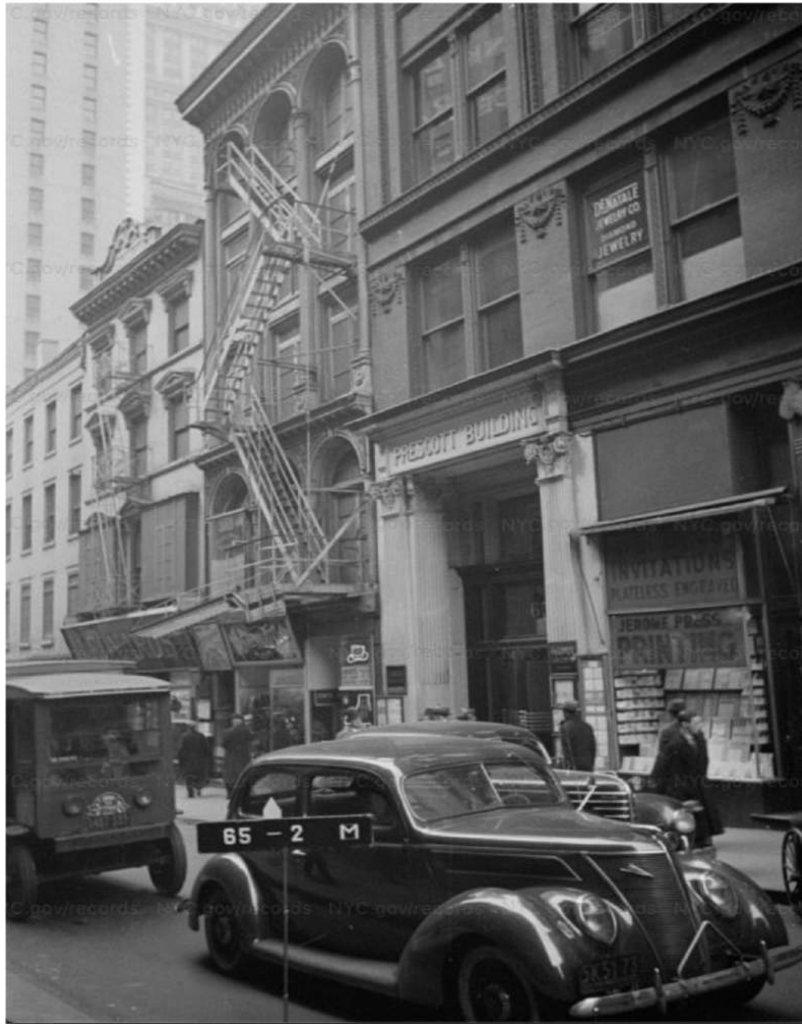
Built c. 1844; cast-iron facade c.1857-59, attributed to James Bogardus
