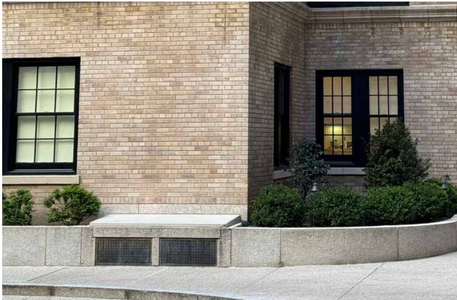
Existing Light Well
