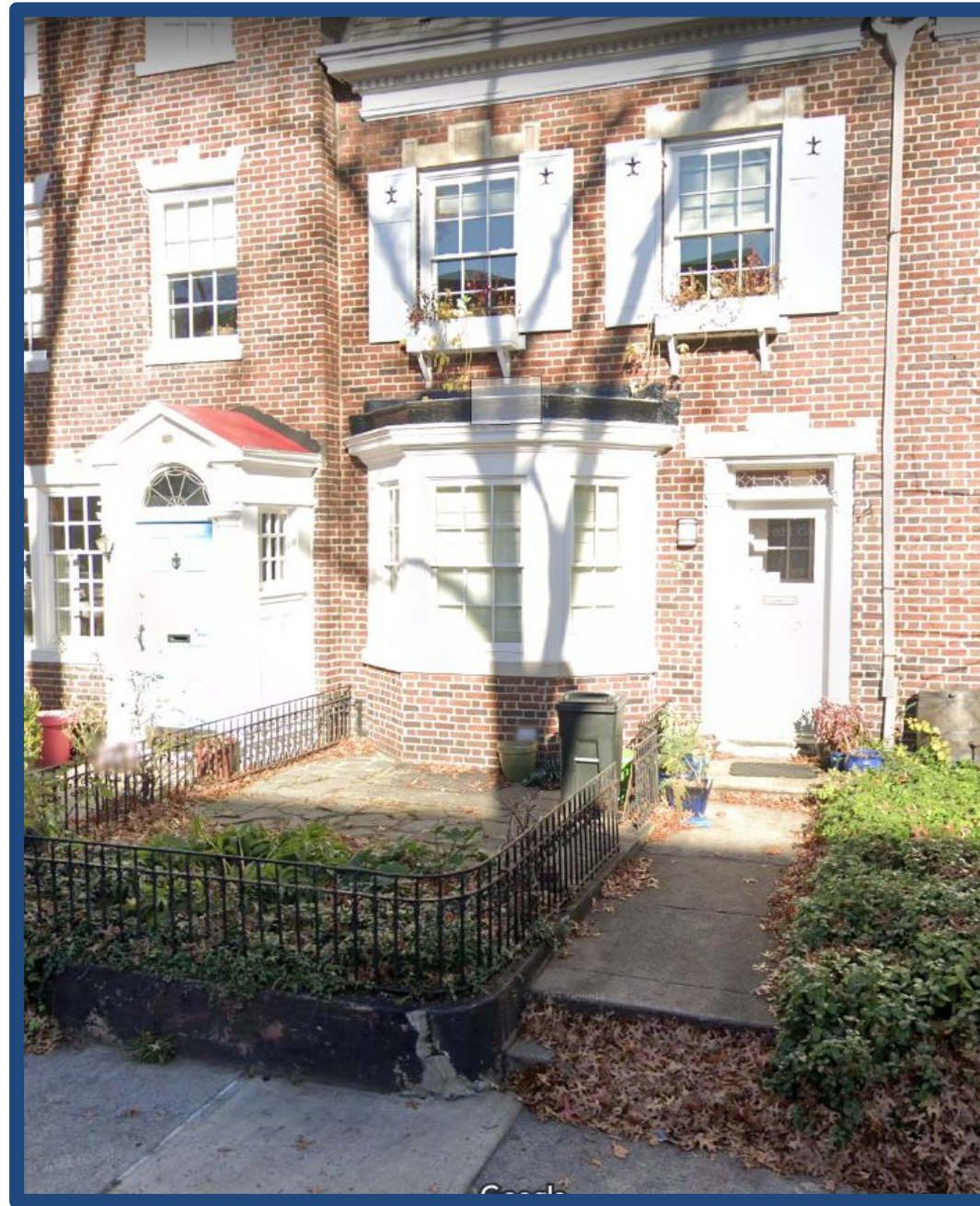
2119 Albemarle Terrace Wall Height above Sidewalk: 23" Wall Height above Walkway: 7"
