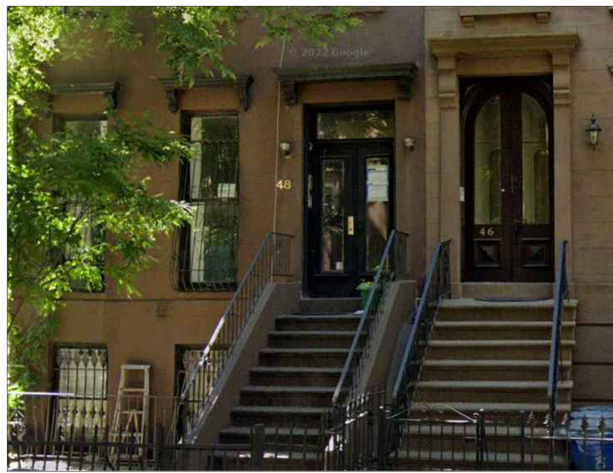
STOOPS AND FRONT DOORS - 48 AND 46 CLIFTON PLACE
