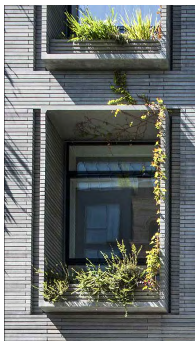
WINDOW DETAILING 41 BOND STREET NOHO HISTORIC DISTRICT EXTENSION
