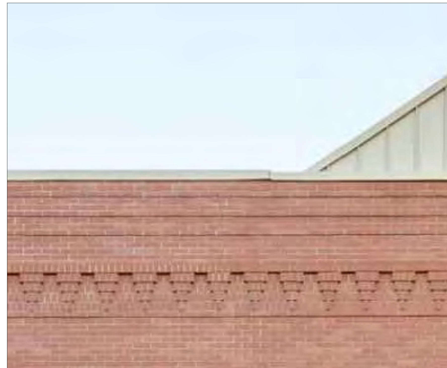
MODERN BRICK STACKED PARAPET, BUILT 2015 259 - 261 BERRY STREET
