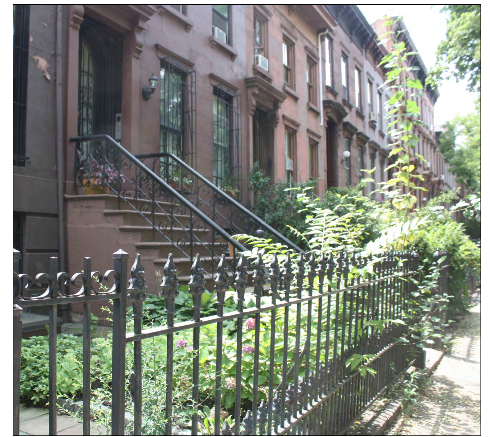
STOOPS AND FRONT DOORS -44 CLIFTON PLACE
