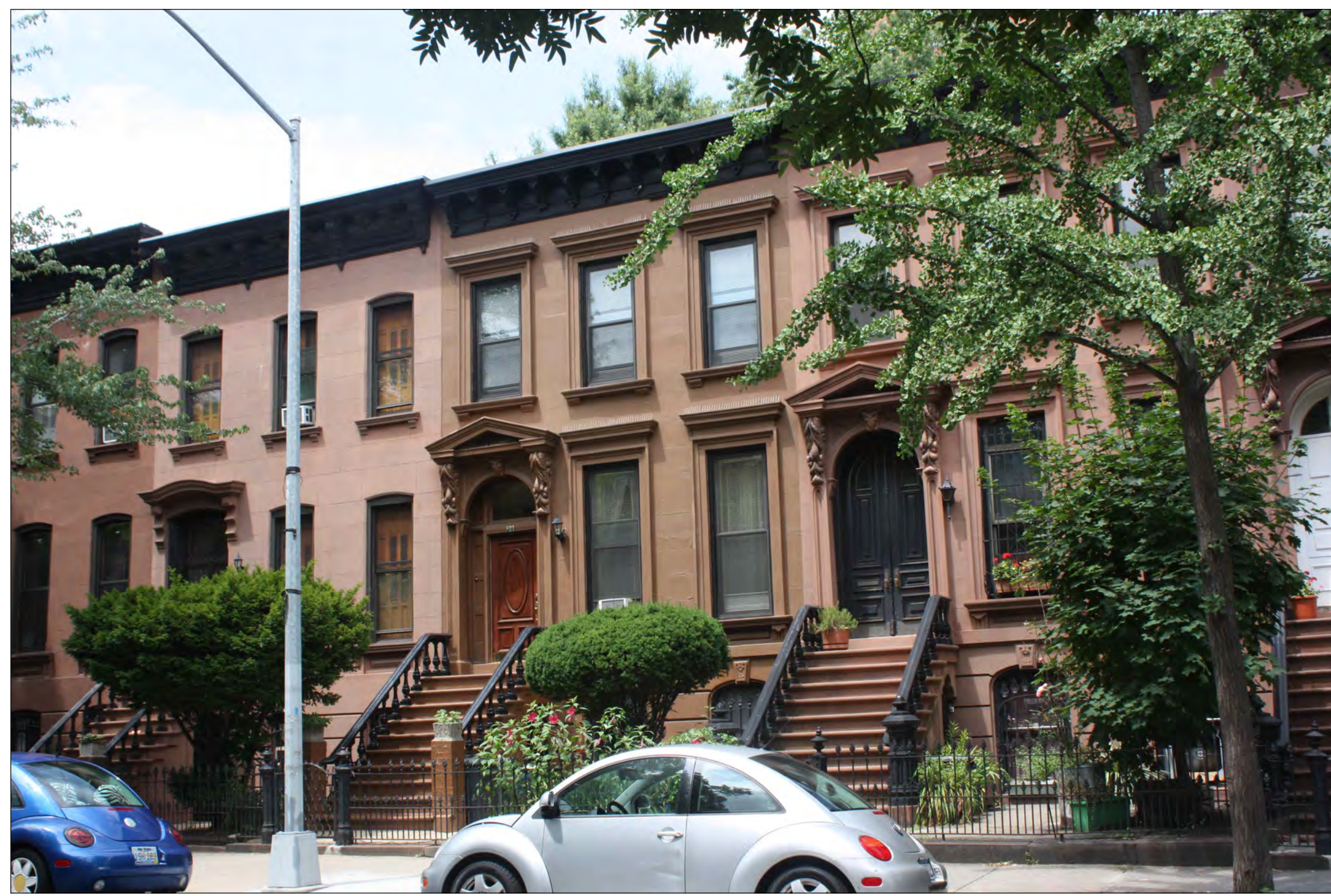
PARAPETS - 29 - 33 CLIFTON PLACE
