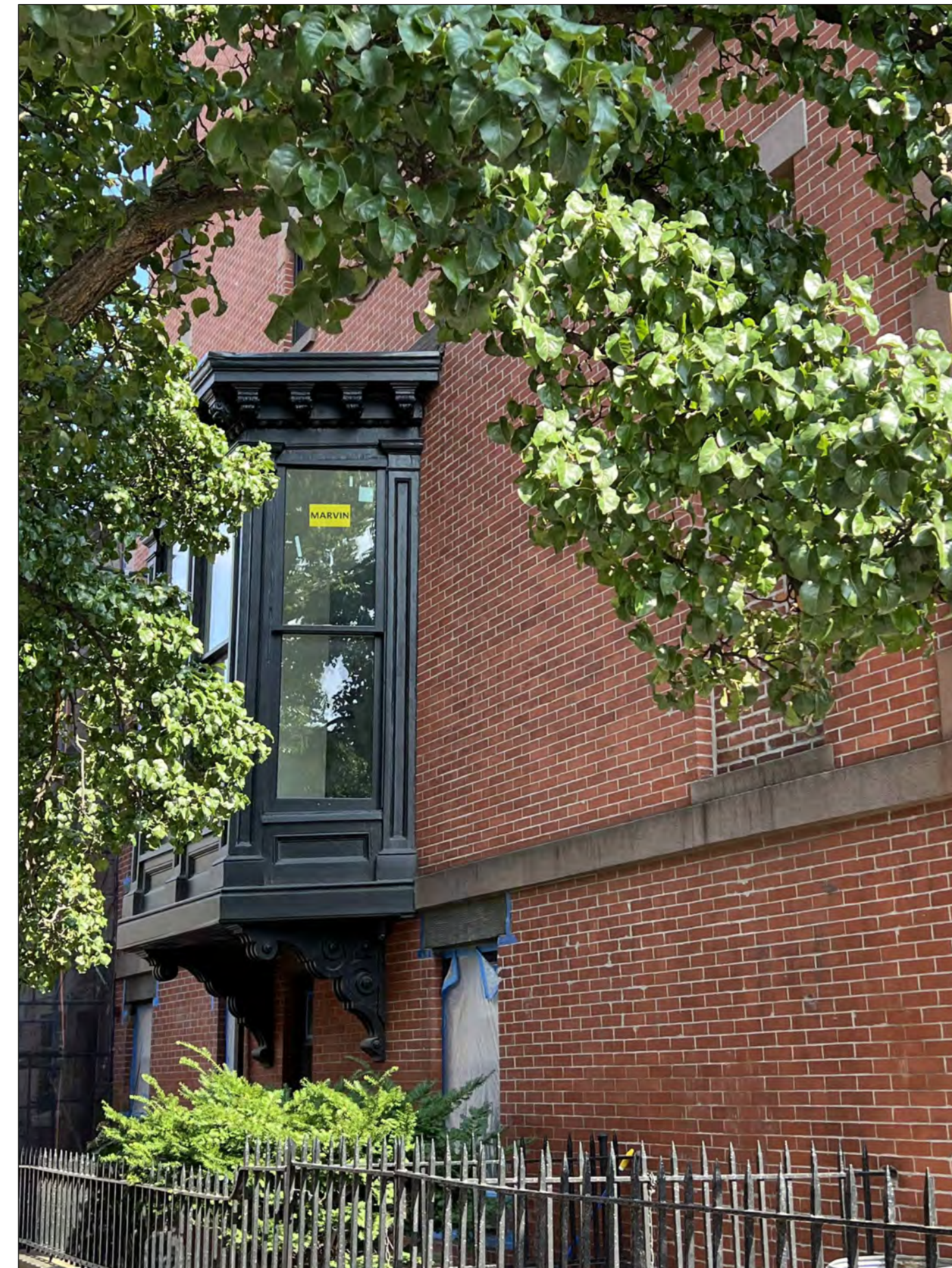
BAY WINDOW - 1 CAMBRIDGE PLACE (NARROW STREET)
