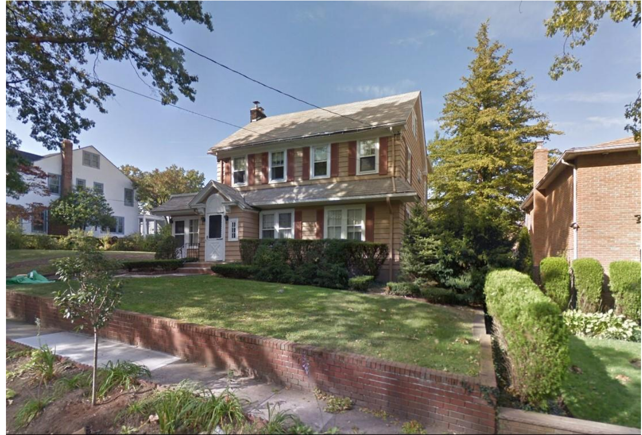
Retaining Wall Prior to Removal and Replacement
