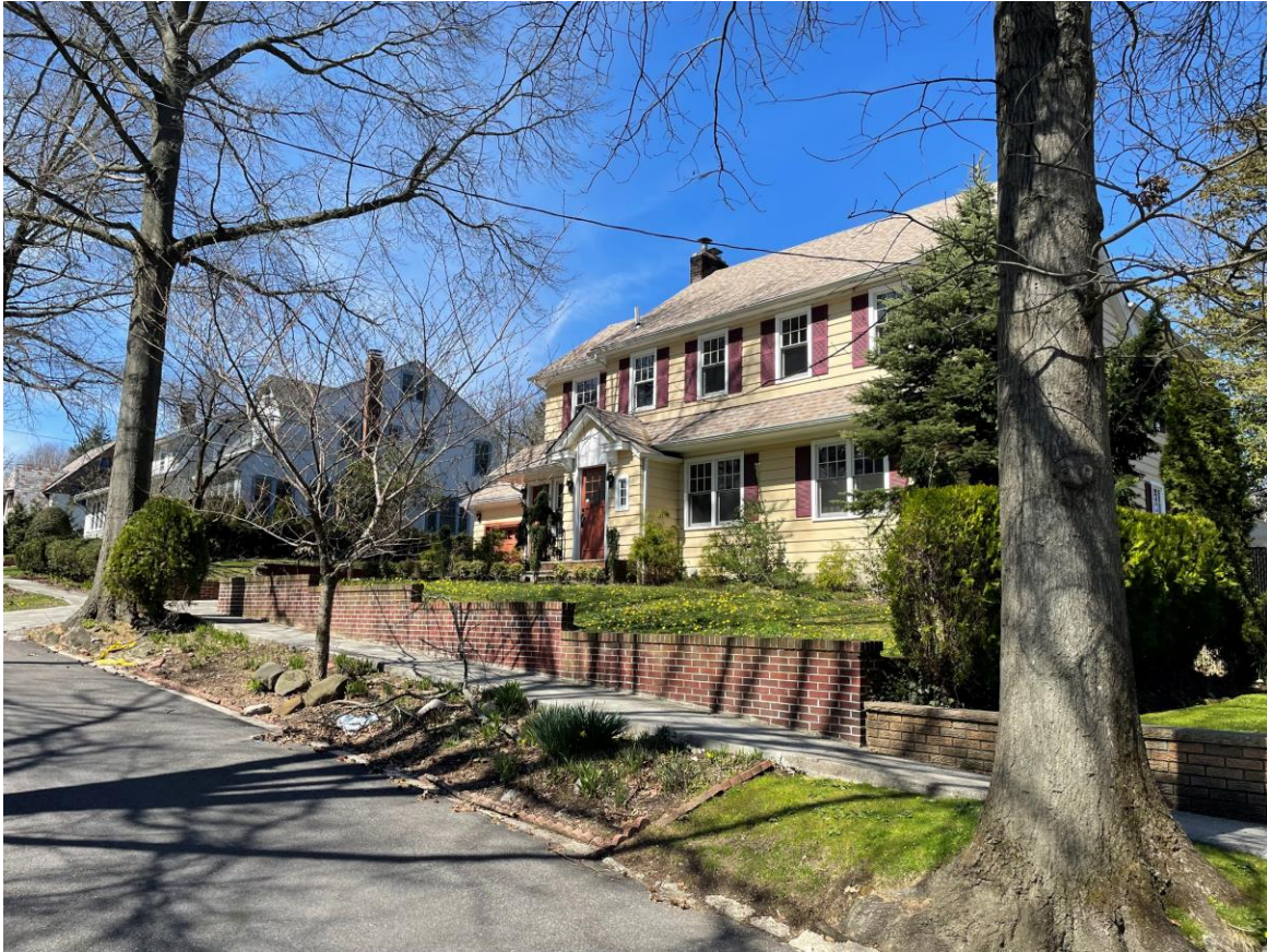
New Stepped Retaining Wall
