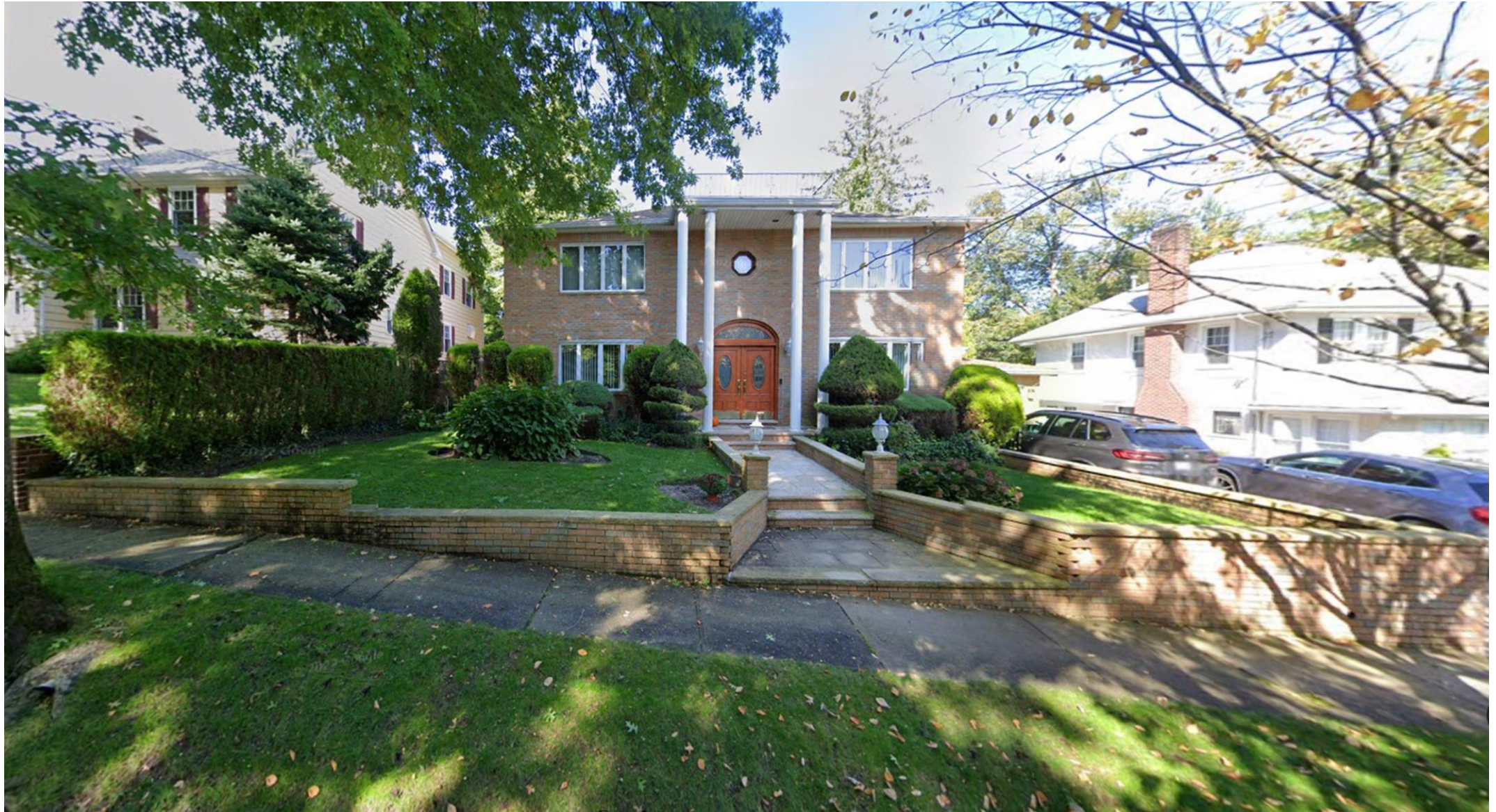
357 Hollywood Avenue – Stepped Retaining Wall
