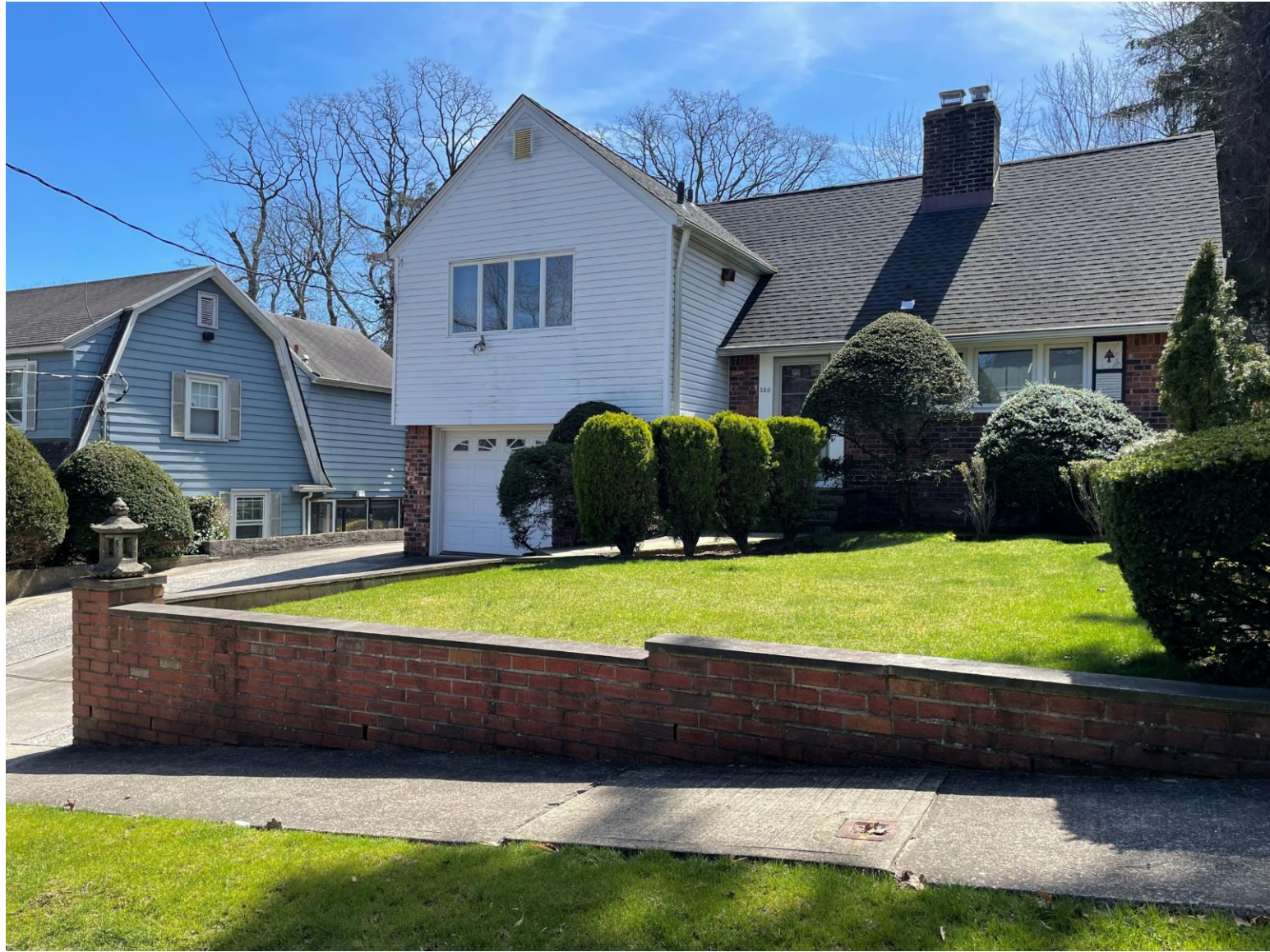
350 Arleigh Road – Stepped Retaining Wall
