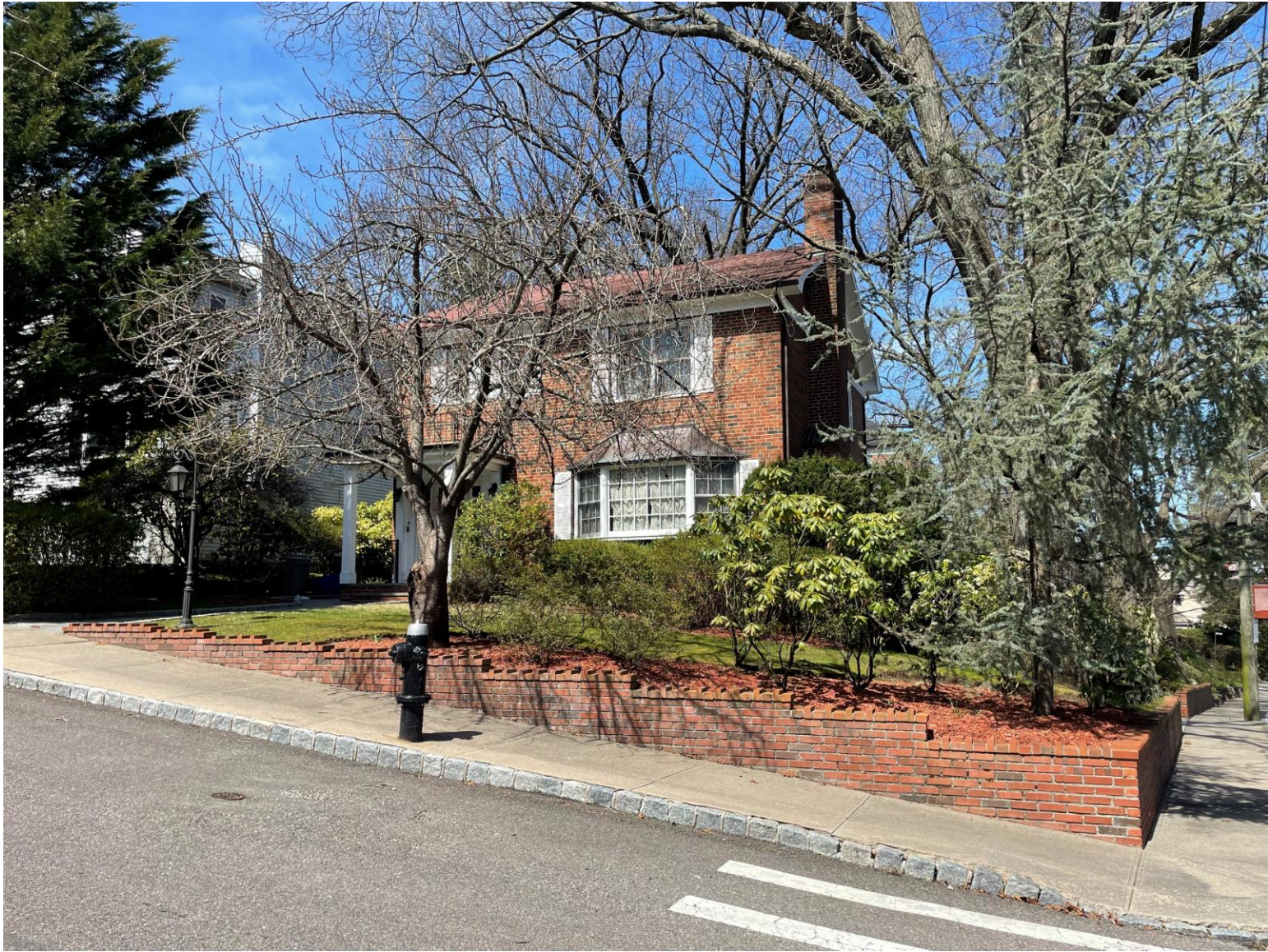
23 Oak Lane – Stepped Retaining Wall
