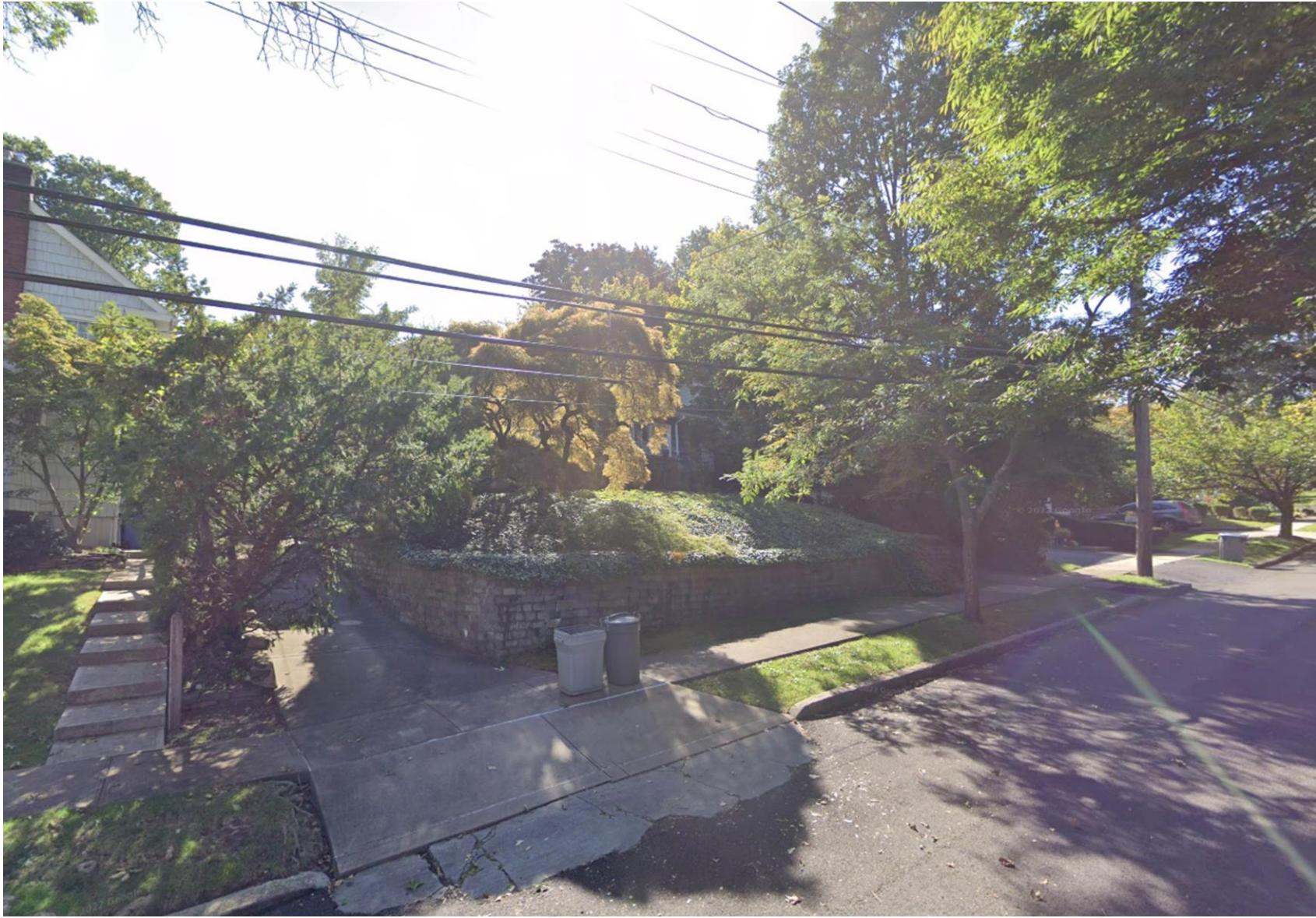
322 Hollywood Avenue – Retaining Wall
