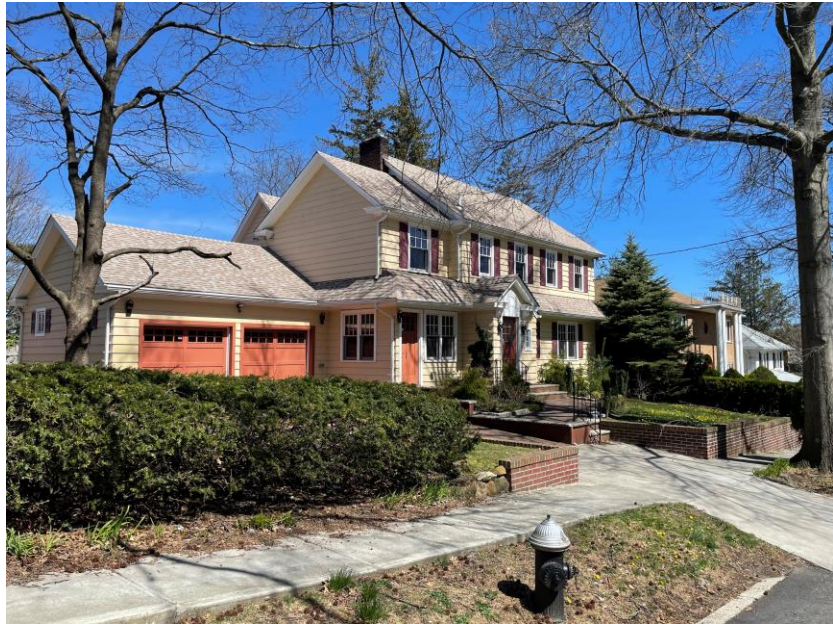
b. Front yard stepped retaining wall – no permit issued
