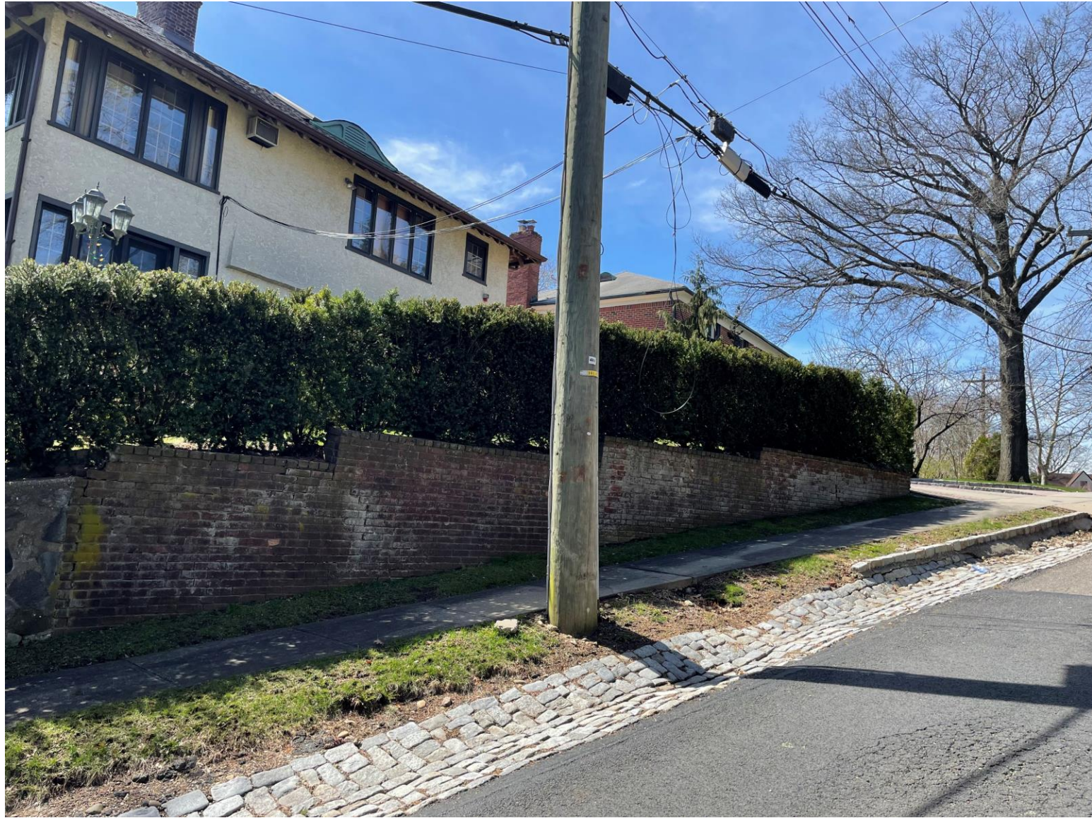
4 Oak Lane – Stepped Retaining Wall
