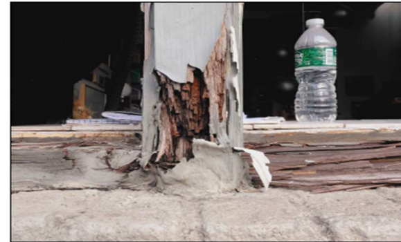
DETERIORATING MULLION REMOVED
