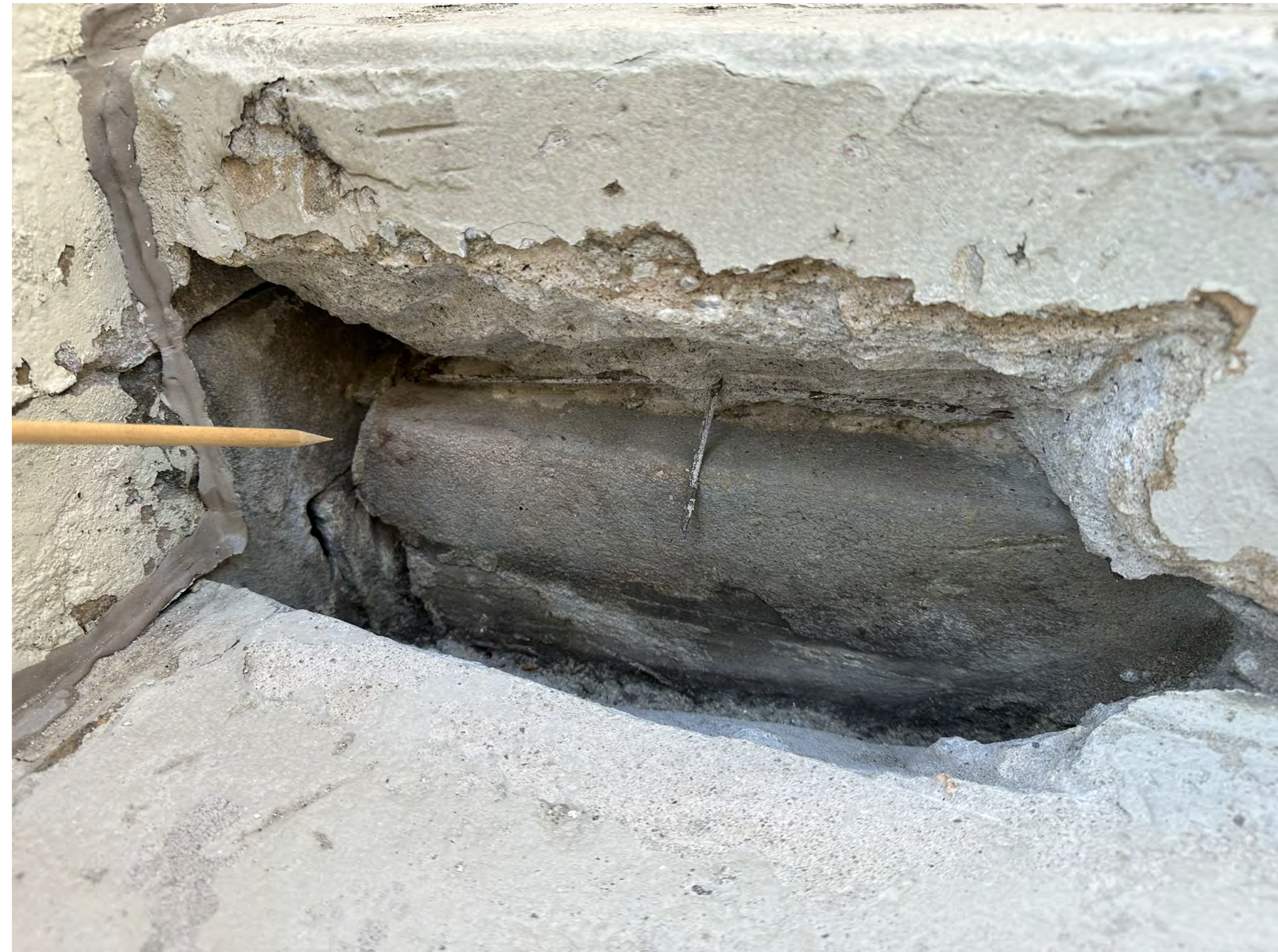
1 EXISTING STEP CONDITION - EXTERIOR SCALE: NTS
