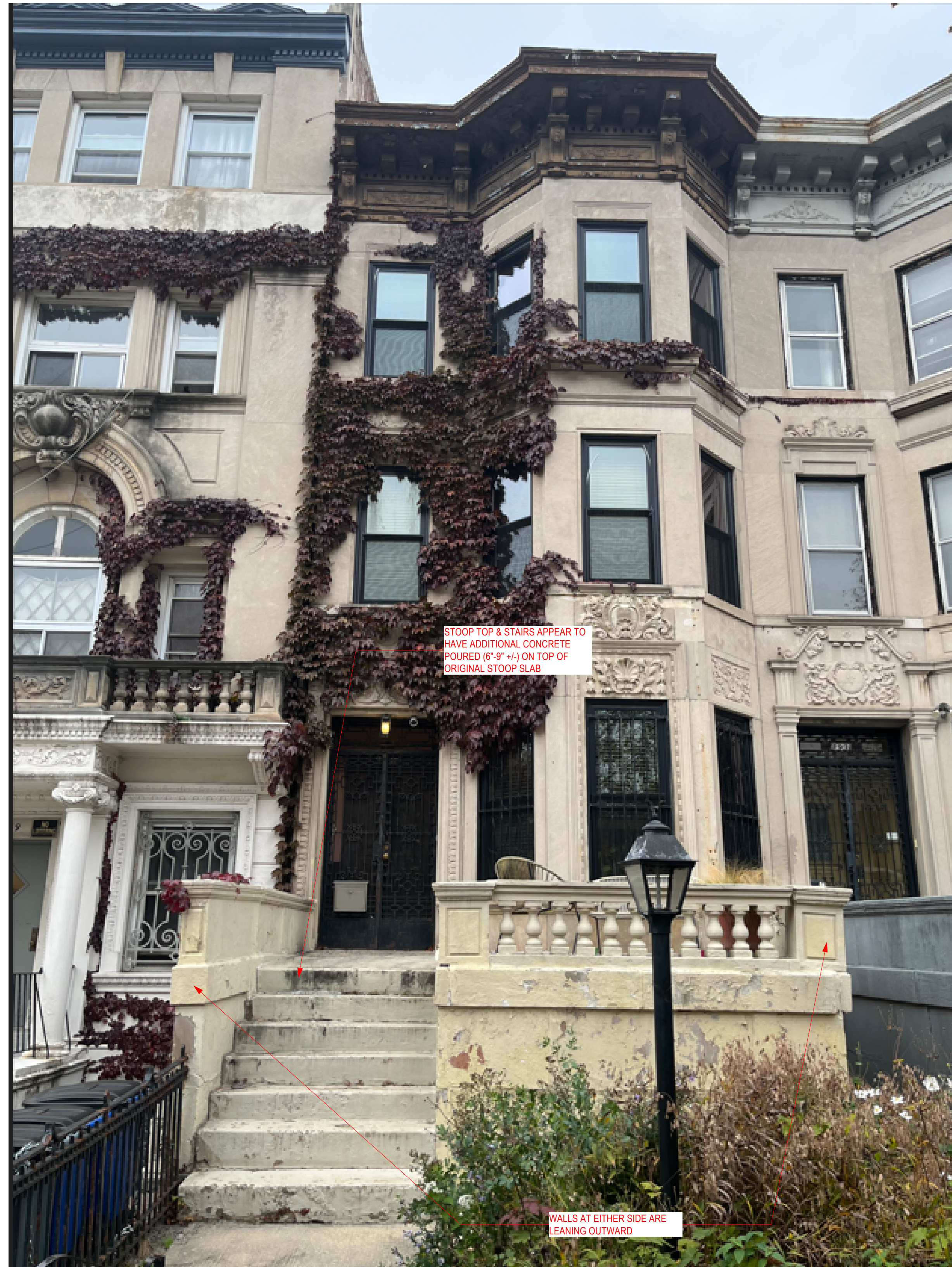
2 CURRENT CONDITION @ FRONT FACADE SCALE: NTS
