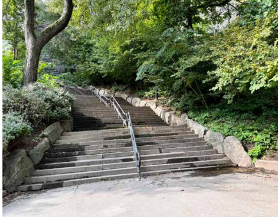
B. Boulder walls early 1900's
