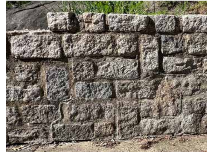
Existing granite block- to be re-used
