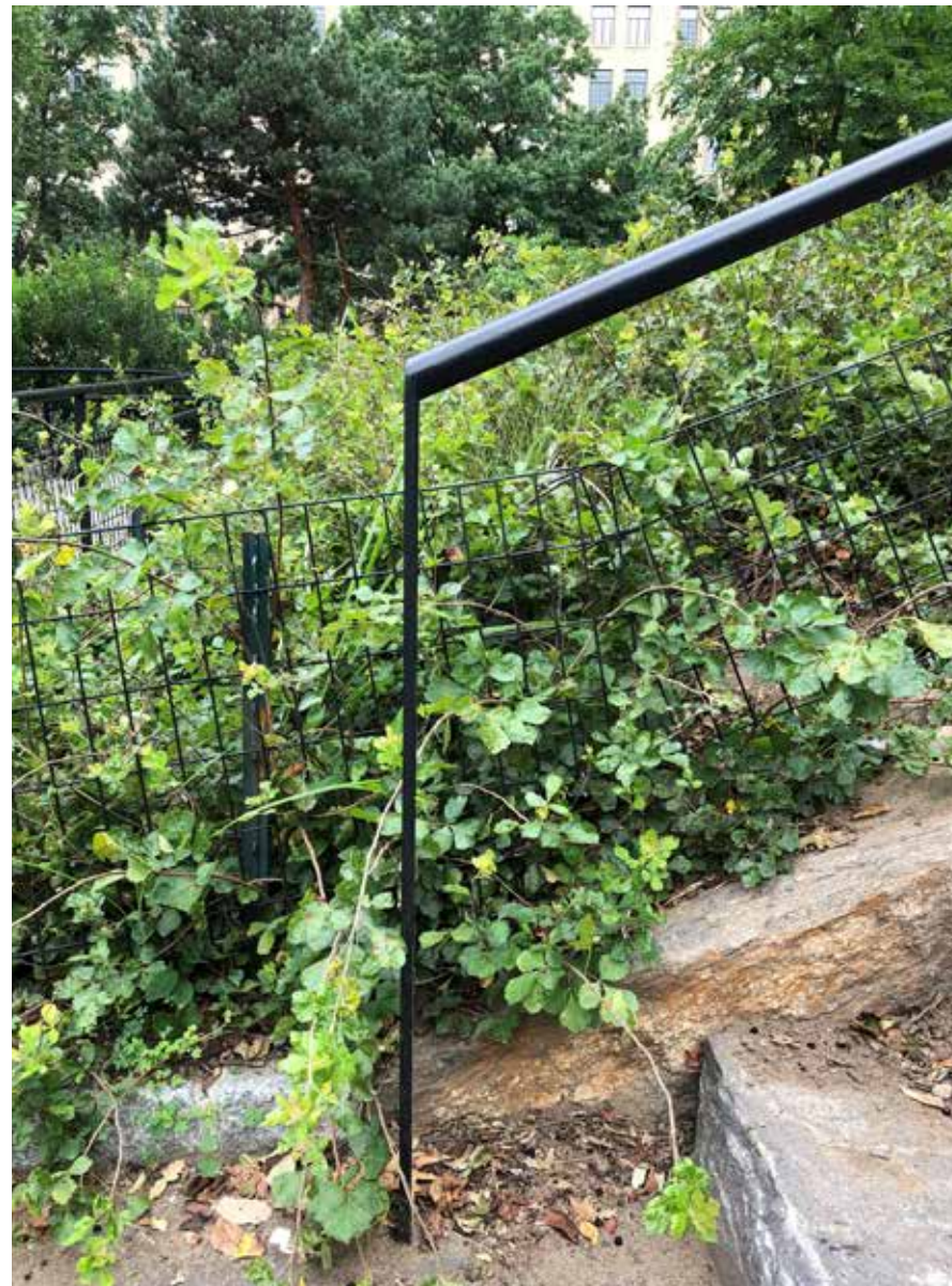
Handrail previously approved by LPC for Morningside Park
