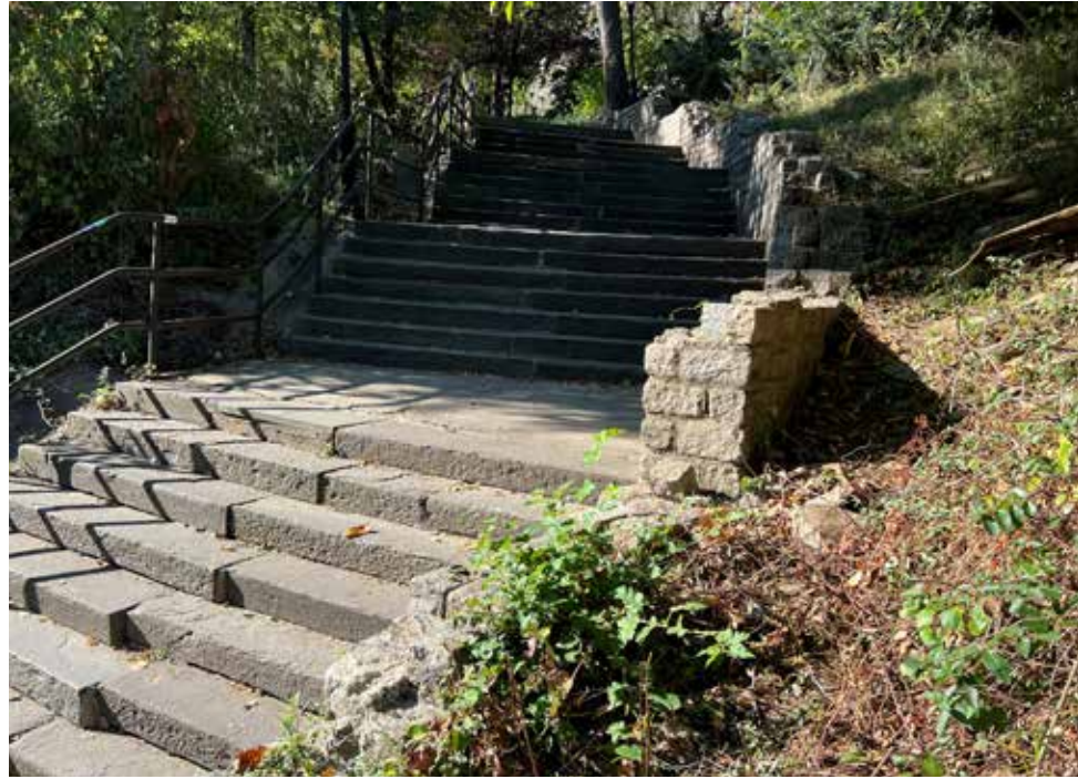
D. 1940's-1960's Granite block cheekwall at 122nd St. to be reconstructed
