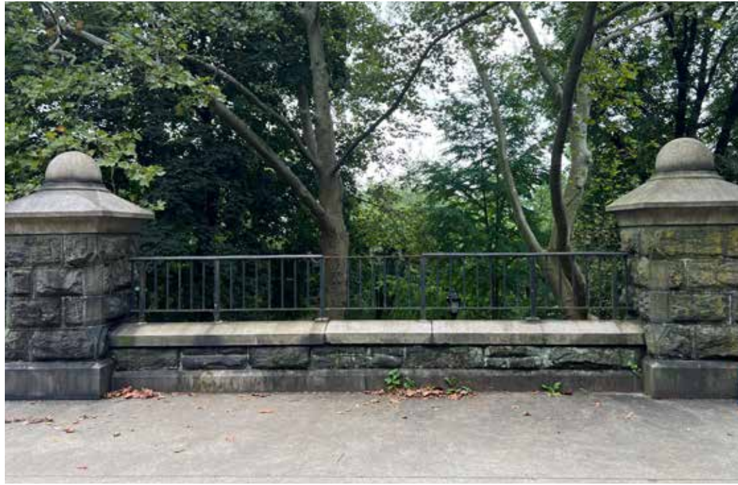
A. Perimeter wall 1890's
