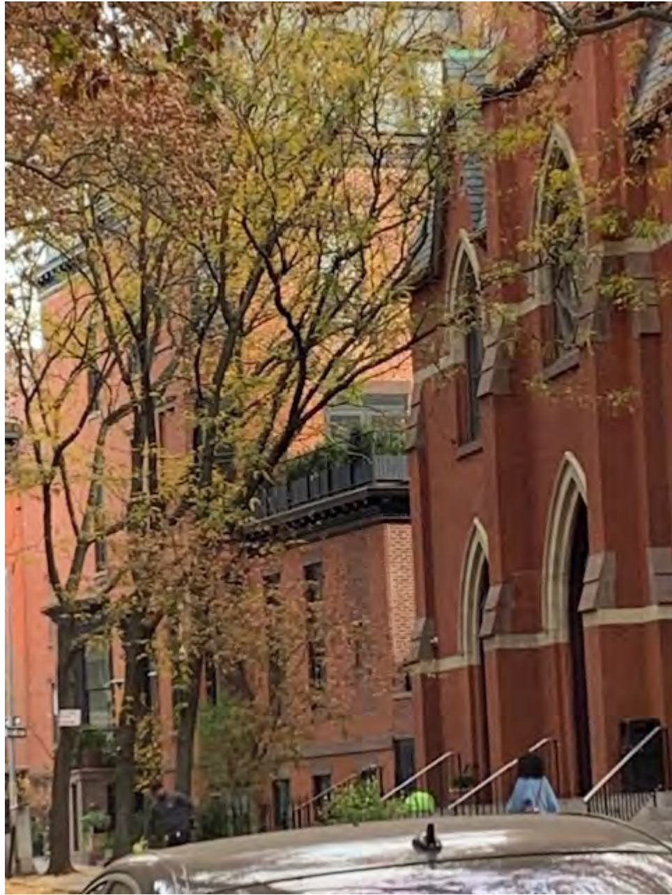
EXISTING TERRACE STREET VIEW
