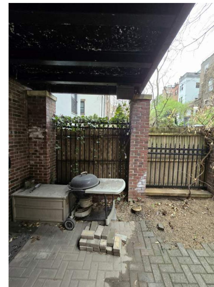
garden level under deck looking east.
