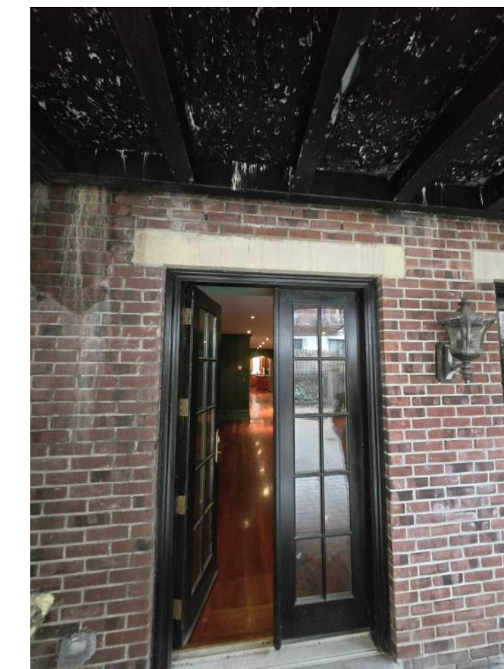
garden door typical - being removed
