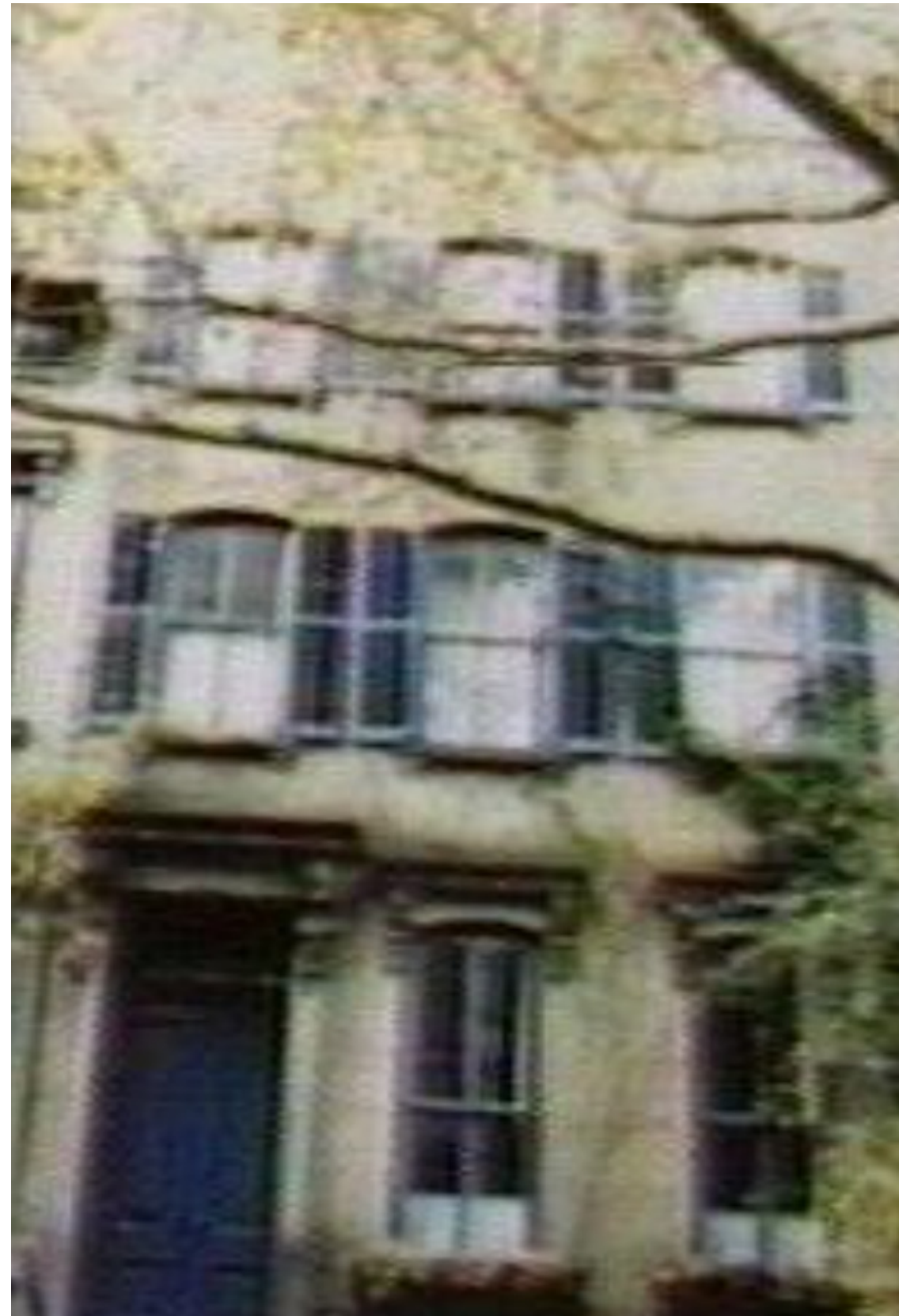
FRONT FACADE Year taken: 1980s - Tax Photo
