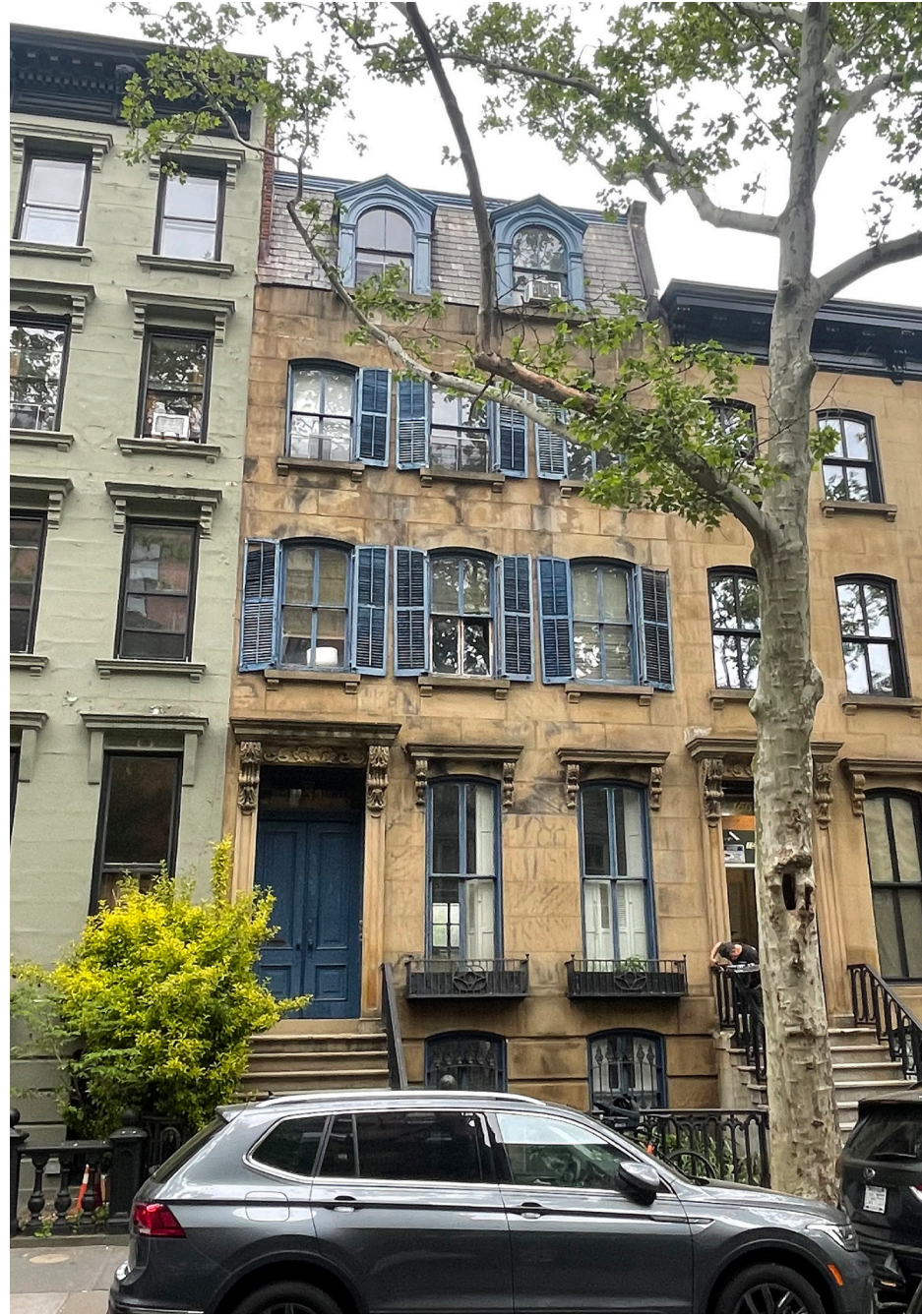
VIEW 2: FRONT VIEW - NOT VISIBLE
