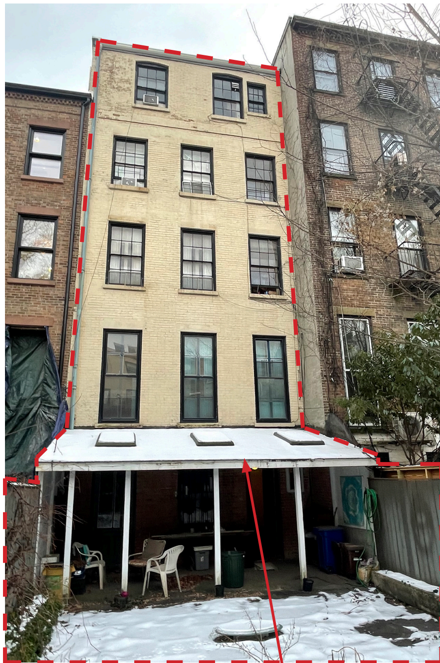
Site Photo: Exterior rear facade view
