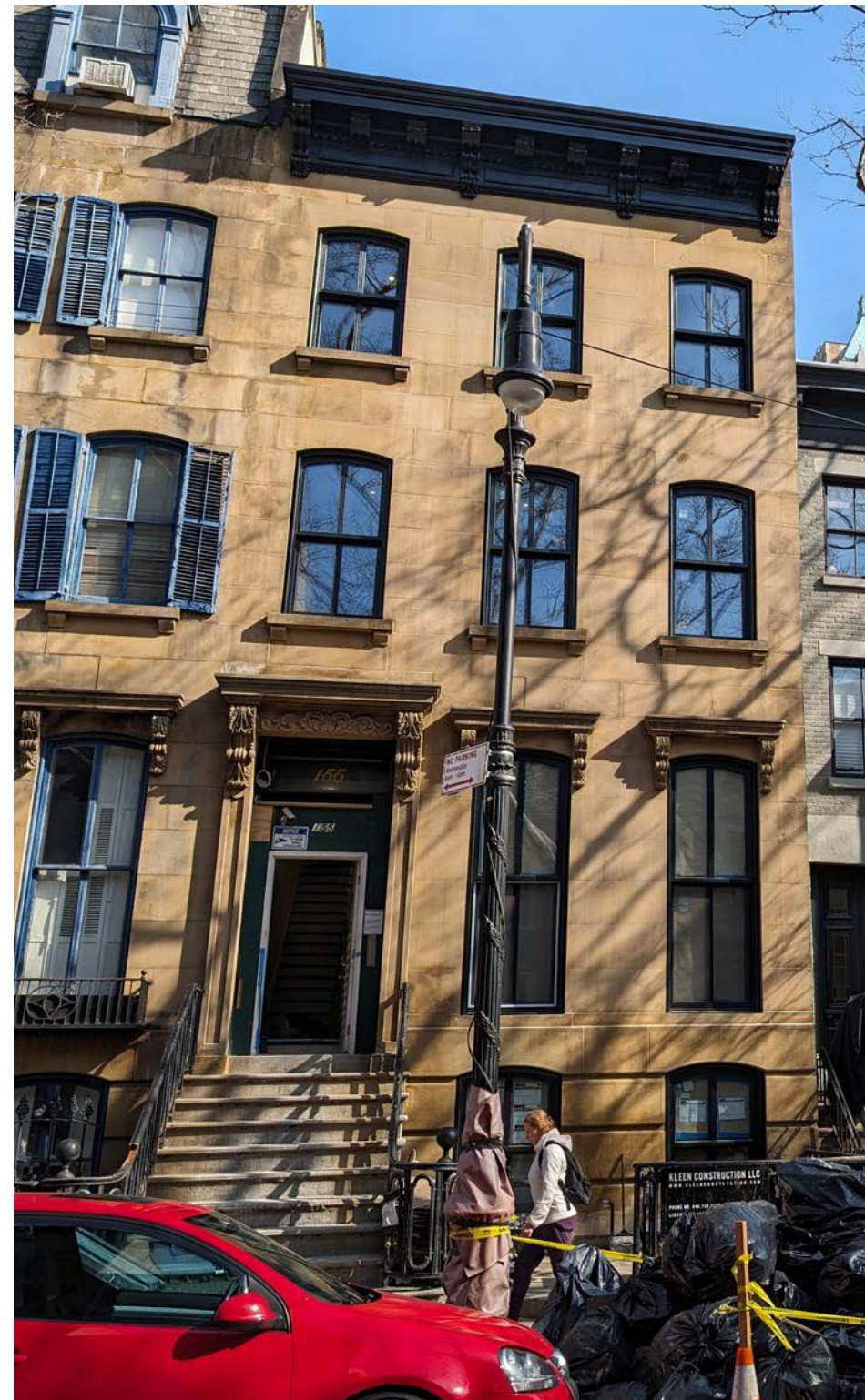
ADJACENT PROPERTY: 155 STATE STREET
