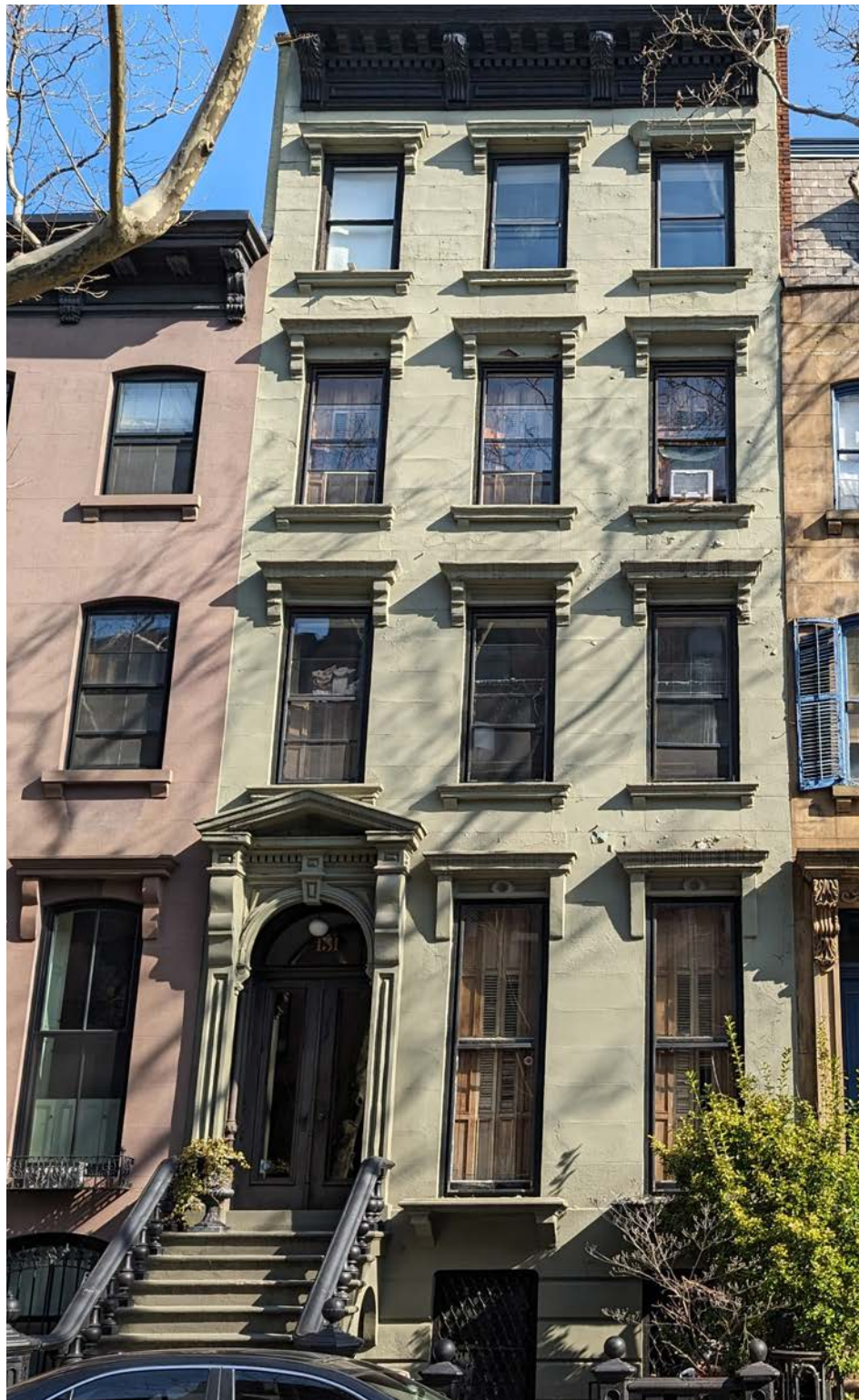
ADJACENT PROPERTY: 151 STATE STREET
