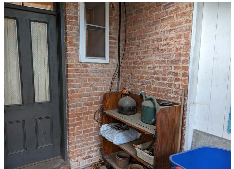
Site Photo: Rear door and window with brick wall
