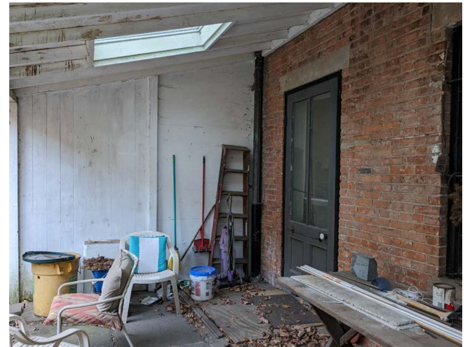
Site Photo: Rear patio showing existing patio and floor hatch location
