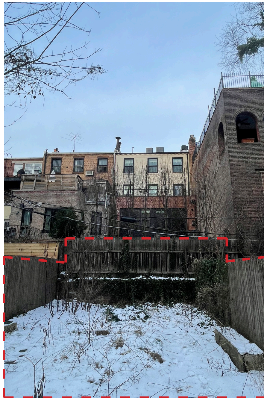
Site Photo: Rear yard
