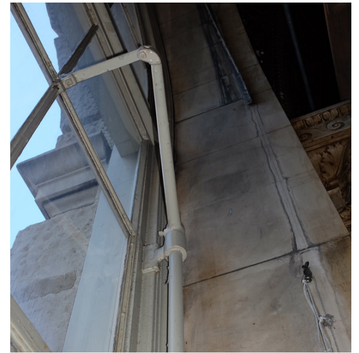
Arm attachments to windows and shaft
