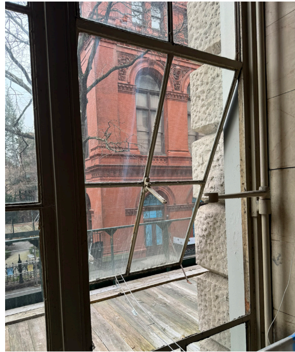
Awning window from interior.
