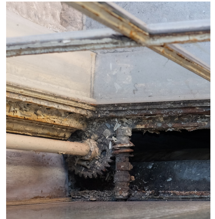
Worm gear and shaft to turn arms (crank is missing)
