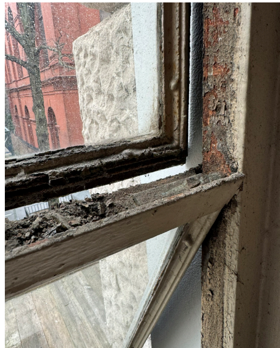
Awning window from interior.
