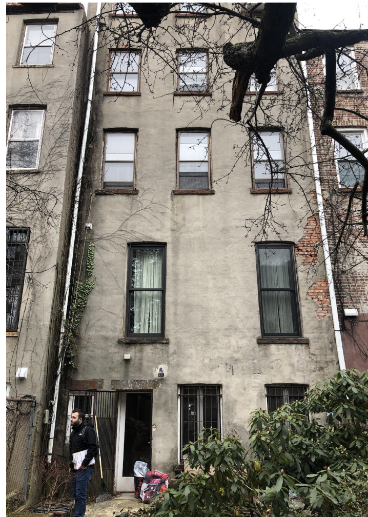
EXISTING CONDITIONS REAR FACADE
