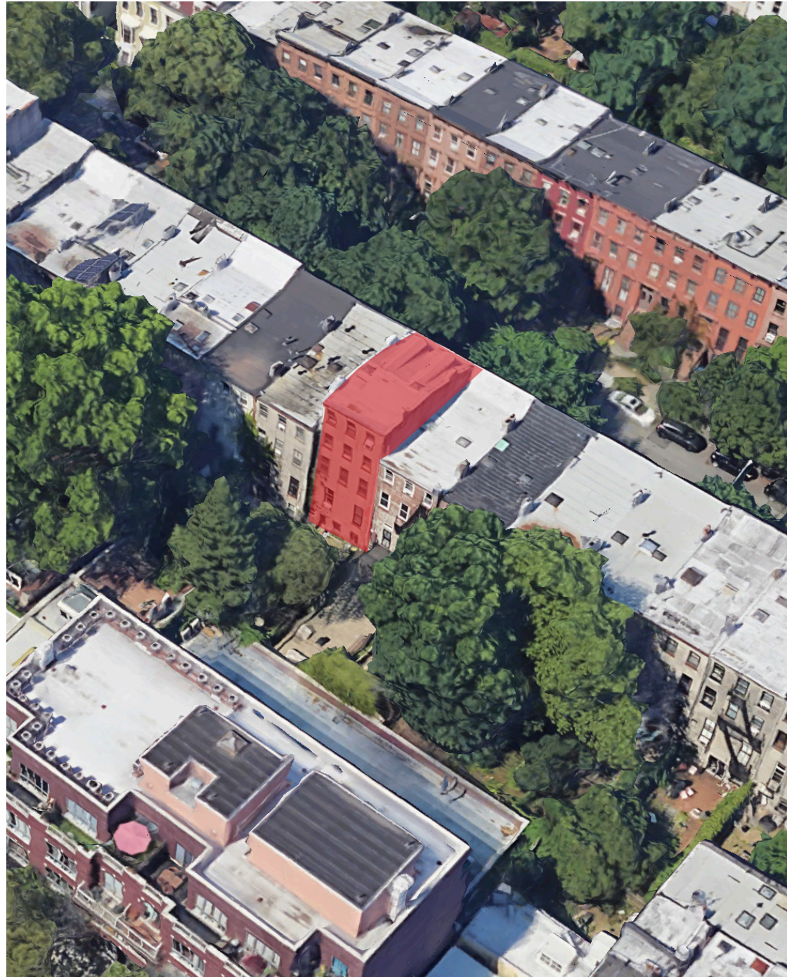
AERIAL VIEW OF REAR FACADE
