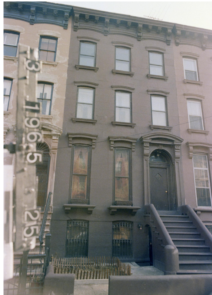
TAX PHOTOS FRONT FACADE
